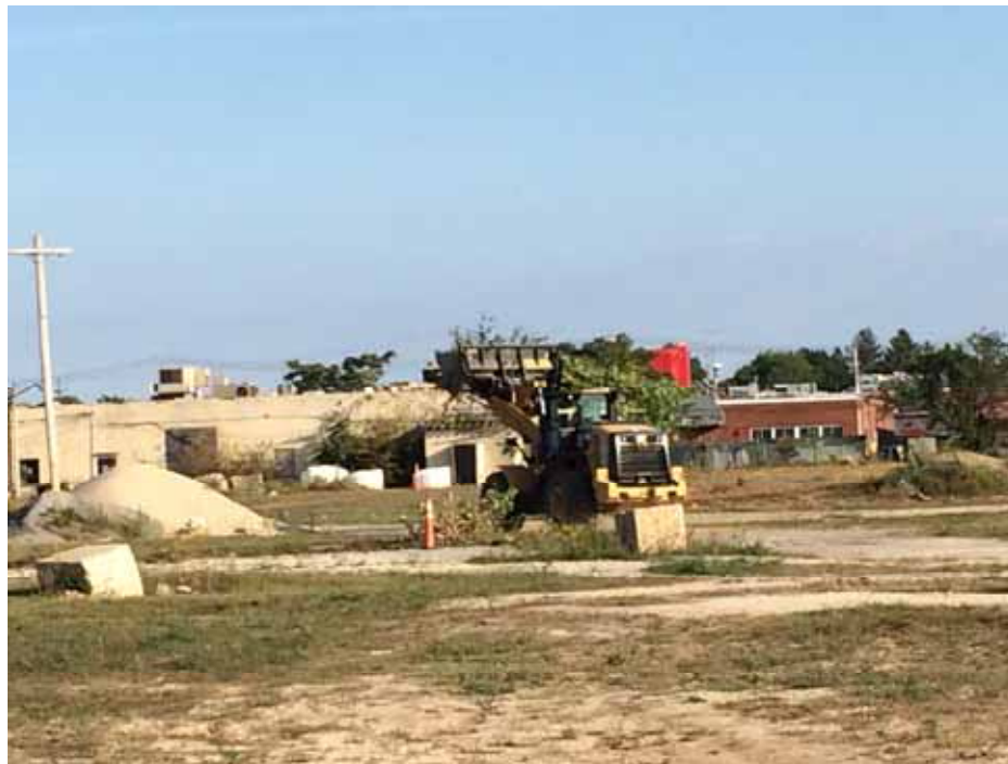
Posillico transporting cleared trees (less than 8-inch in diameter) and large brush across site during site clearing activities.
