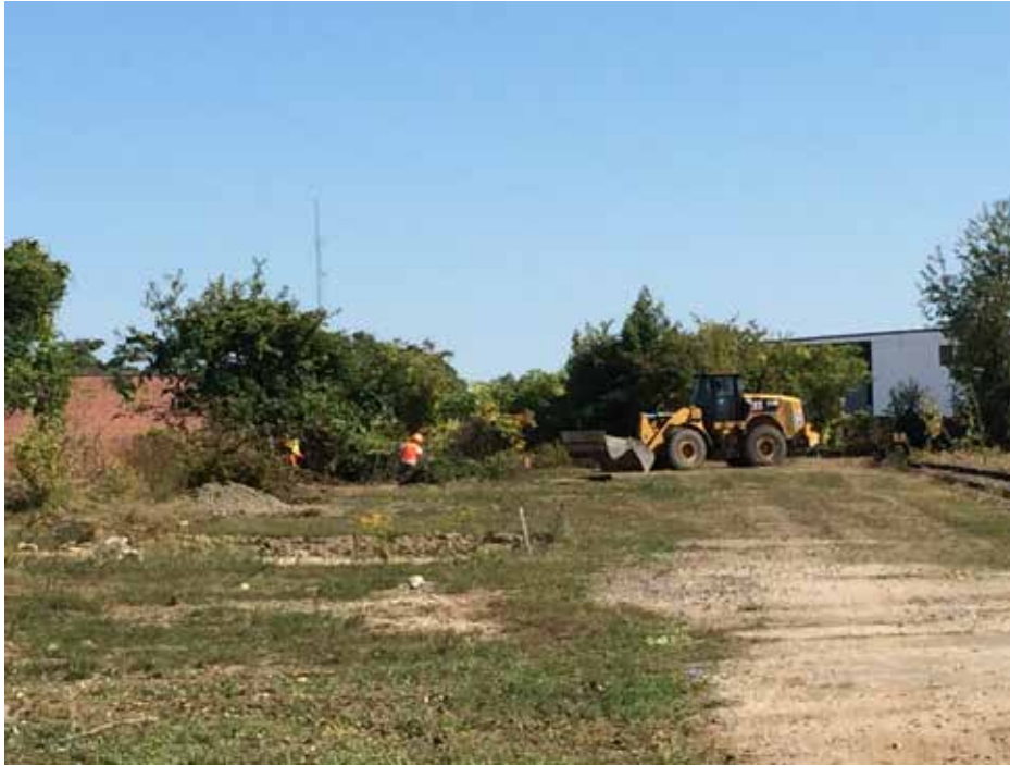
Posillico conducting site clearing activities with Caterpillar 950K Loader with Brush-Hog attachment.
