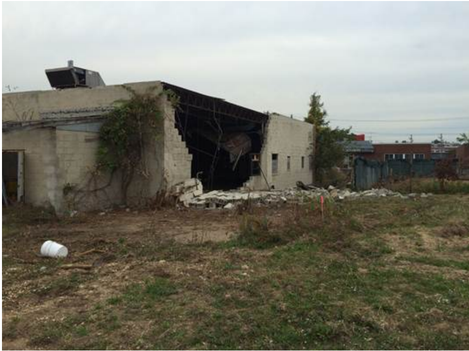
East side of Administration Building after cinderblock wall collapsed outward.
