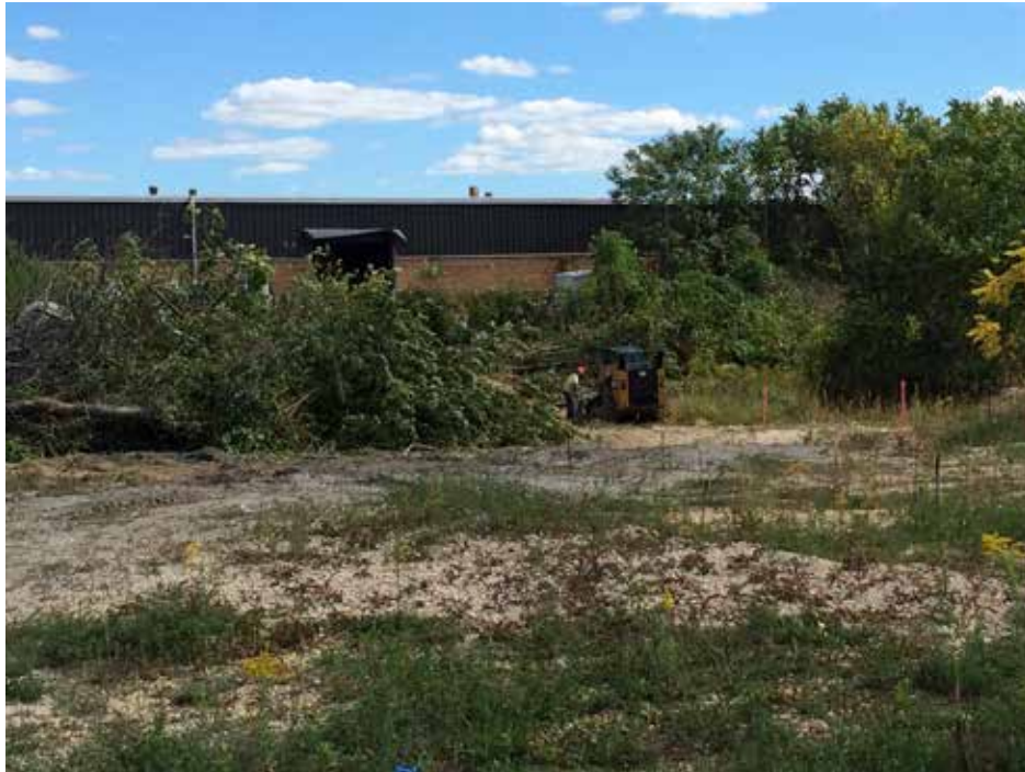
Posillico conducting site clearing activities with the Caterpillar 299D Compact Track Loader.
