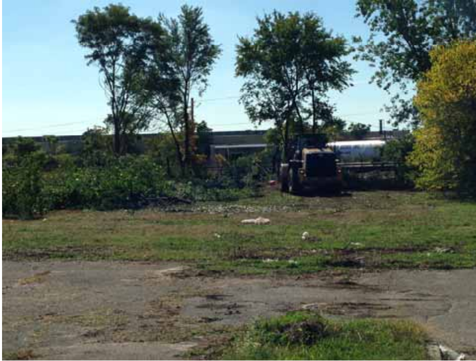
Posillico performing site clearing activities with the Caterpillar 950K loader.
