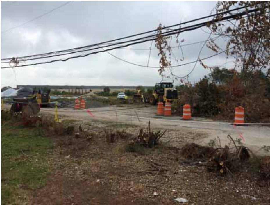
Posillico performing wood chipping with the Vermeer BC1800 wood chipper.
