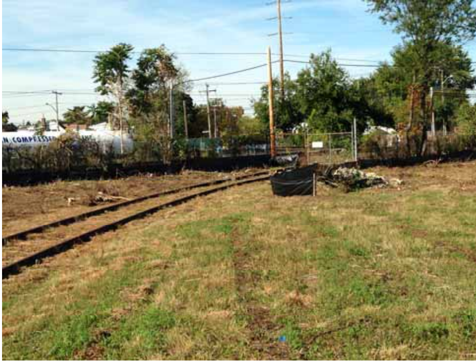
Photo of installed silt fence.
