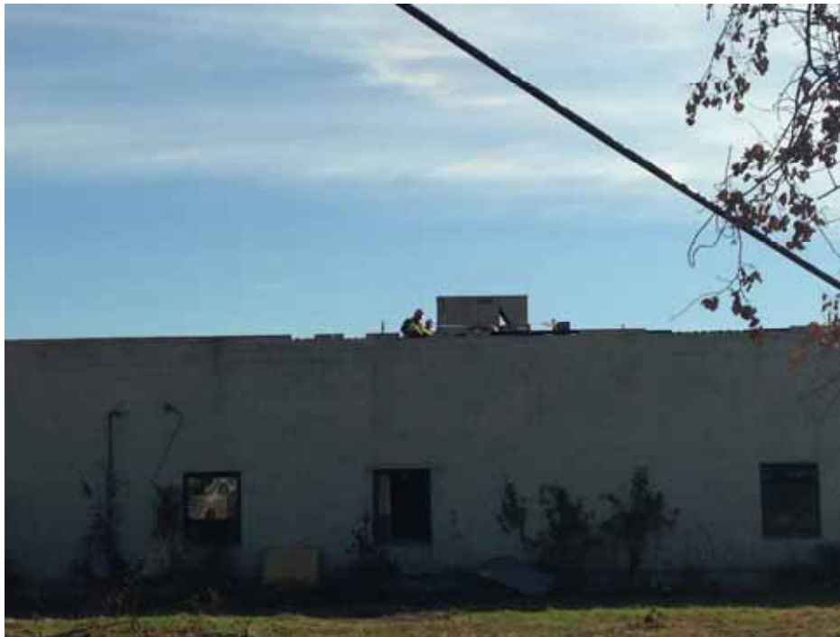
Posillico performing partial disassembly of west HVAC unit.
