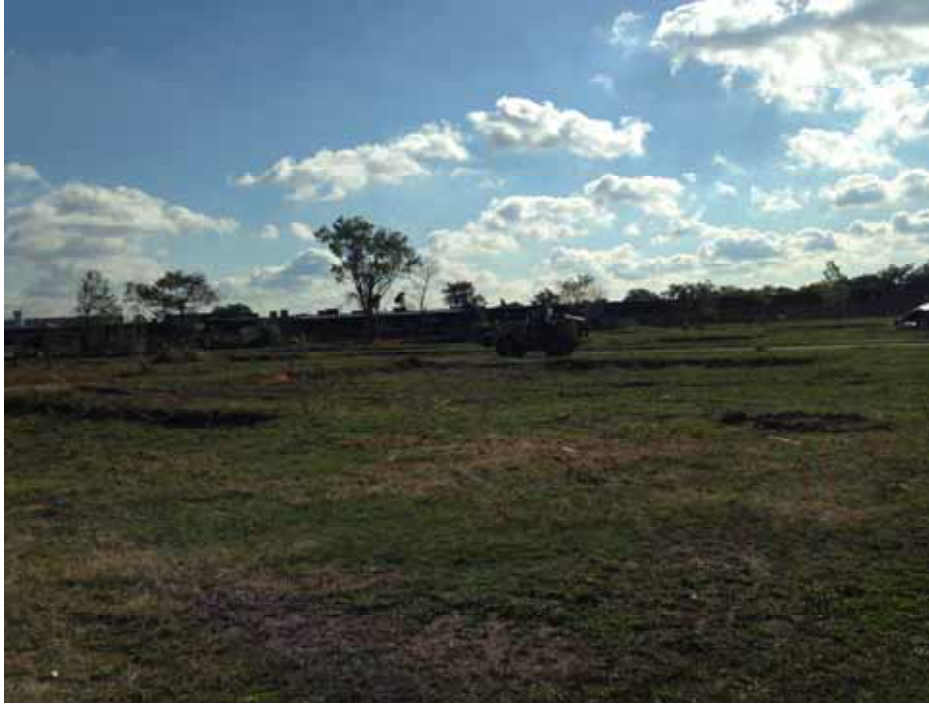
Posillico performing haul road construction with the Caterpillar 950K loader.
