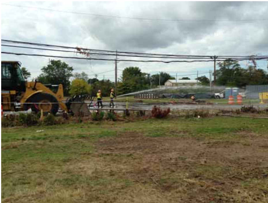
Posillico preformed dust suppression.
