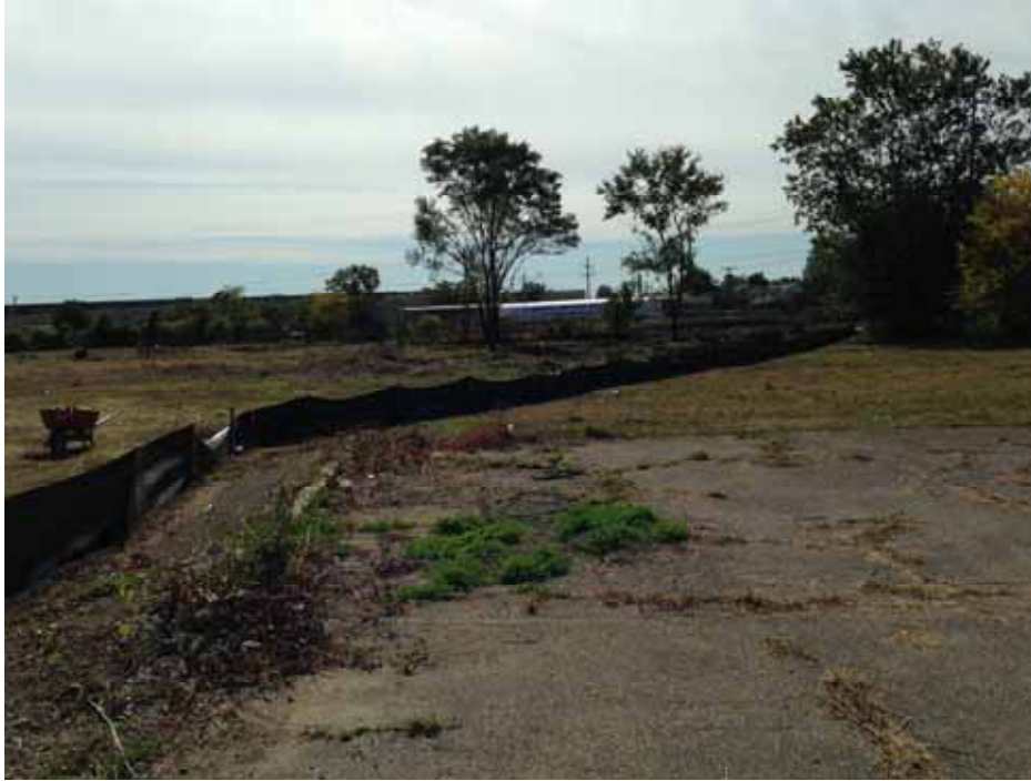
Photo of installed silt fence.
