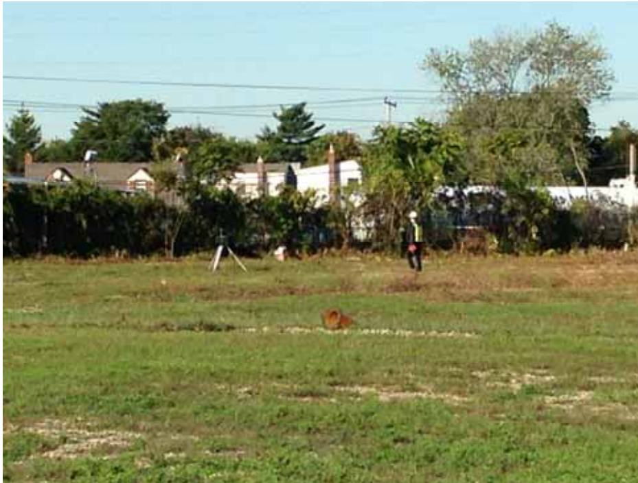
Posillico's air monitoring subcontractor, Preferred, performing CAMP implementation.
