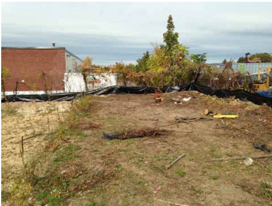
Photo of installed silt fence.
