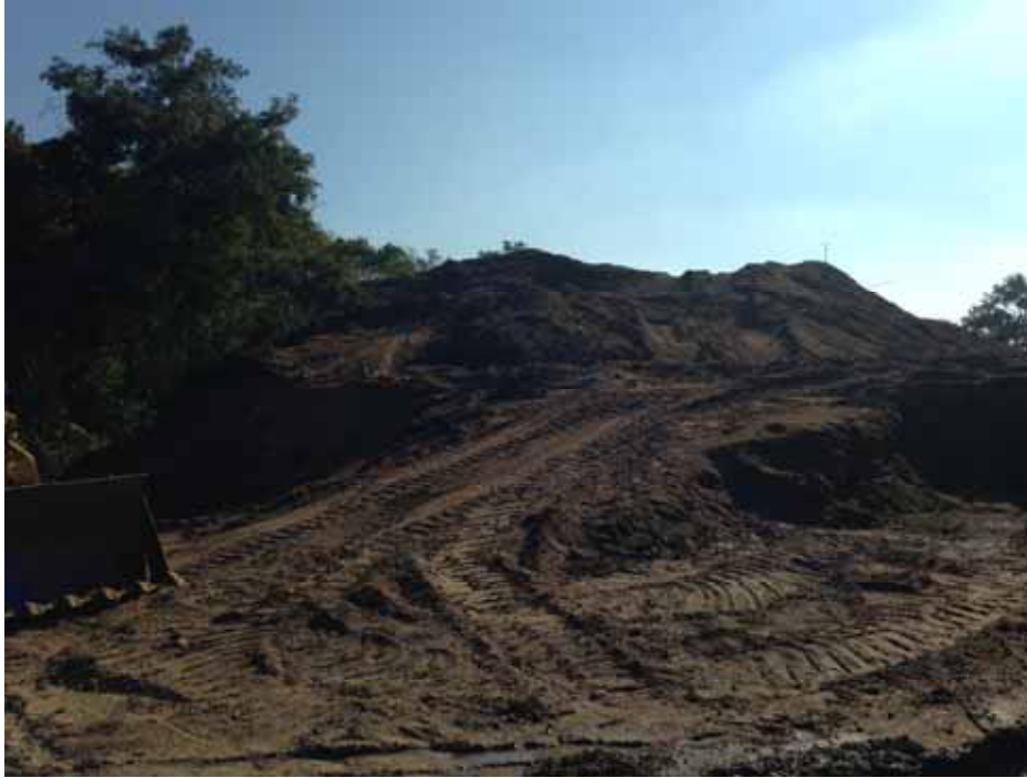
Photo of proposed backfill at Beth Moses Cemetery.
