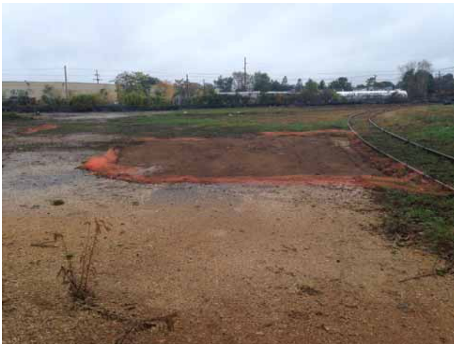
Backfill of Area 23B performed by Posillico.
