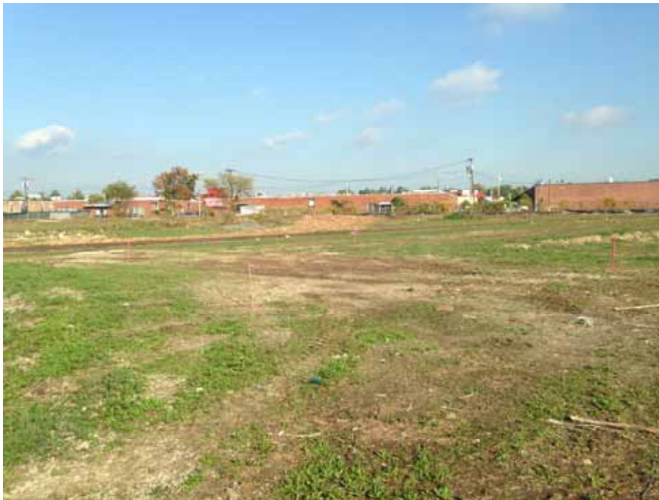
Pre-excavation survey mark out of Area 4C performed by Posillico's in-house surveyor.
