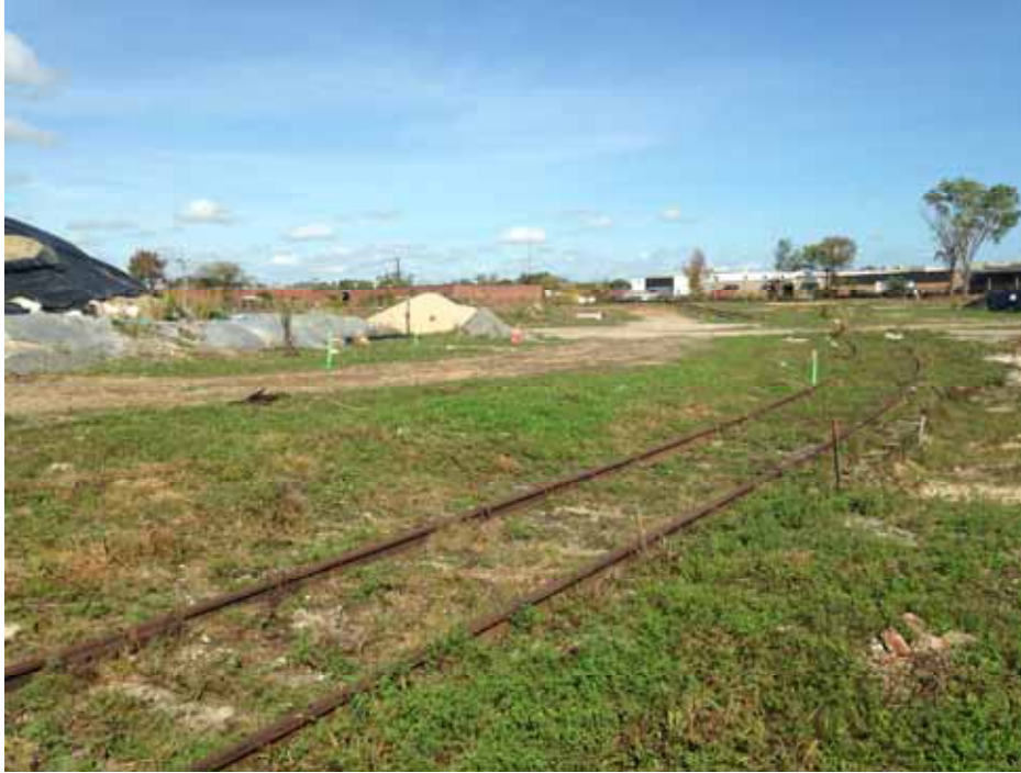
Pre-excitation survey mark out of Area 8C performed by Posillico's in-house surveyor.
