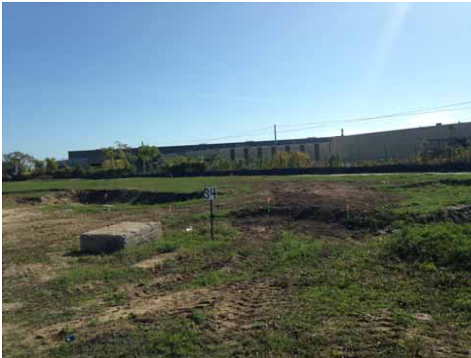
Pre-excitation survey mark out of Area 10C performed by Posillico's in-house surveyor.
