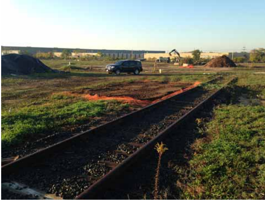
Backfill of east side of Area 6B performed by Posillico.
