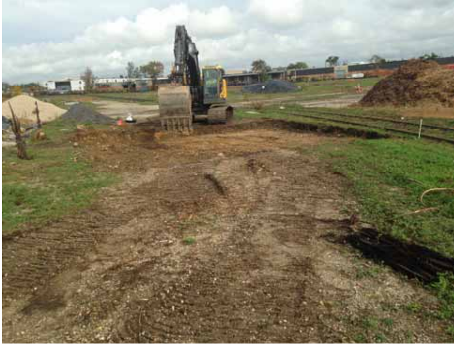
Posillico preforming excavation of Area 8C with GPS-enabled Volvo EC460CL Excavator.
