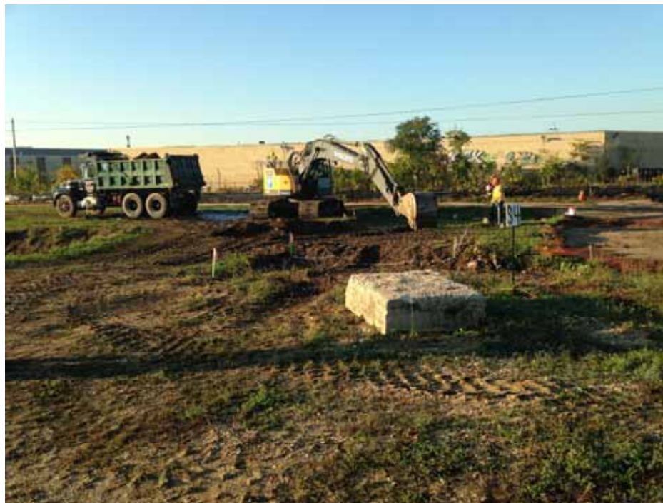
Posillico preforming excavation of Area 10C with GPS-enabled Volvo EC460CL Excavator.
