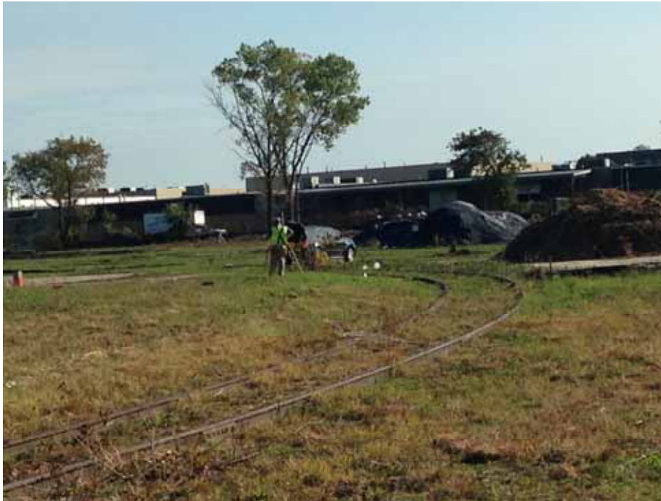
Survey activities being performed by Posillico's in-house surveyor.
