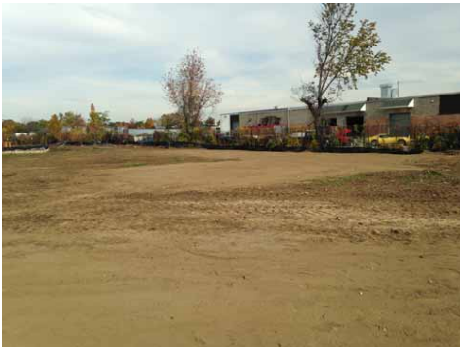
Completed backfill of Areas 4A and 2B performed by Posillico.
