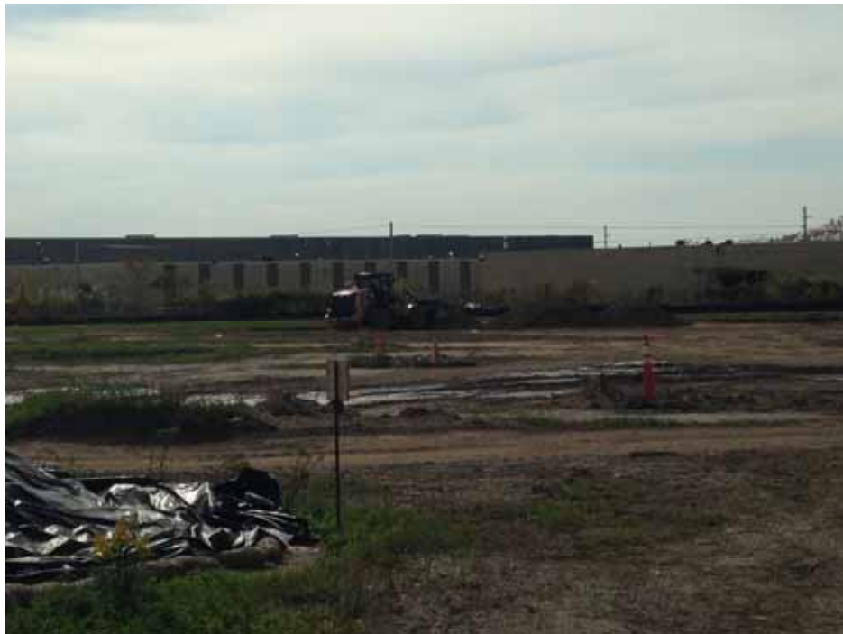
Posillico performing backfill of Area 34A with CAT 950K Loader.
