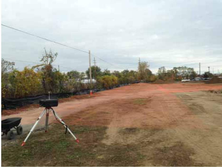
Demarcation layer installed in cap area by Posillico.
