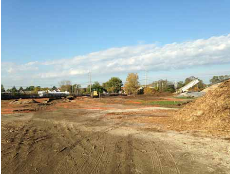
Posillico performing compaction of site wide cap with the Caterpillar 563 Dirt Roller.
