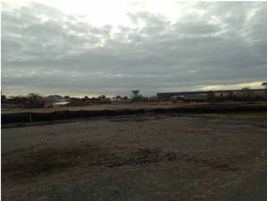
Posillico performing installation of site wide cap with GPS-enabled John Deere 850 Dozer.
