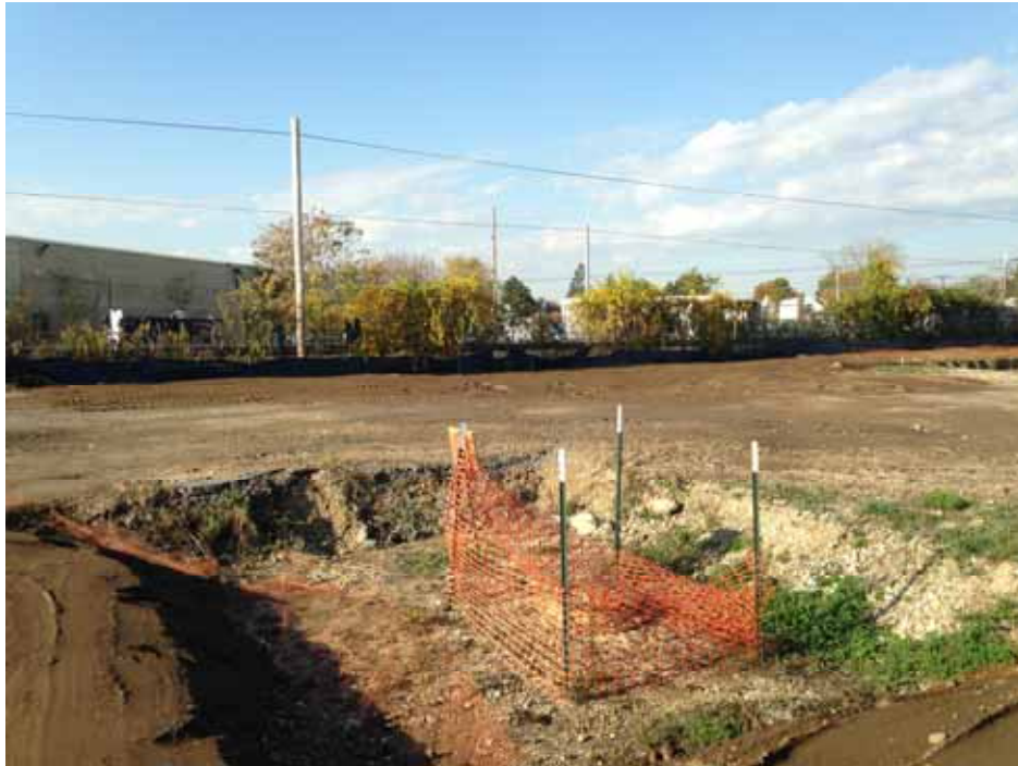
Completed backfill of Area 21B performed by Posillico.
