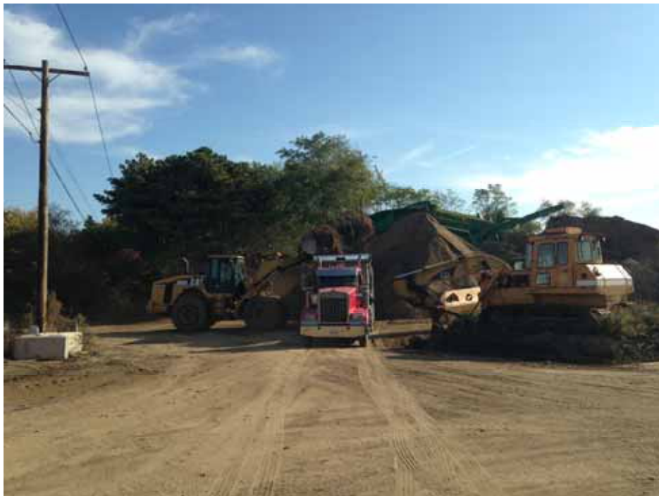
Truck being loaded with clean fill at Beth Moses Cemetery.
