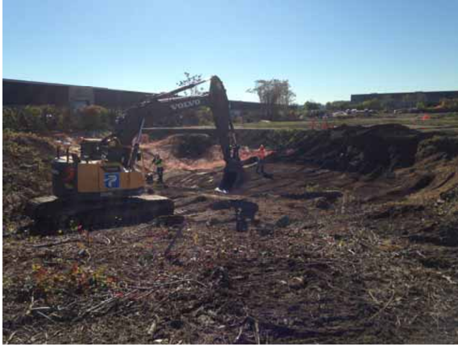
Posillico performing backfill of Area 6A with GPS-enabled Volvo EC460CL Excavator.
