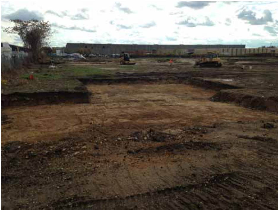
Completed excavation areas 12C and 13C.
