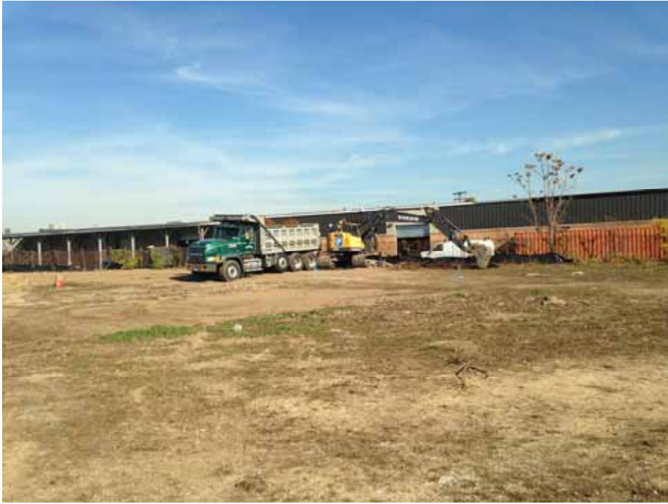
Posillico performing excavation of Area 12C with GPS-enabled Volvo EC460CL Excavator.
