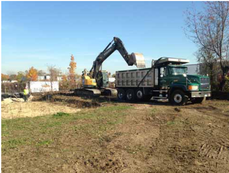
Posillico performing excavation of Area 2C with GPS-enabled Volvo EC460CL Excavator.
