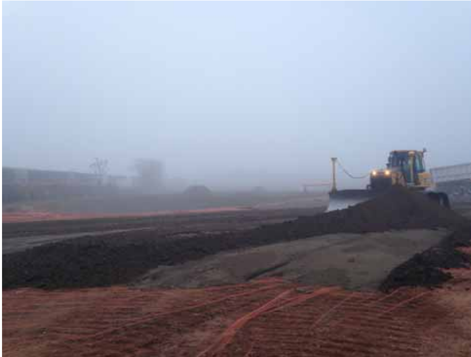
Grading the imported clean fill with a GPS-enabled John Deere 850 to construct the 8-inch cap base.
