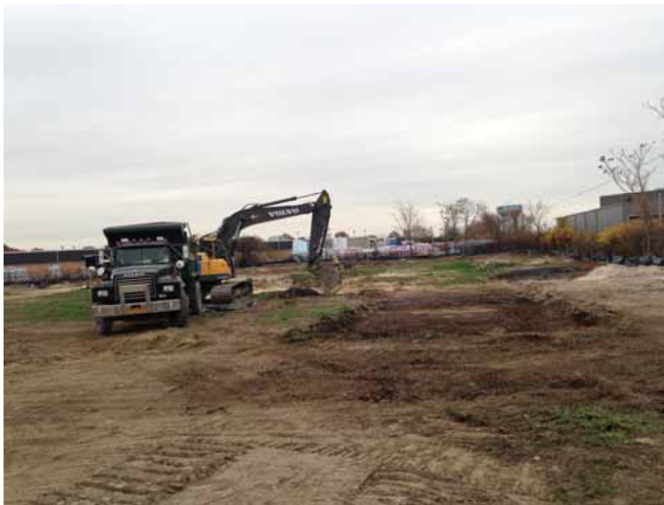
Posillico excavating soil from Area 17B-1 with a GPS-enabled Volvo EC460CL Excavator.
