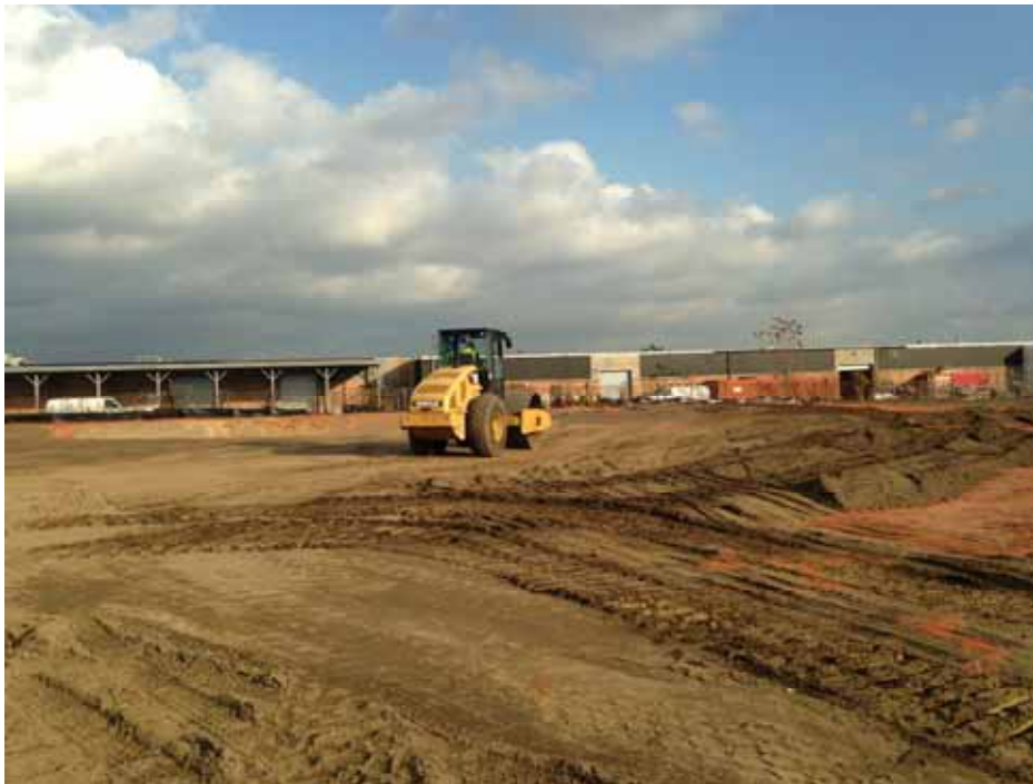
Posillico compacting the 8-inch cap base with a Caterpillar 563 Dirt Roller.
