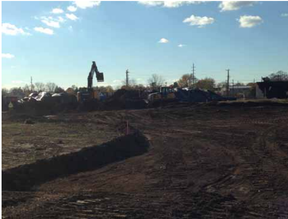
Posillico excavating soil from Area 23C with a GPS-enabled Volvo EC460CL Excavator.
