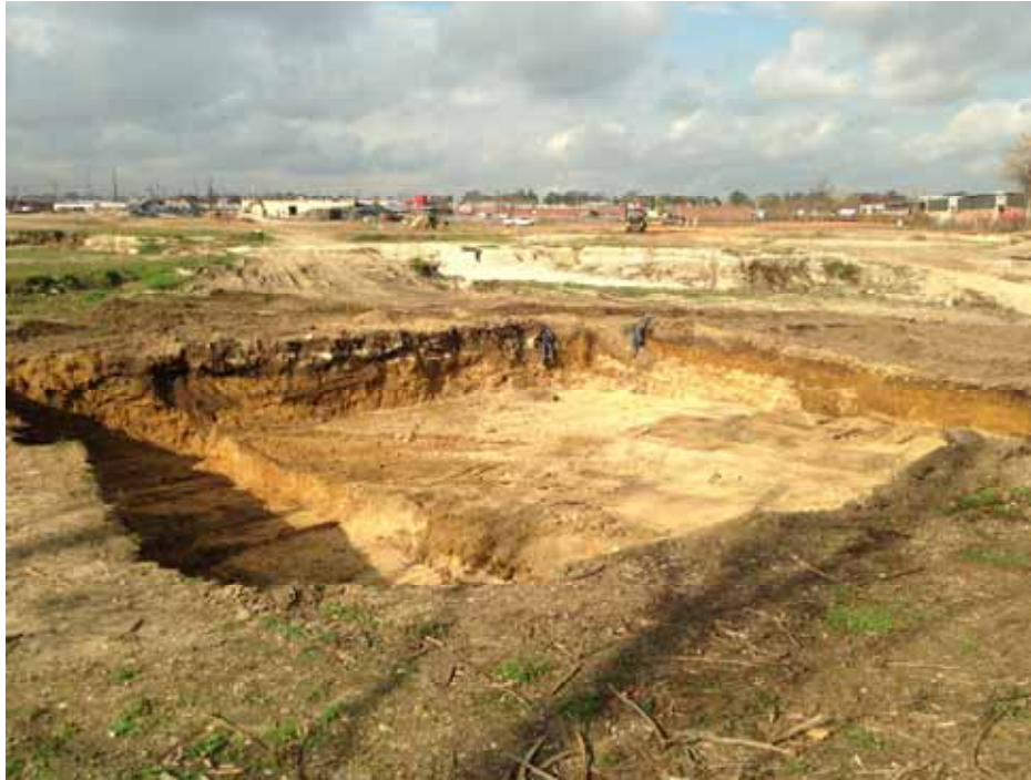
Completed "B" Group Excavation Area 16B-3.
