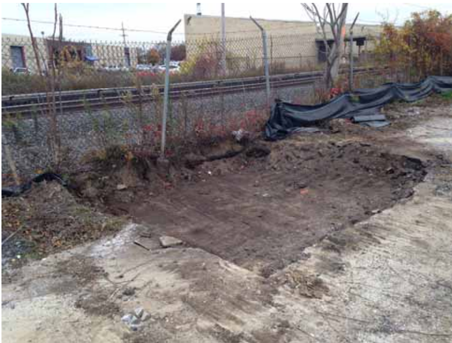
Completed "B" Group Excavation Area 17B-3.
