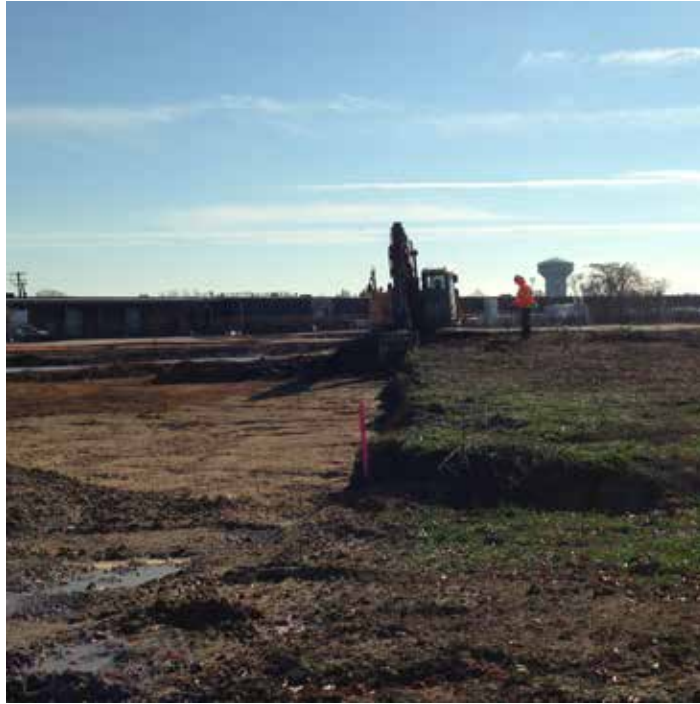
Posillico excavating soil from Area 23C with a GPS-enabled Volvo EC460CL Excavator.
