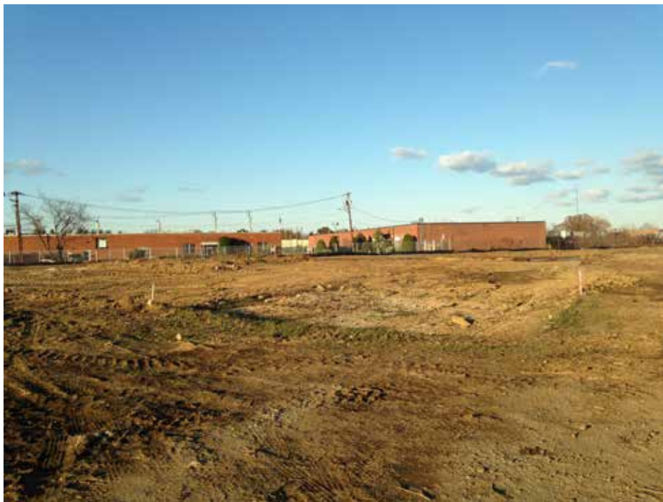
Completed "C" Group Excavation Area 23C.
