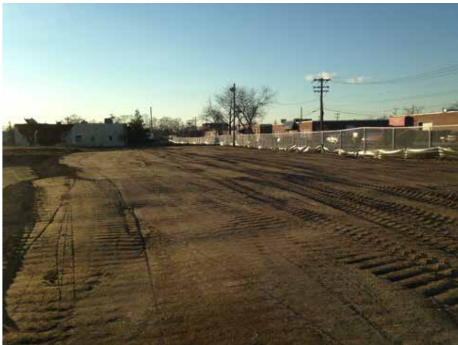
Completed backfill of "A" Group Excavation Area 1A.
