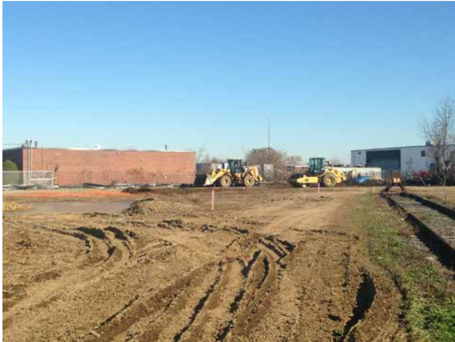
Posillico performing imported backfill material grading and compaction of areas 2A and 3A with GPS-enabled John Deere 850 Dozer and Caterpillar 563 Dirt Roller, respectively.
