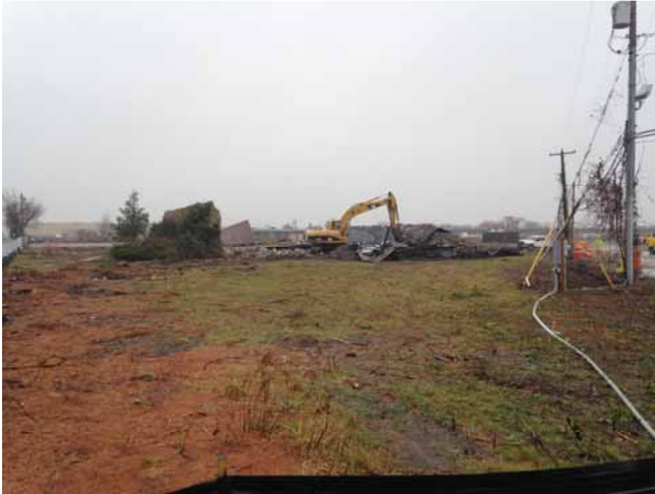
Posillico performing Administration Building Demolition.
