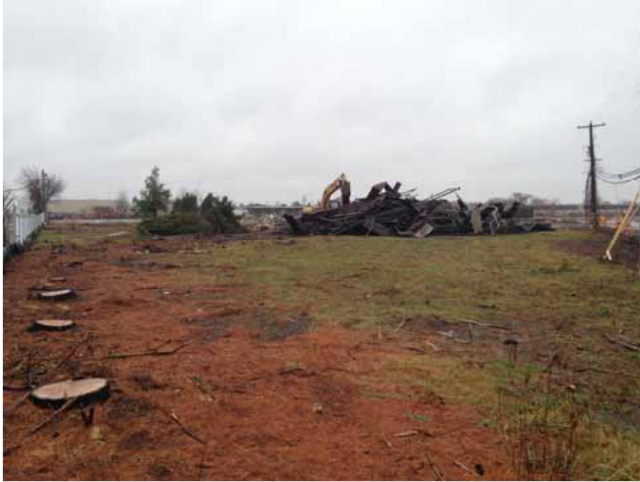
Administration Building Demolition status at the end of day on November 26, 2014.
