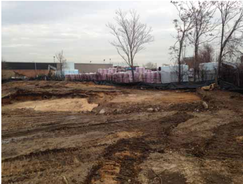
Completed "C" Group Excavation Area 25C.
