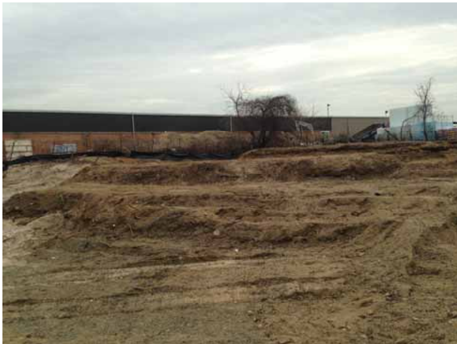
Completed "C" Group Excavation Area 19C.
