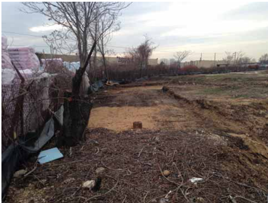
Completed "C" Group Excavation Area 26C.
