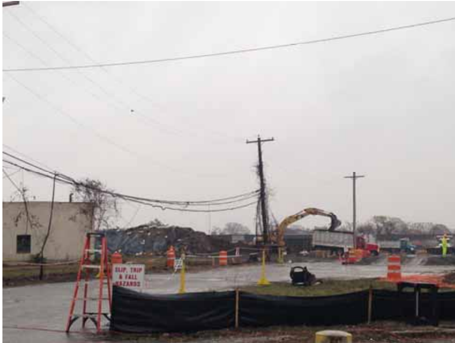
A truck being loaded with non-hazardous waste soil for offsite transportation and disposal at Gloucester County Landfill.
