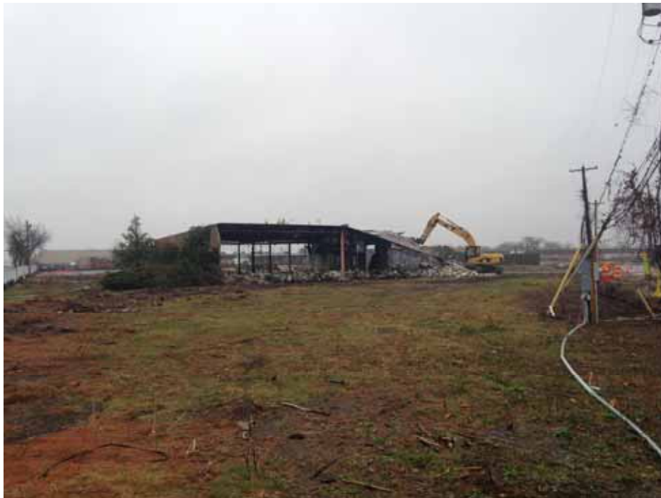
Posillico performing Administration Building Demolition.
