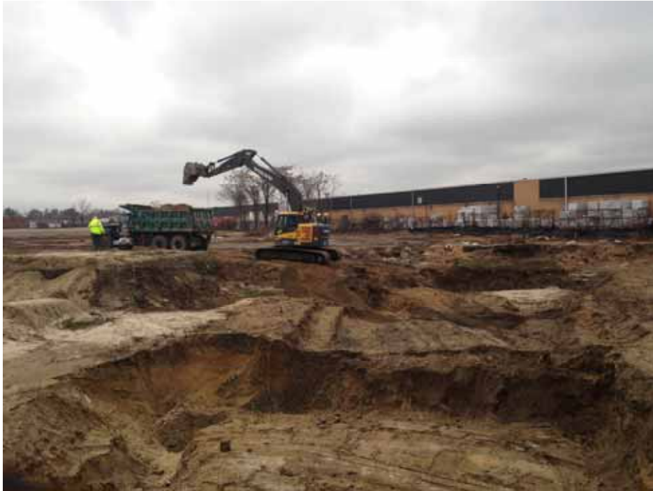
Posillico performing excavation of "A" Group Excavation Area 24A.
