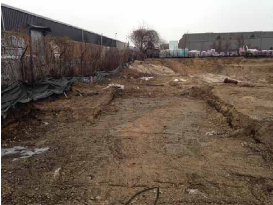
Completed "B" Group Excavation Area 16B-1.
