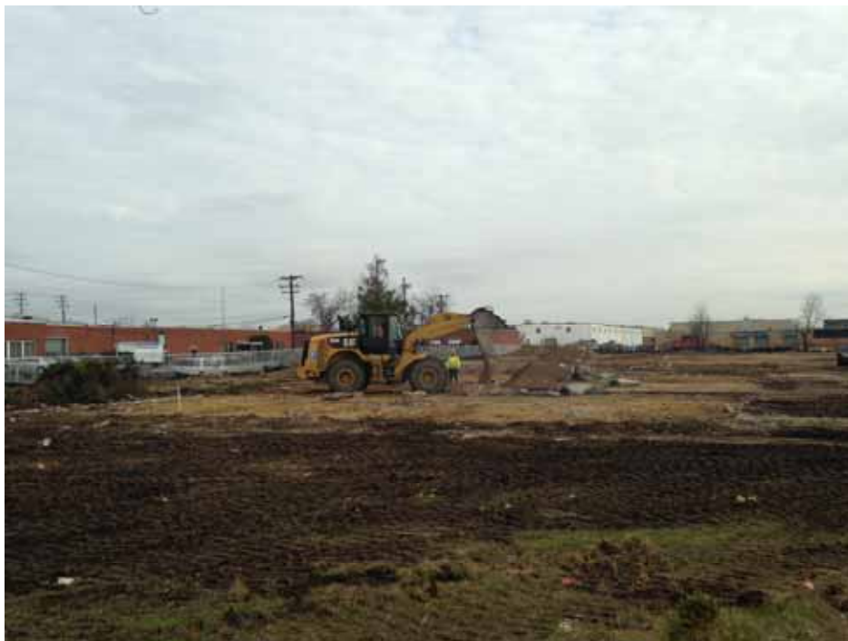
Posillico performing removal of Administration Building foundation.
