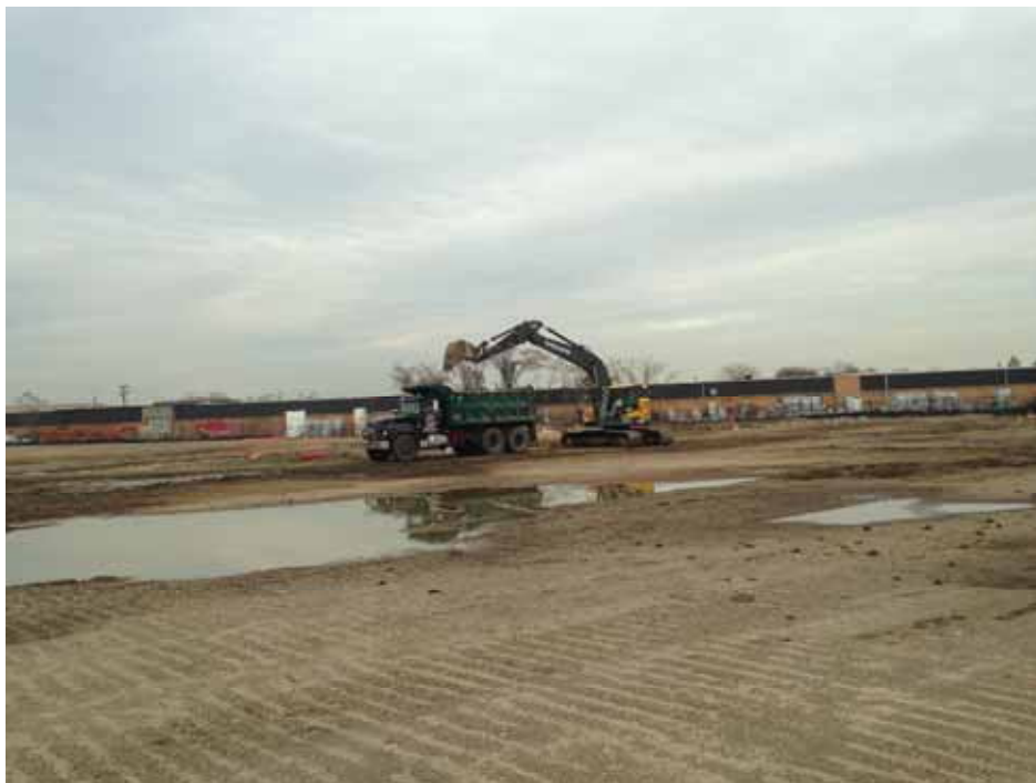
Posillico performing excavation of "A" Group Excavation Area 13A-1.
