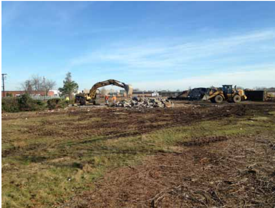
Posillico performing removal of Administration Building foundation.
