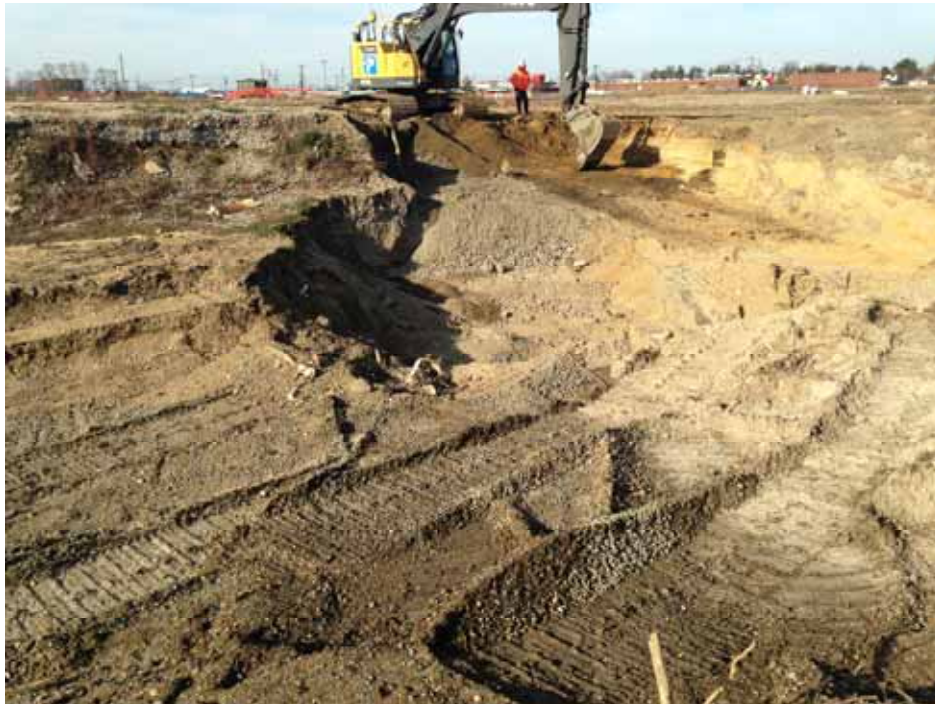
Posillico performing excavation of "A" Group Excavation Area 21A.
