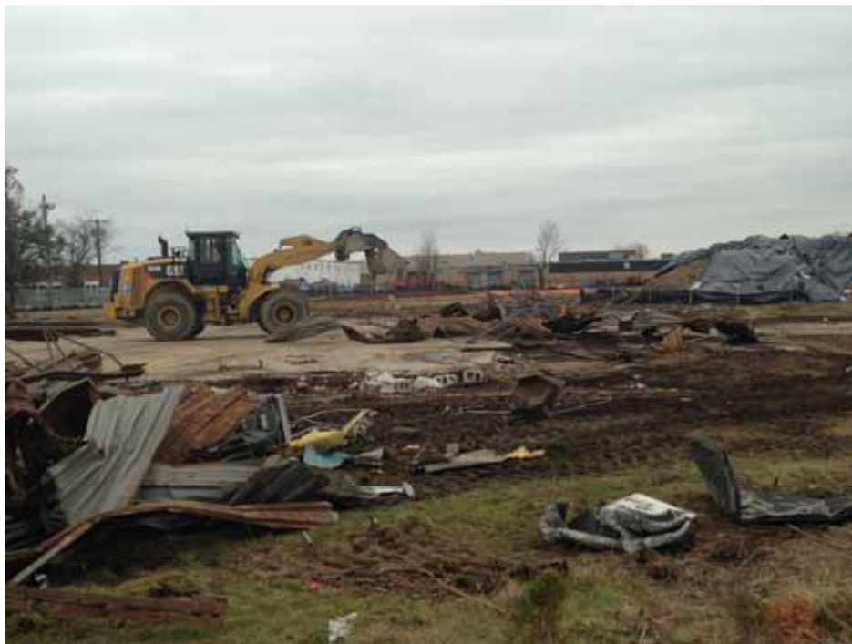
Posillico performing segregation of Administration Building concrete and masonry debris and scrap metal.
