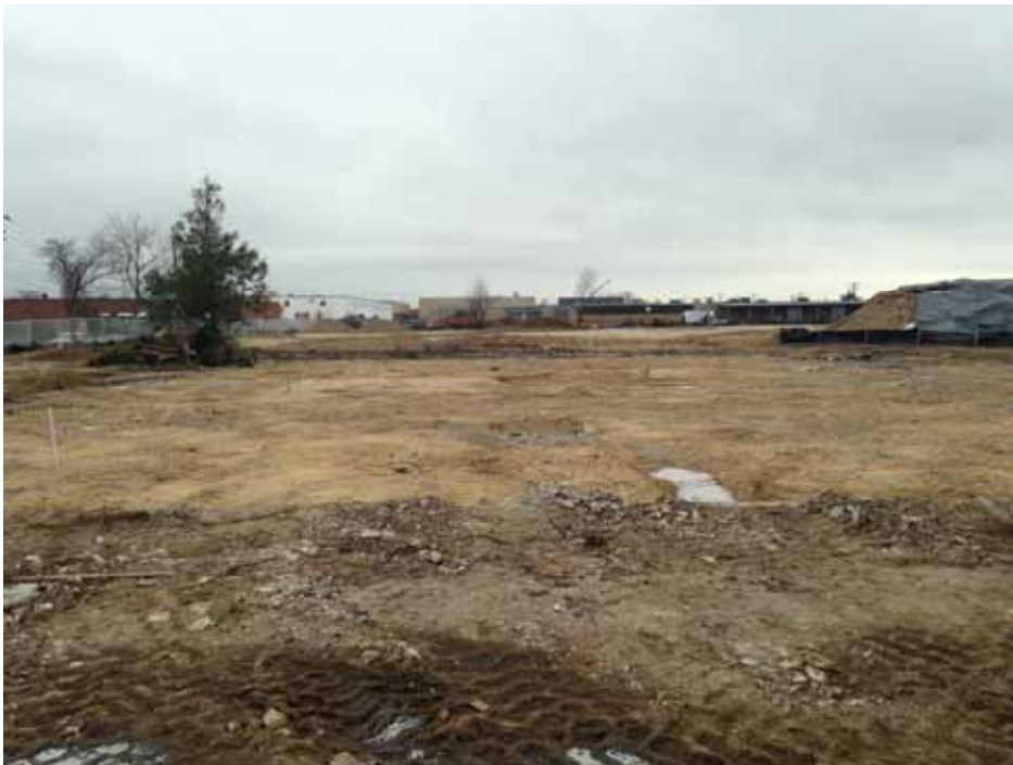
Administration Building footprint after concrete slab removal.
