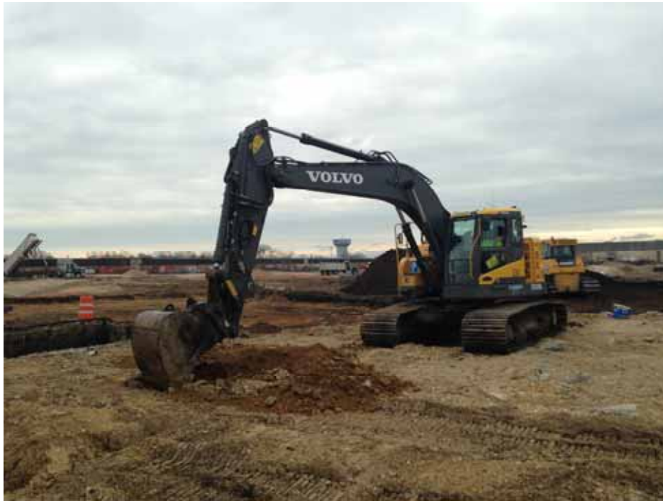
Posillico preforming test pit in Administration Building footprint.
