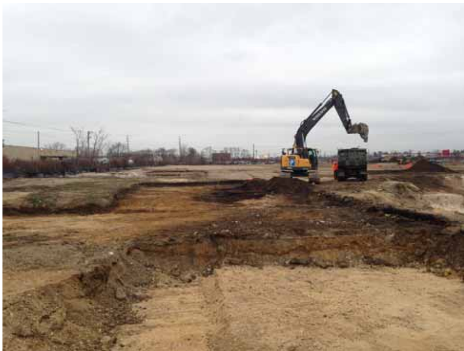
Posillico performing excavation of "B" Group Excavation Area 17B-2
