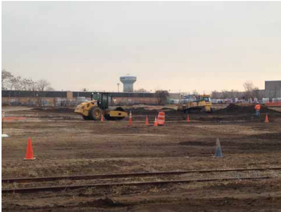
Posillico performing installation of 8 inch base cap.
