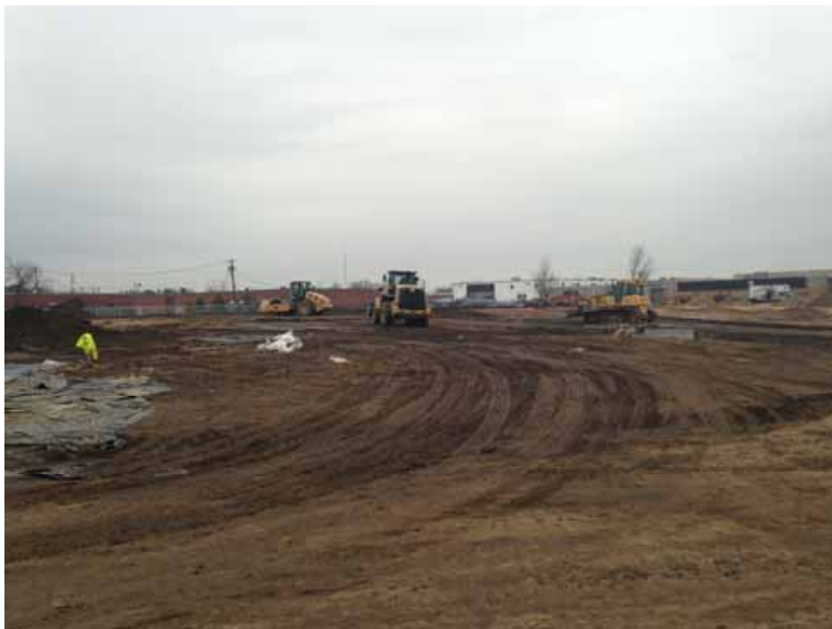
Posillico performing installation of 8 inch base cap.
