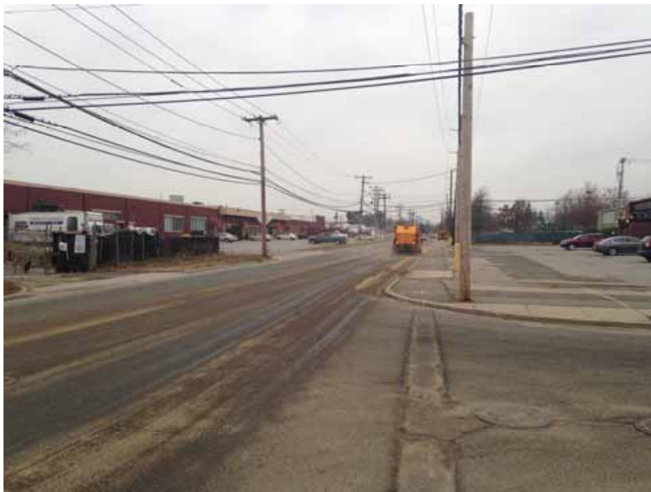
Street sweeper conducting road cleaning on New South Road.
