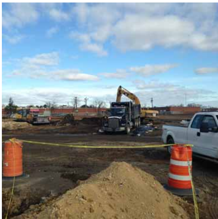
A truck being loaded with non-hazardous waste soil for offsite transportation and disposal at Gloucester County Landfill.
