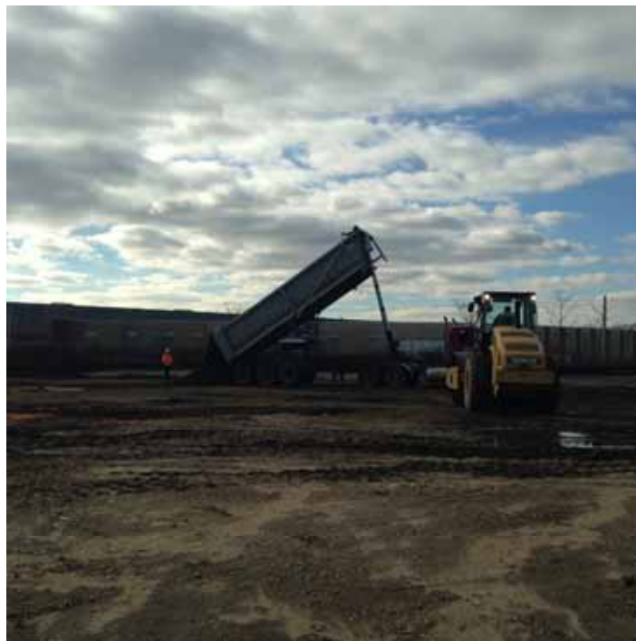
Posillico performing delivery of clean backfill.
