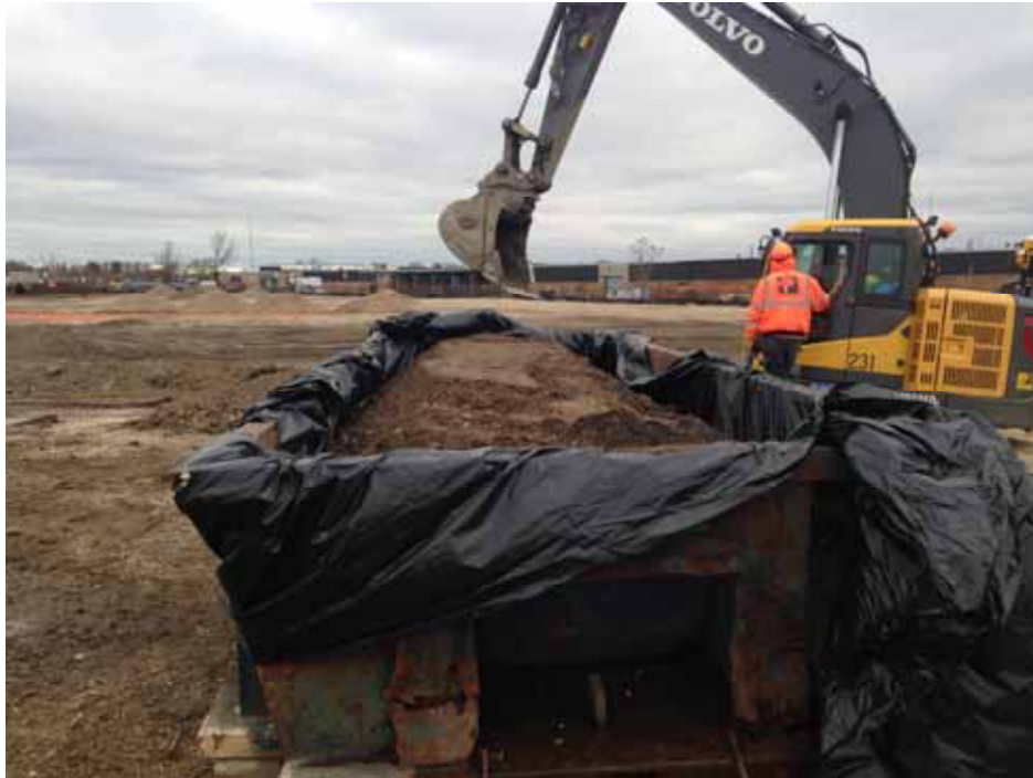
Excavated visually stained/discolored soil from "A" Group Excavation Area 13A-1.
