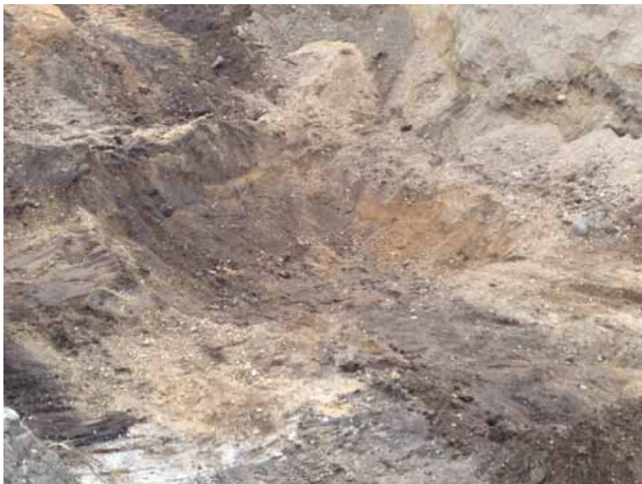
Completed excavated visually stained/discolored soil from "A" Group Excavation Area 13A-1.
