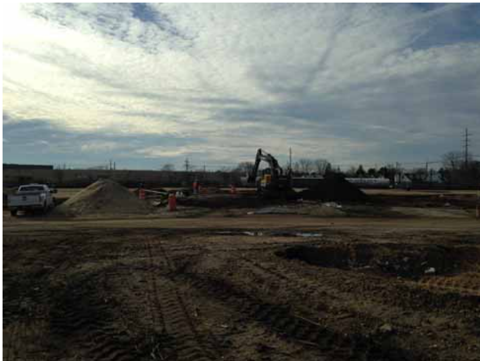
Posillico performing excavation of "C" Group Excavation Area 7C.
