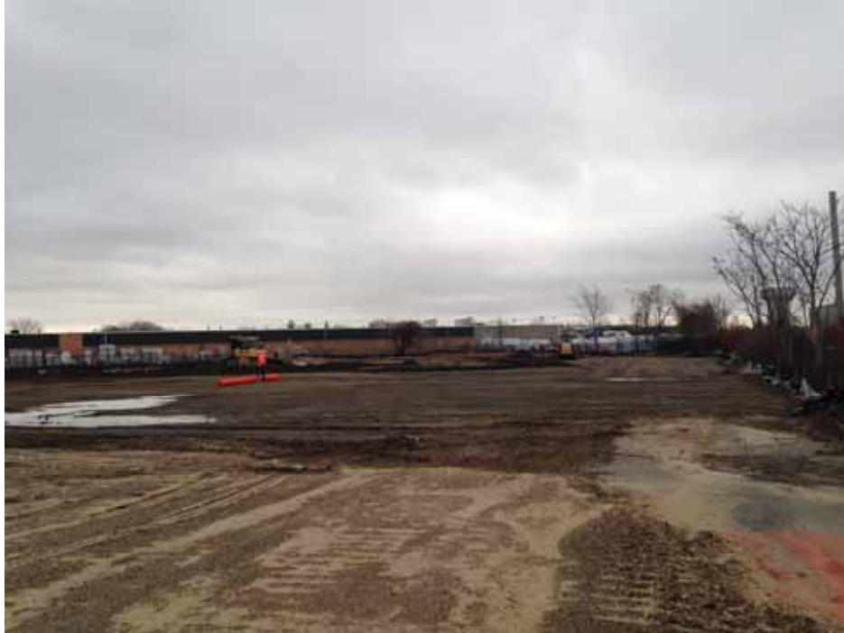
Posillico performing installation of 8 inch base cap.
