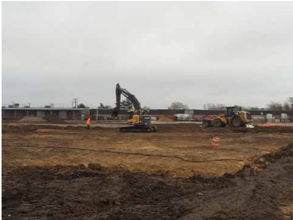
Posillico performing excavation of "C" Group Excavation Area 24C.
