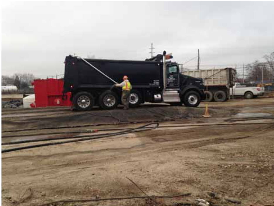
Posillico performing decontamination of a truck loaded with non-hazardous waste soil.
