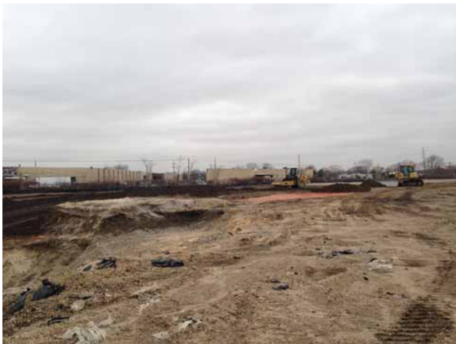
Posillico performing backfill of "A" Group Excavation Areas 26A and 27A.
