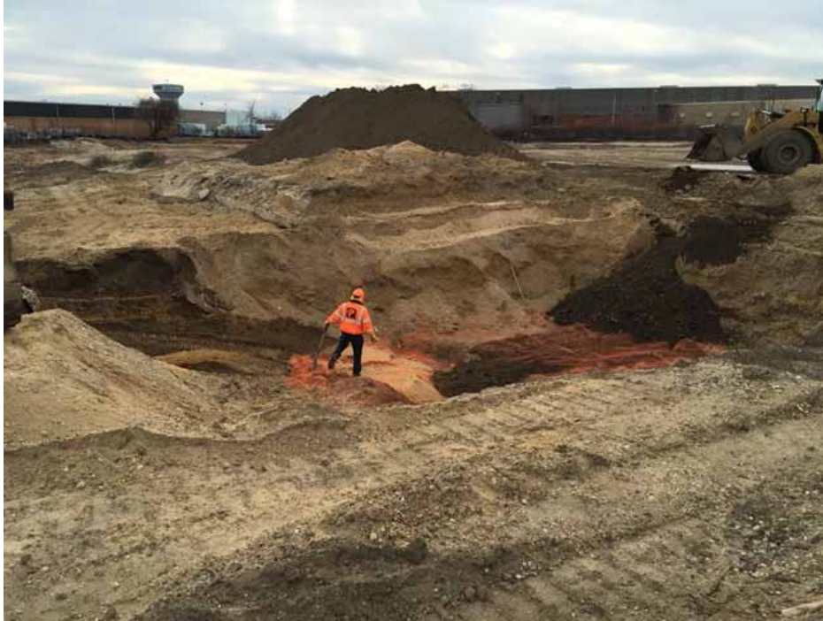
Posillico performing backfill "A" Group Excavation Areas 13A-1 and 13A-2.
