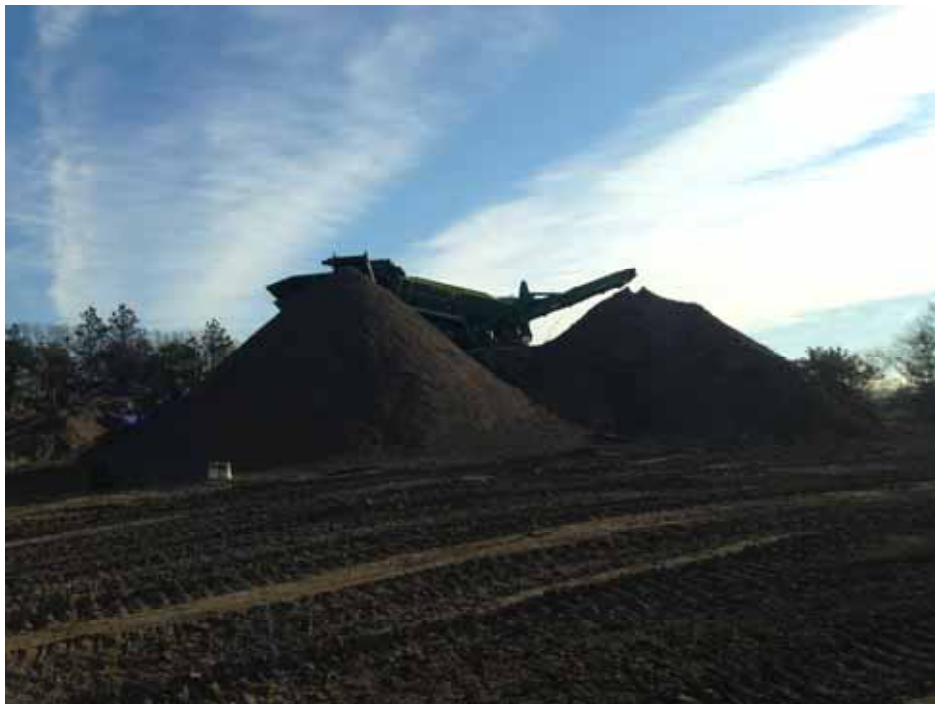
Clean fill soil screening being conducted at Beth Moses Cemetery.
