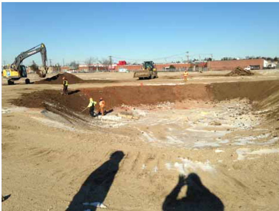
Posillico performing installation of 8 inch base cap in Sump No. 1.
