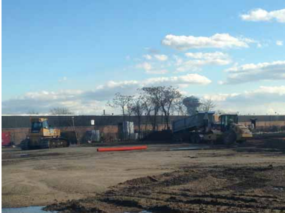
Posillico accepting delivery of clean backfill and performing installation of 8 inch base cap.
