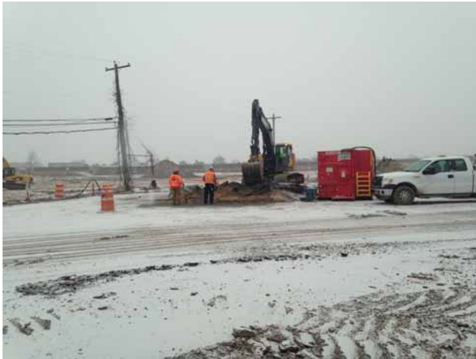
Posillico performing removal of decontamination pad.
