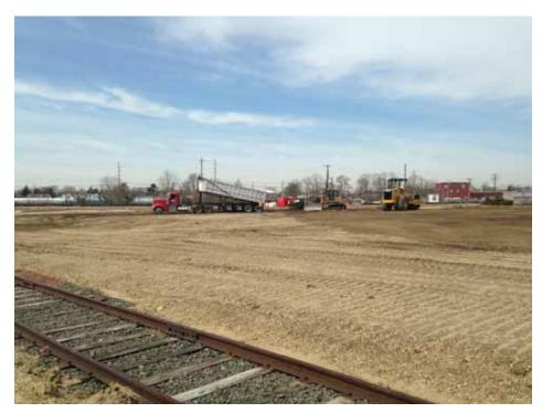
Posillico accepting delivery of clean backfill and performing backfill of "C" Group Excavation Area 24C.
