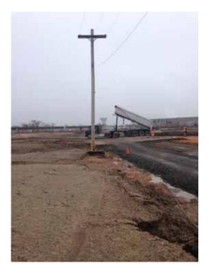
Posillico accepting delivery of clean backfill and performing backfill of "C" Group Excavation Area 7C.
