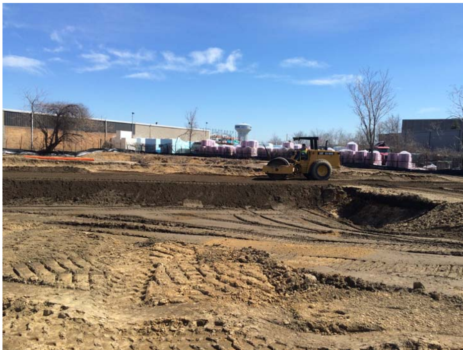
Backfill in progress in “C” Group Excavation Area 19C.
