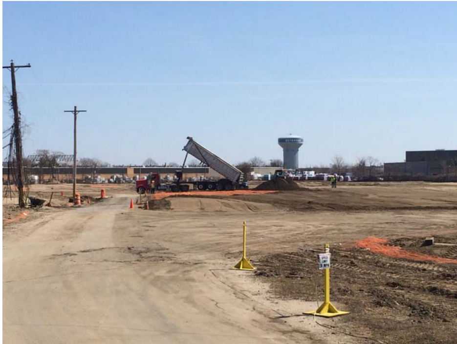
Posillico performing installation of 8-inch base cap.
