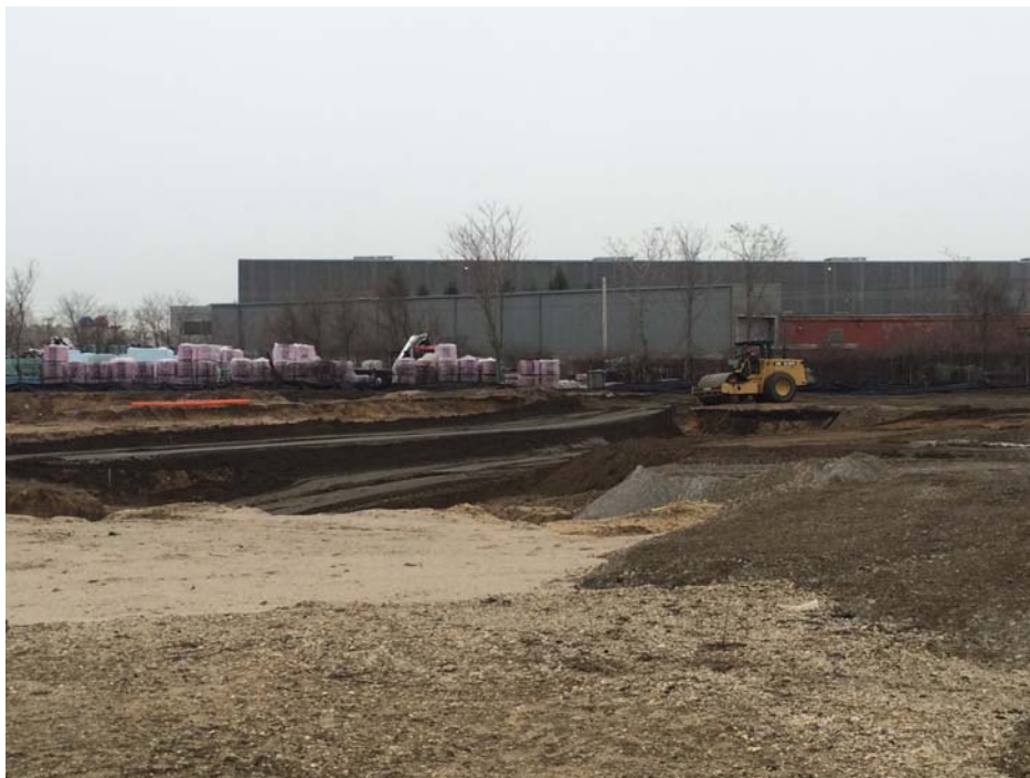
Posillico performing backfill of "C" Group Excavation Area 19C.
