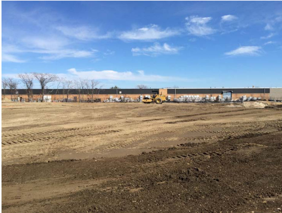
Posillico performing compaction of backfill in southeastern re-grade area
