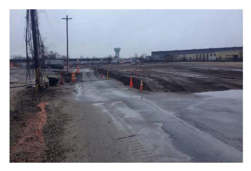
Posillico accepting delivery of clean backfill but no grading occurred due to wet conditions.
