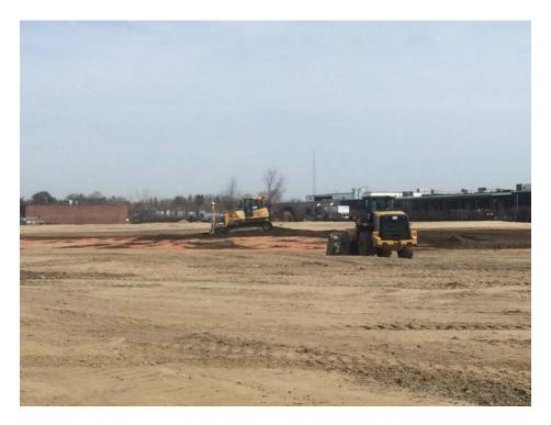
Posillico performing installation of 8-inch soil base cap.
