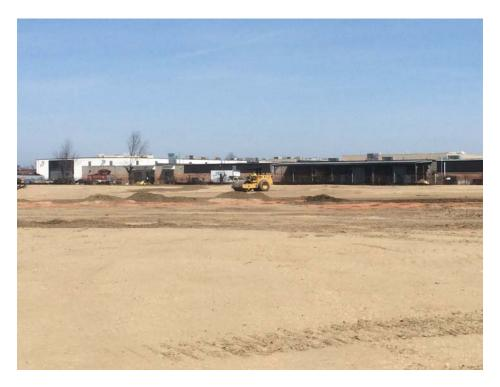
Posillico performing compaction of 8-inch soil base cap.
