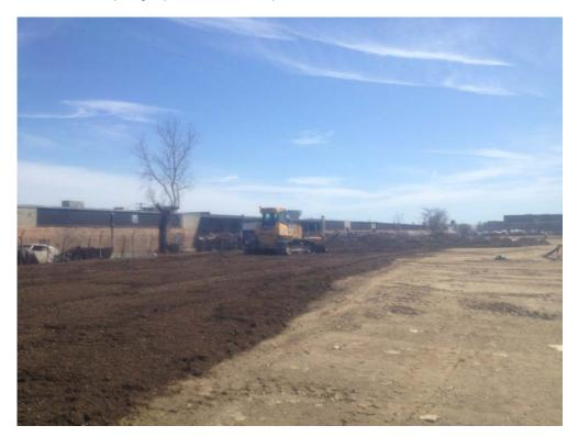
Posillico grading topsoil on eastern side of the Site.
