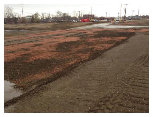
Posillico performing compaction of 8-inch soil base of cap (southeast corner of Site).
