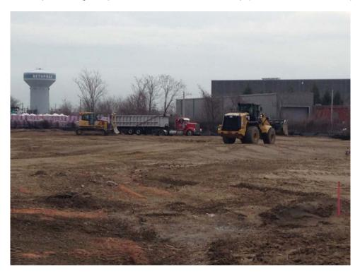
Posillico moving backfill to Sump #4 located in the southeast corner of the Site.
