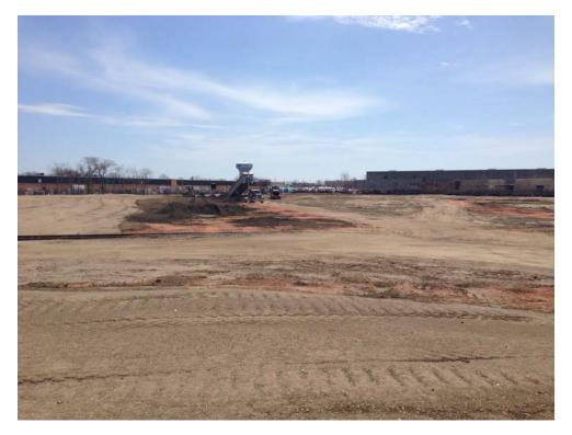
Posillico performing installation of 8-inch soil base of cap.
