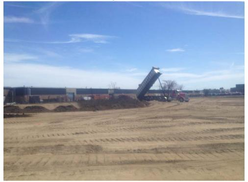
Posillico stockpiling topsoil for the sumps located in the southern corner of the Site.
