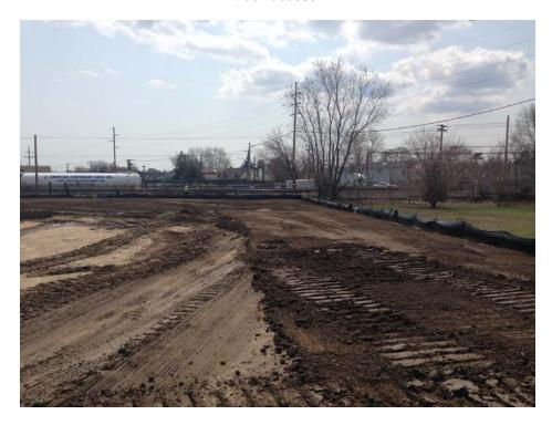
Posillico spreading topsoil across the southwest portion of the Site.
