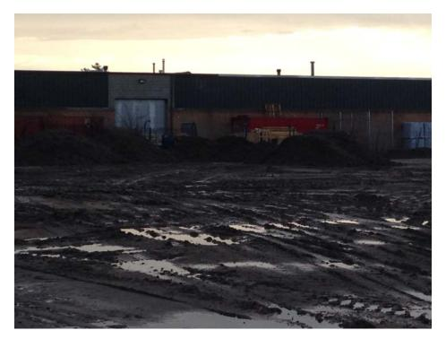
Posillico stockpiling topsoil until the rainfall stopped and conditions were favorable for grading.
