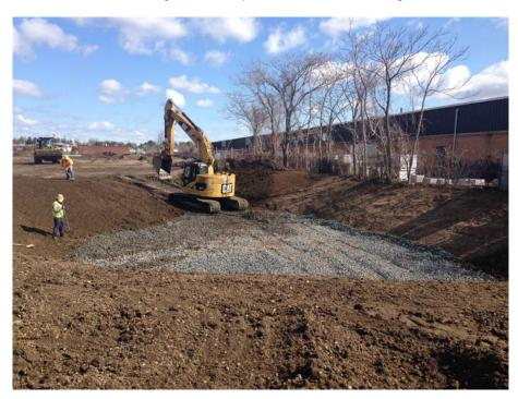
Posillico placing washed crushed limestone in the bottom and topsoil on the sides of Sump #2.
