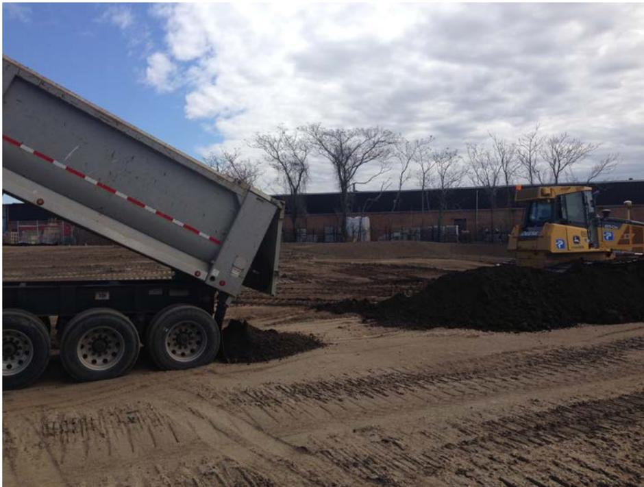
Posillico stockpiling topsoil adjacent to Sump #3.
