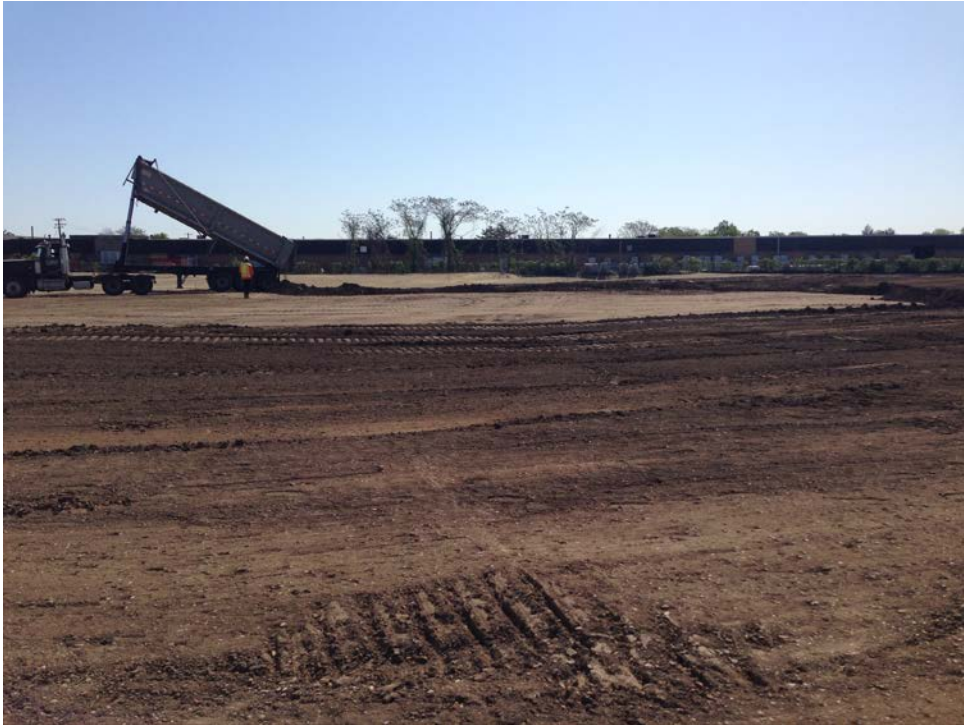
Posillico stockpiling topsoil in the southeastern corner of the Site.
