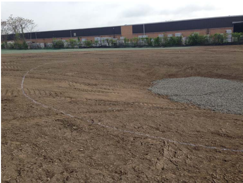
Posillico marking area to place the erosion control blankets in Sump #3.
