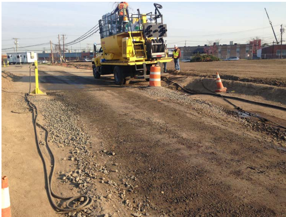
Hydroseed mixture being prepared for application.
