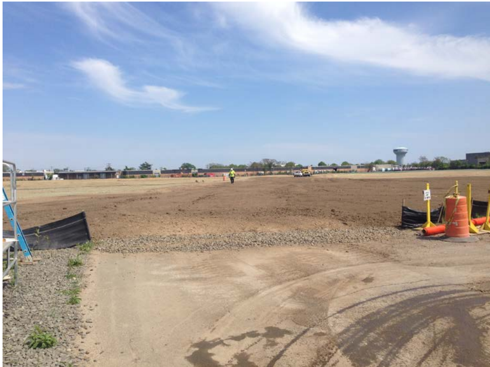
View of site from northwest asphalt parking lot showing the completed soil cover ready for hydroseeding.
