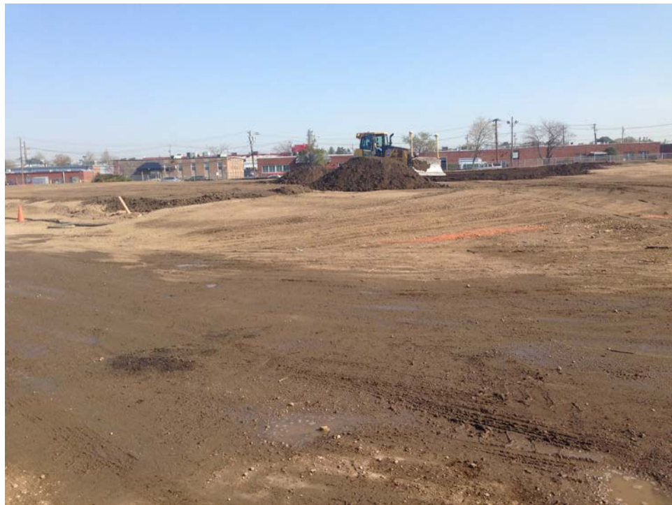
Posillico stockpiling topsoil near the middle of the Site.
