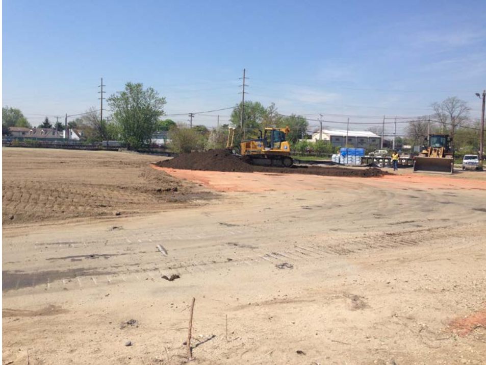
Posillico spreading general fill after placing the demarcation layer.
