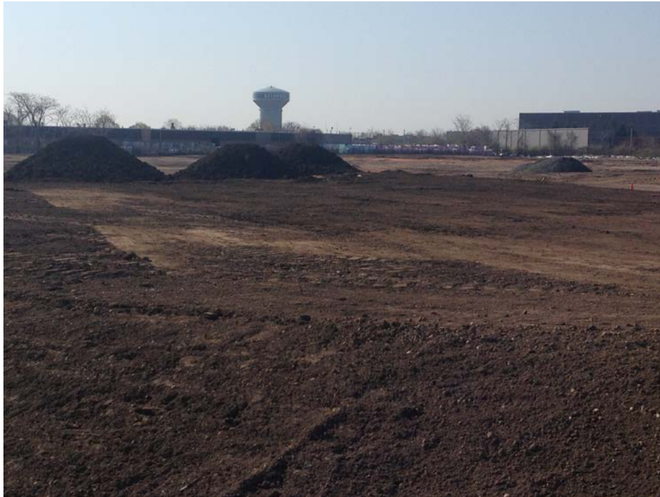
Posillico spreading topsoil across the middle of the property west of the railroad spur.
