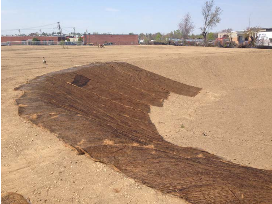
Posillico installing erosion blankets at Sump #1.
