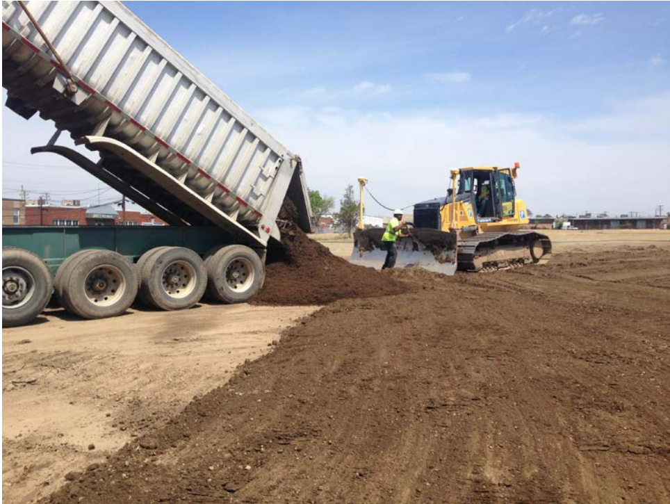
Posillico grading the final load of topsoil.
