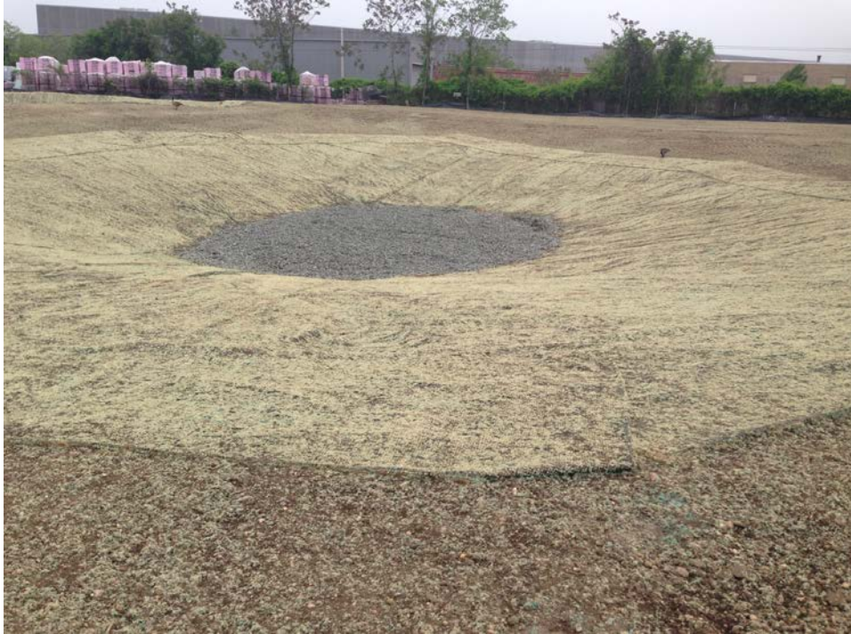
Posillico installing erosion control blanket in Sump #3.
