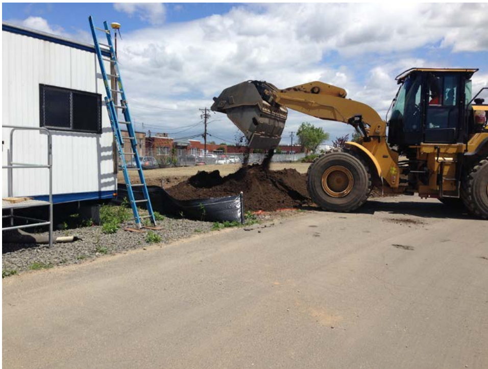
Posillico placing fill along the northwestern limit of the soil cover.
