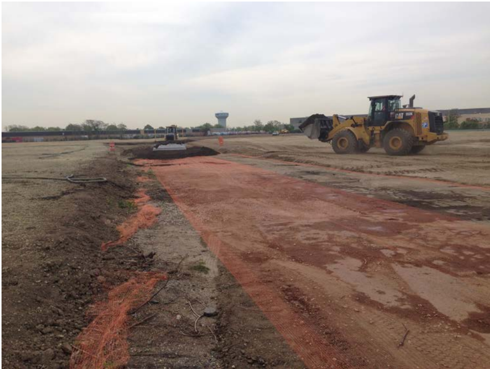
Posillico grading general fill over a demarcation layer across the truck tire wash area/site access road (remaining portion of Excavation Area 24C).
