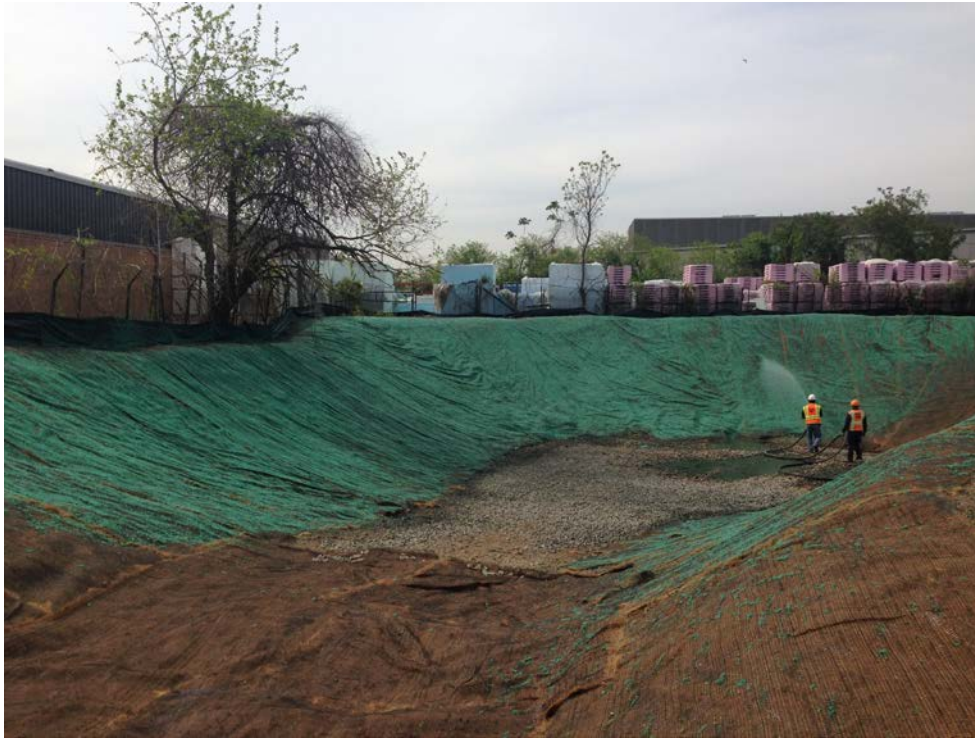
Posillico hydroseeding Sump #4 after placing the erosion control blanket.
