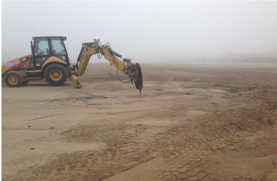
Posillico using a hoe ram to puncture holes in the asphalt pavement area before placing the soil cover system.
