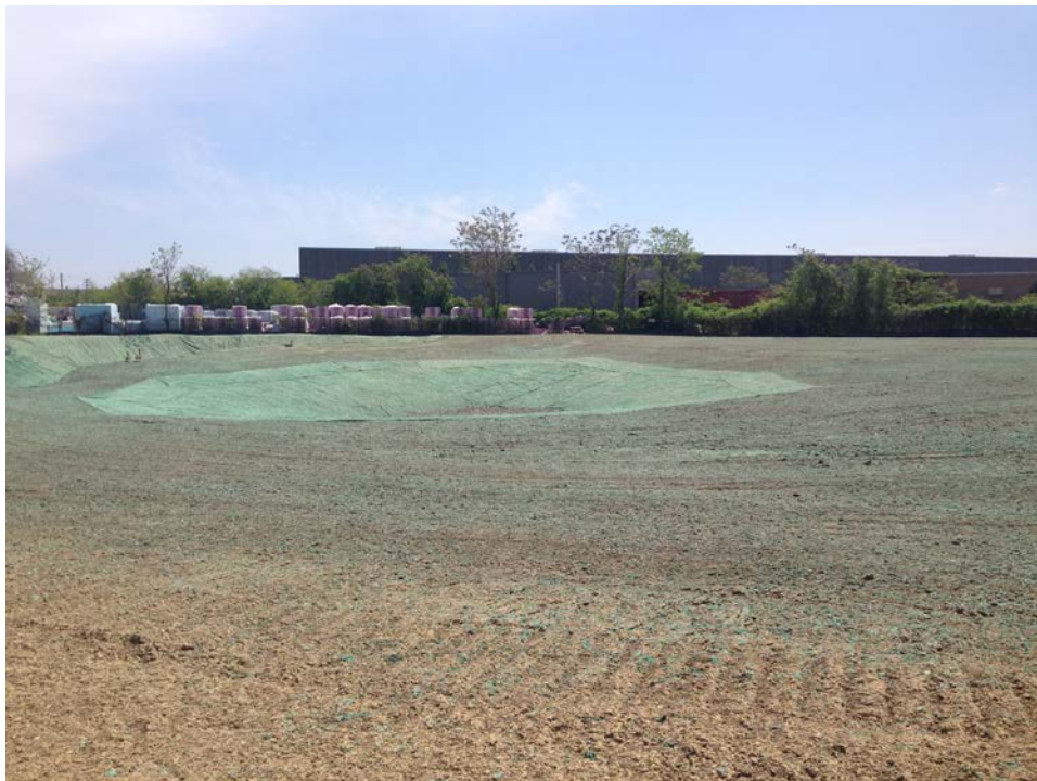
Hydroseeding completed in areas surrounding Sumps #3 and #4 (southeast corner of Site).
