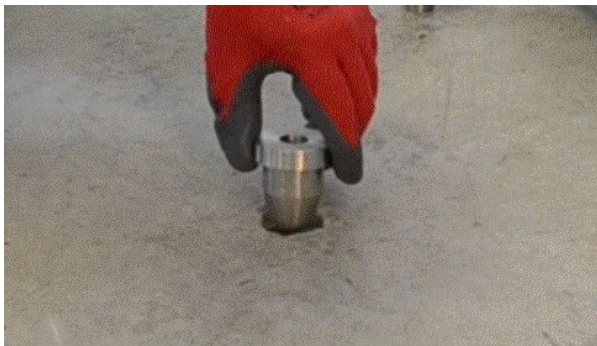
Figure 3. Testing Depth with the Drilling Guide.
