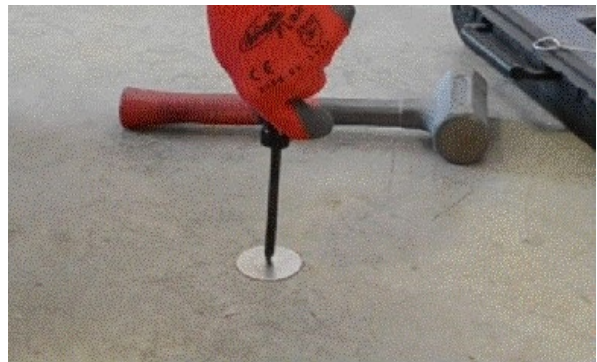
Figure 5. Tightening the Secured Cover.
