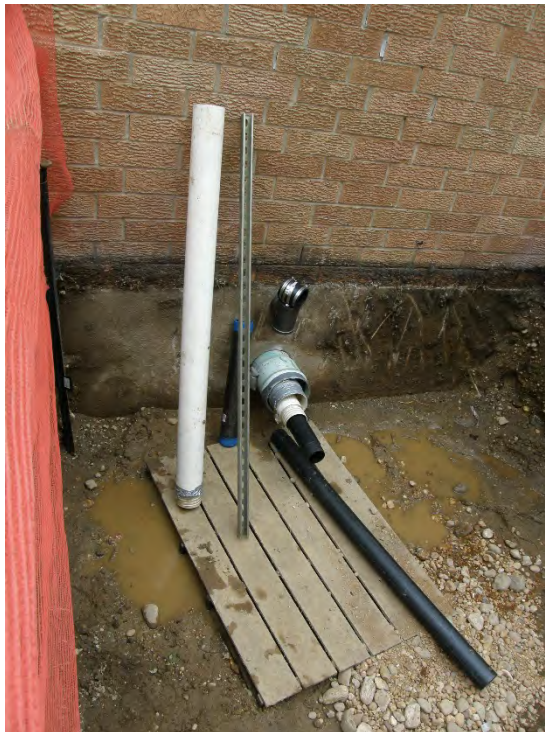
Photo 2 - Casing pipes and 3-inch extraction pipe after installation
