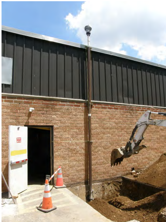
Photo 6 - Completed riser pipe with "downspout" cover. Backfilling ongoing.
