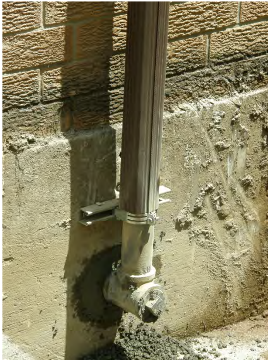
Photo 5 - Sealed corehole through foundation wall
