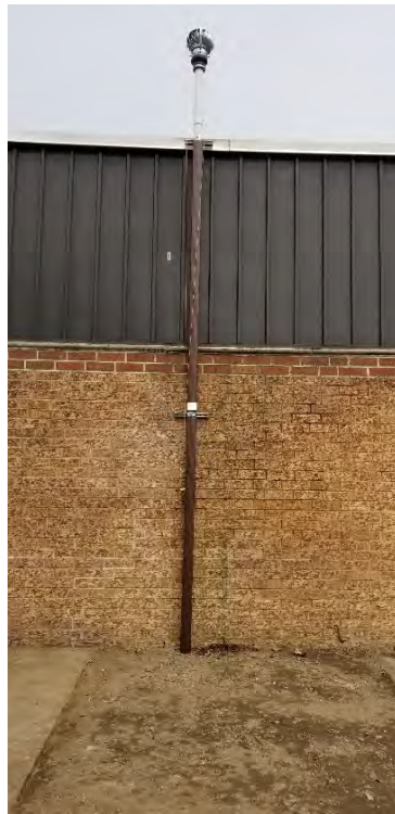
Photo 5 - Completed installation at SSD-1
