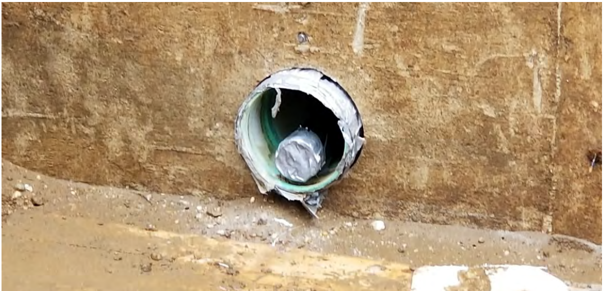
Photo 2 - Casing pipes and 3-inch extraction pipe during installation at SSD-6
