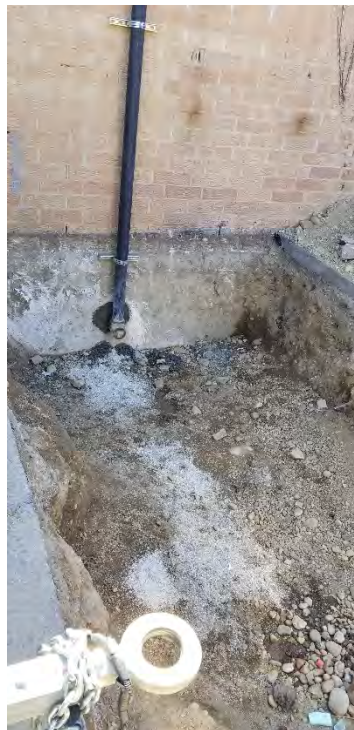
Photo 4 - Riser Pipe at SSD-2
