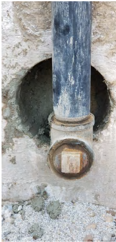
Photo 3 - Connection between vertical riser and horizontal pipe at SSD-2
