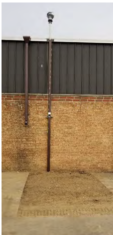
Photo 7 - Completed installation at SSD-3
