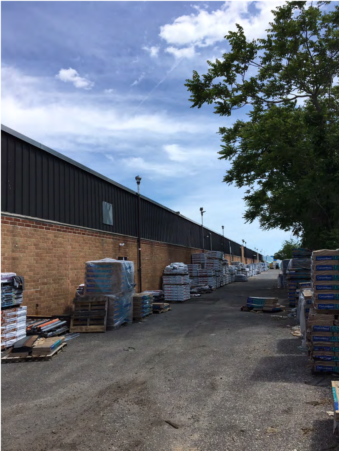
Photo 11 – Completed system – view looking south
