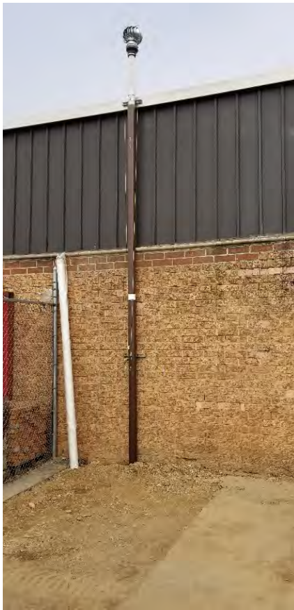
Photo 9 - Completed installation at SSD-6
