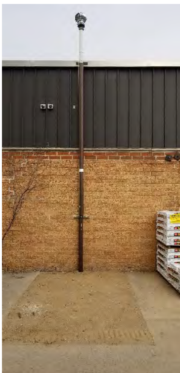
Photo 8 - Completed installation at SSD-4
