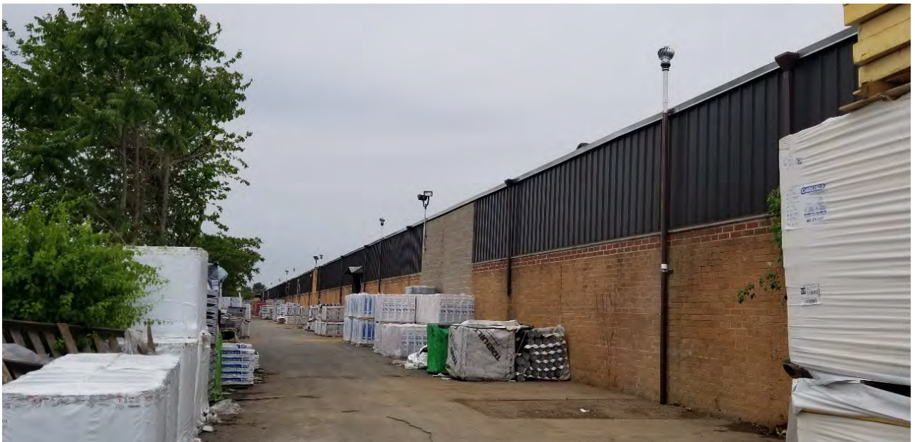
Photo 10 - Completed system – view looking north
