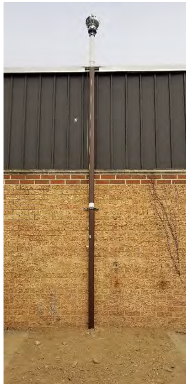
Photo 6 - Completed installation at SSD-2
