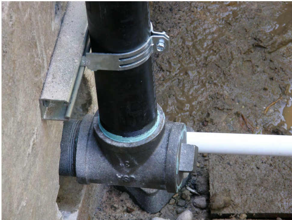
Photo 3 - Connection between vertical riser and horizontal pipe
