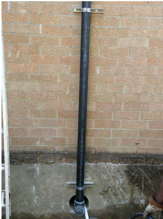
Photo 3 - Connection between vertical riser and horizontal pipe
