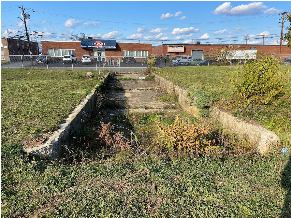
Photograph 4: Looking north, concrete loading dock.
