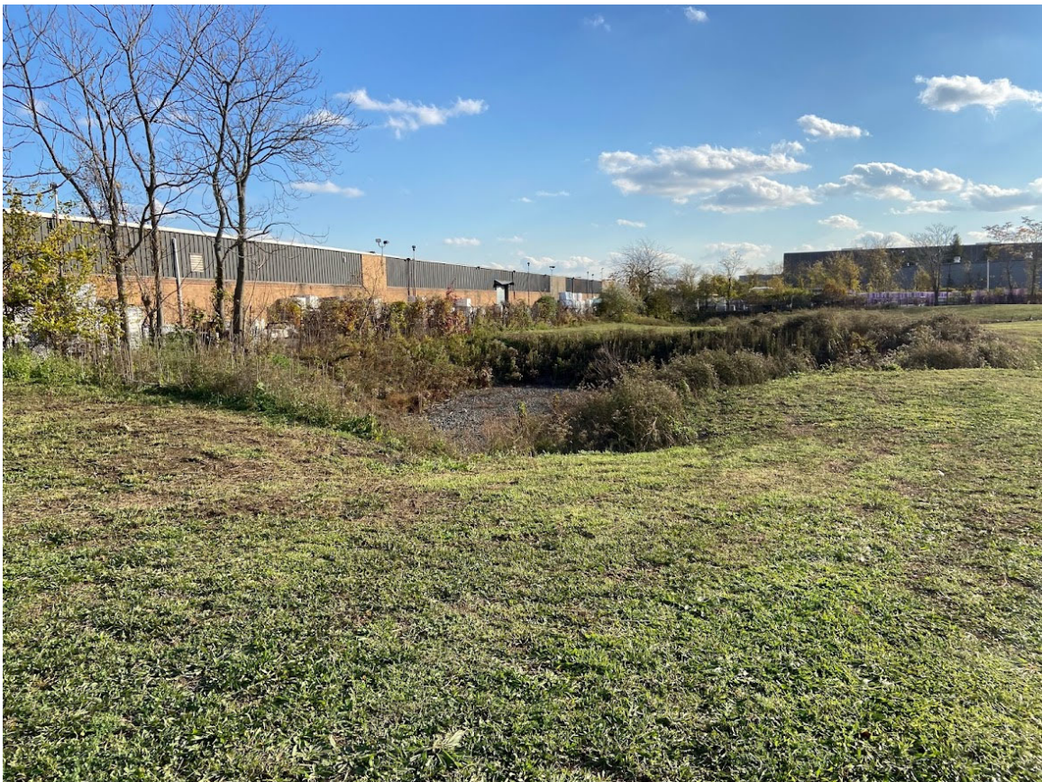
Photograph 8: Looking southeast, location of Sump-2.
