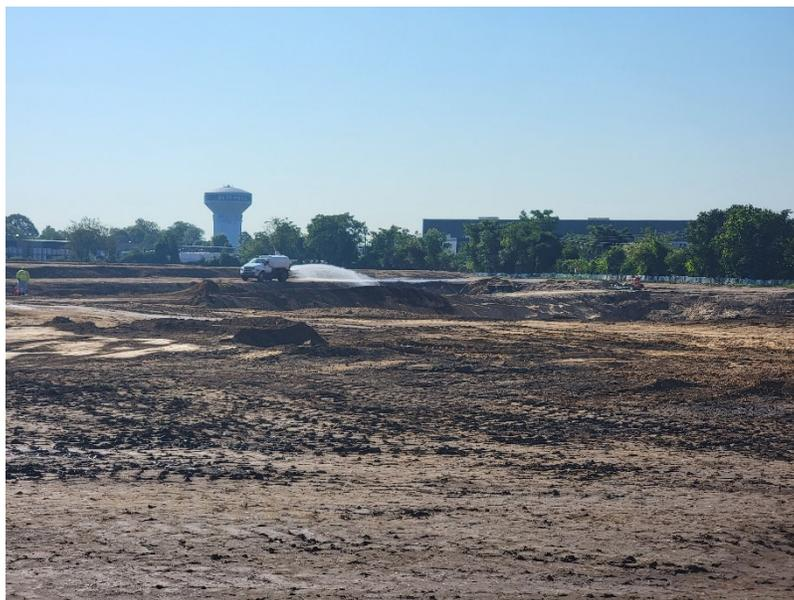
**Photo 2:** Looking south, Pratt continues excavation to subgrade for future parking lot area. Water truck in distance for dust mitigation.
