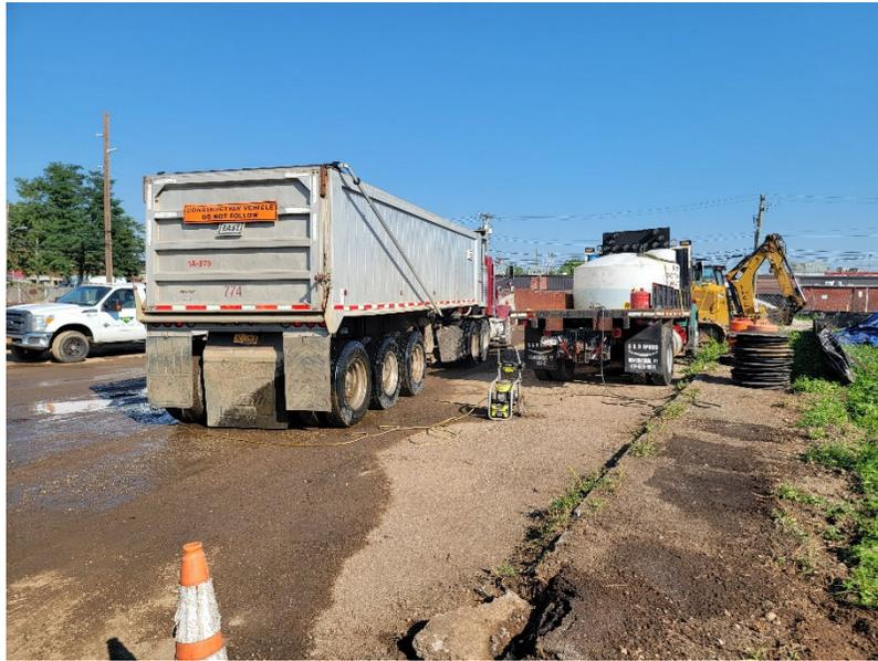
**Photo 1:** Looking north, Pratt uses power washer and truck pads to clean trucks post loading for dust mitigation and sediment track out control.
