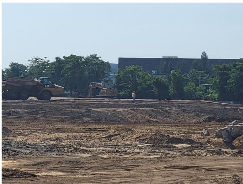
**Photo 2:** Looking south, Pratt continues excavation to subgrade for future parking lot area, Langan onsite to perform SWPPP and compaction testing.
