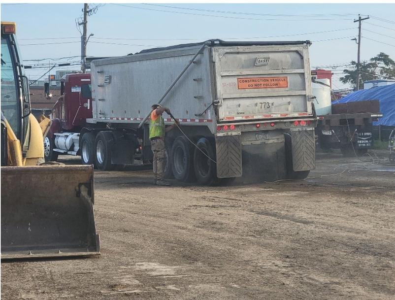
**Photo 4:** Looking north, Pratt uses power washer and truck pads to clean trucks post loading for dust mitigation and sediment track out control.
