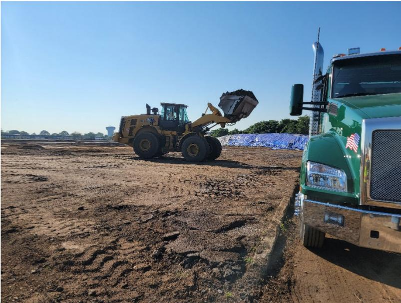
**Photo 3:** Looking south, Pratt loading stockpiled soil to truck for offsite disposal.
