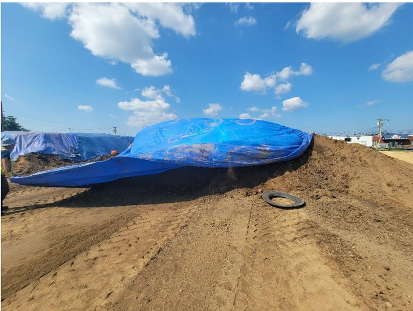
**Photo 4:** Looking north, Pratt covers topsoil stockpile at end of workday.
