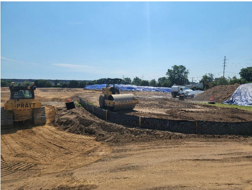
**Photo 4:** Looking south, Pratt continues regrading/drum rolling for soil compaction. Water truck in distance mitigating dust.
