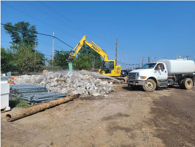
**Photo 1:** Looking northwest, Pratt begins breaking up concrete stockpiles for offsite disposal. The water truck is used for dust mitigation.
