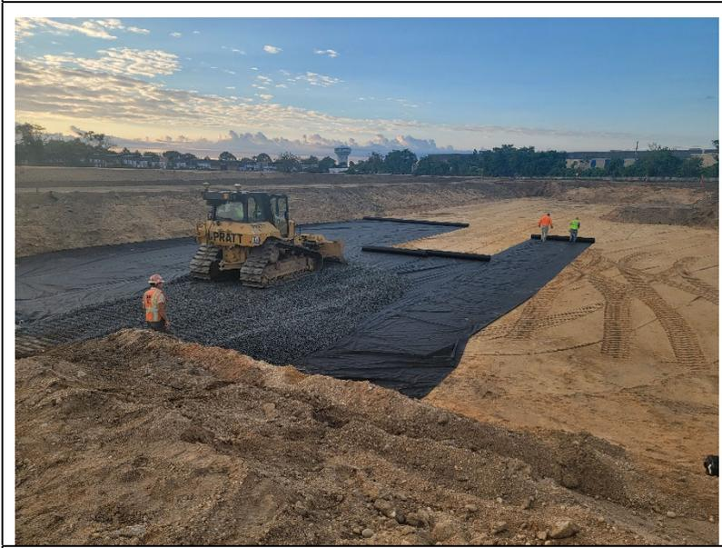
**Photo 1:** Looking south, view of Pratt laying filter fabric and grading imported #4 stone in drainage basin.
