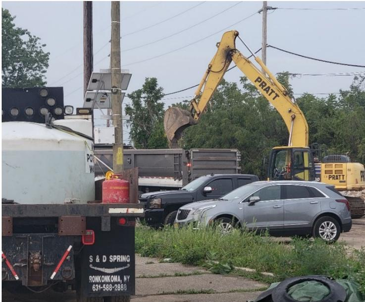
**Photo 1:** Looking southwest, Pratt loads concrete for disposal. Water truck prepared to clean truck wheels exiting the site for dust mitigation and sediment track out control.
