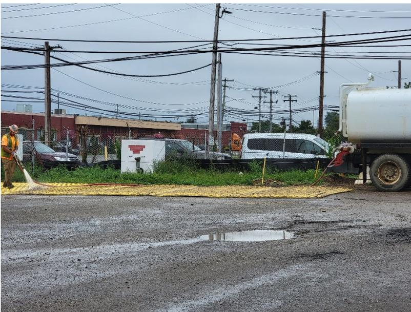
**Photo 4:** Looking north, Pratt uses power washer to clean truck pads for dust mitigation and sediment track out control.
