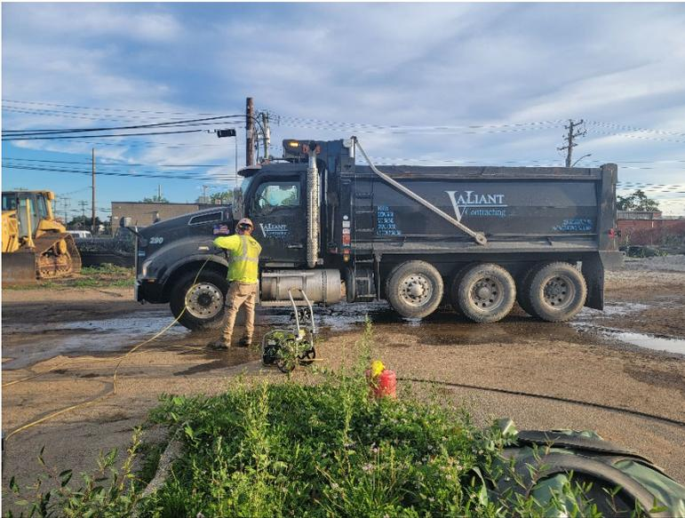
**Photo 3:** Looking north, Pratt cleans truck wheels exiting the site prior to tracking pads for dust mitigation and sediment track out control.
