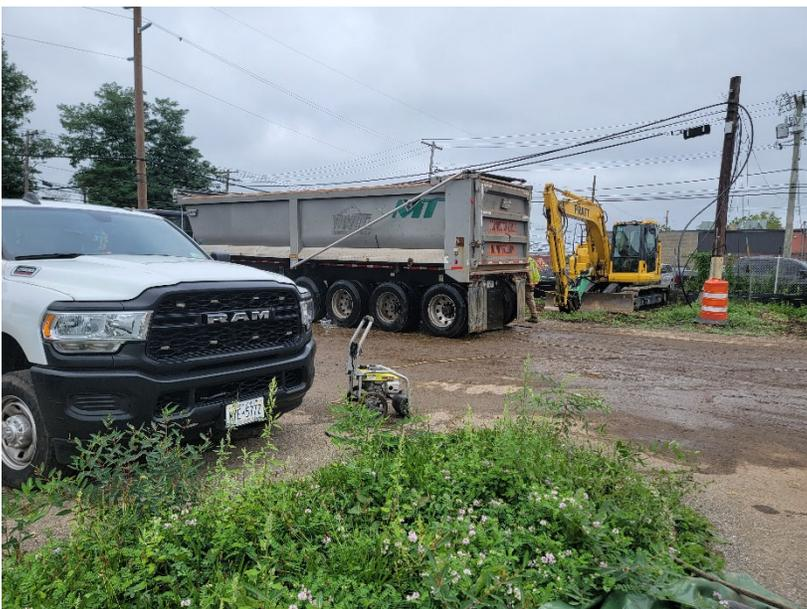
**Photo 4:** Looking north, Pratt uses power washer to clean trucks exiting site for dust mitigation and sediment track out control.
