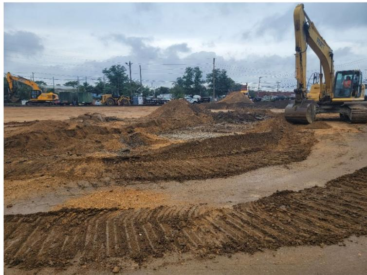
**Photo 4:** Looking west, Pratt continues excavating to subgrade for future asphalt parking area.
