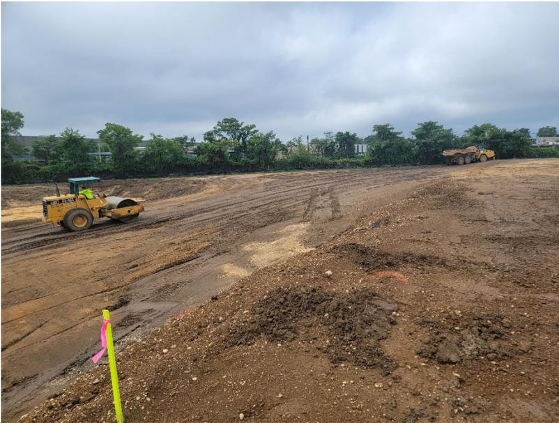
**Photo 3:** Looking southwest, Pratt continues regrading and compaction work on southern end of site.
