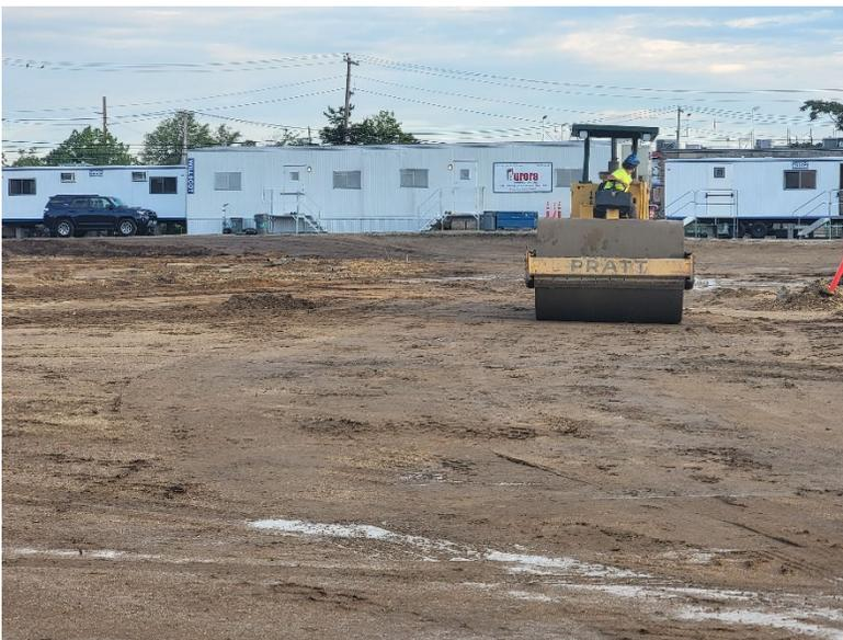
**Photo 4:** Looking north, Pratt continues compaction work in subgrade proposed asphalt parking area.
