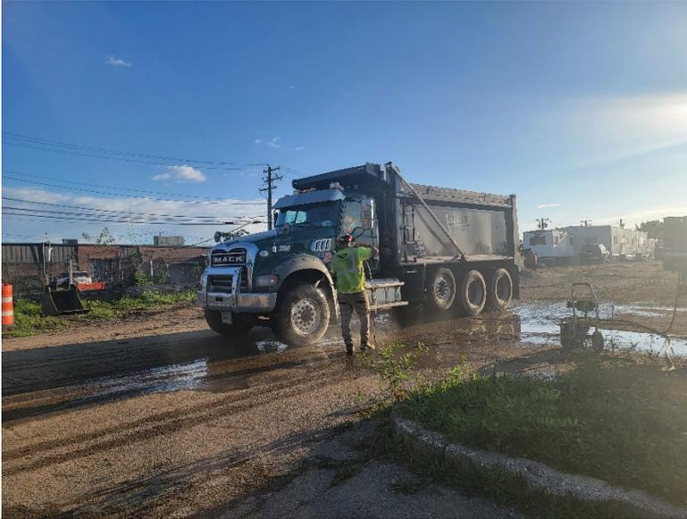
**Photo 3:** Looking northeast, Pratt cleans truck wheels exiting the site prior to tracking pads for dust mitigation and sediment track out control.
