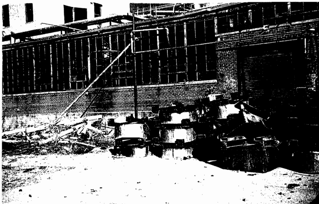
AOC 5 Transfer Station in rear of Plant 1
