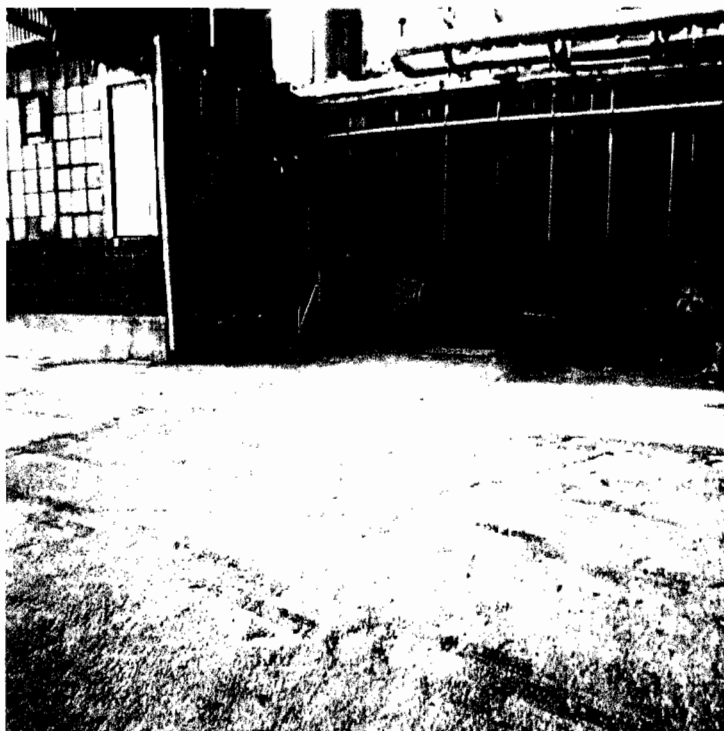
AOC 10 UST closed and AOC 11 Boiler Condensate Run-off
