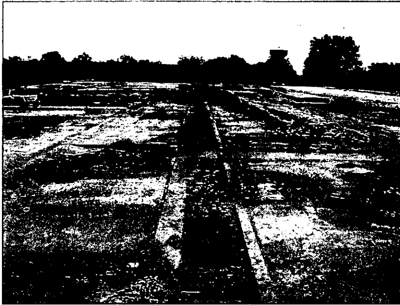
View of the trench in Plant 1 foundation.
