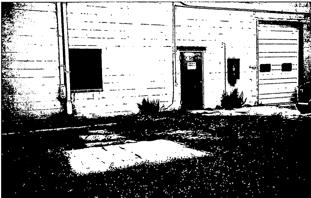
Photo of the closed laboratory storage area.
