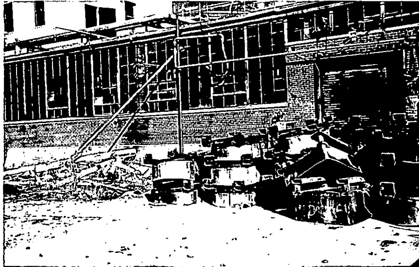
A portion of the transfer station and piping behind Plant No. 1.
