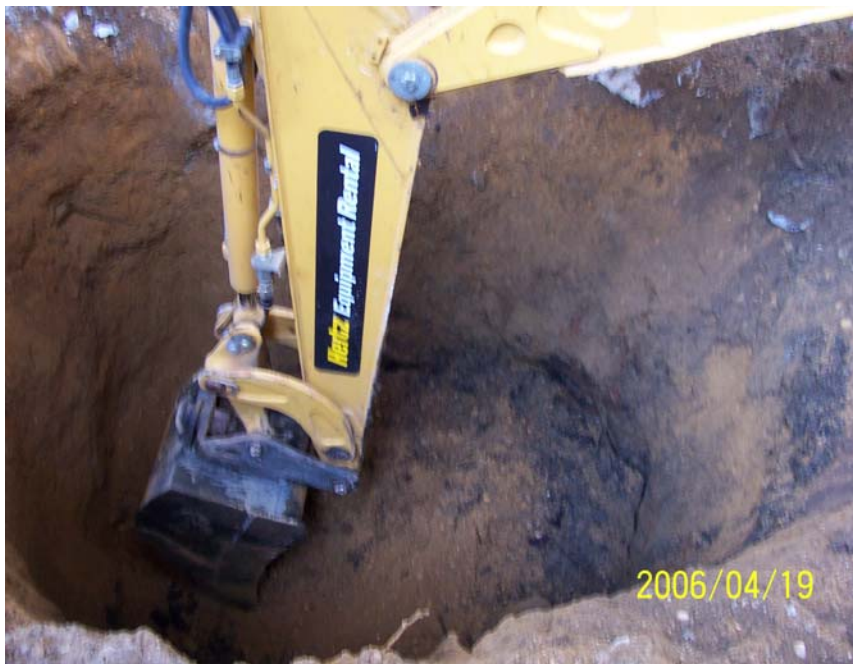
Photograph 5 - View of SF-03, interpreted as a storm water catch basin; SF-03 was a 32-inch diameter cinder block and brick-walled basin, ~10 feet deep with an open bottom and covered by a 34-inch square steel plate. The basin widened with depth and contained two terra cotta inlet/outlet pipes located approximately two feet bgs.
