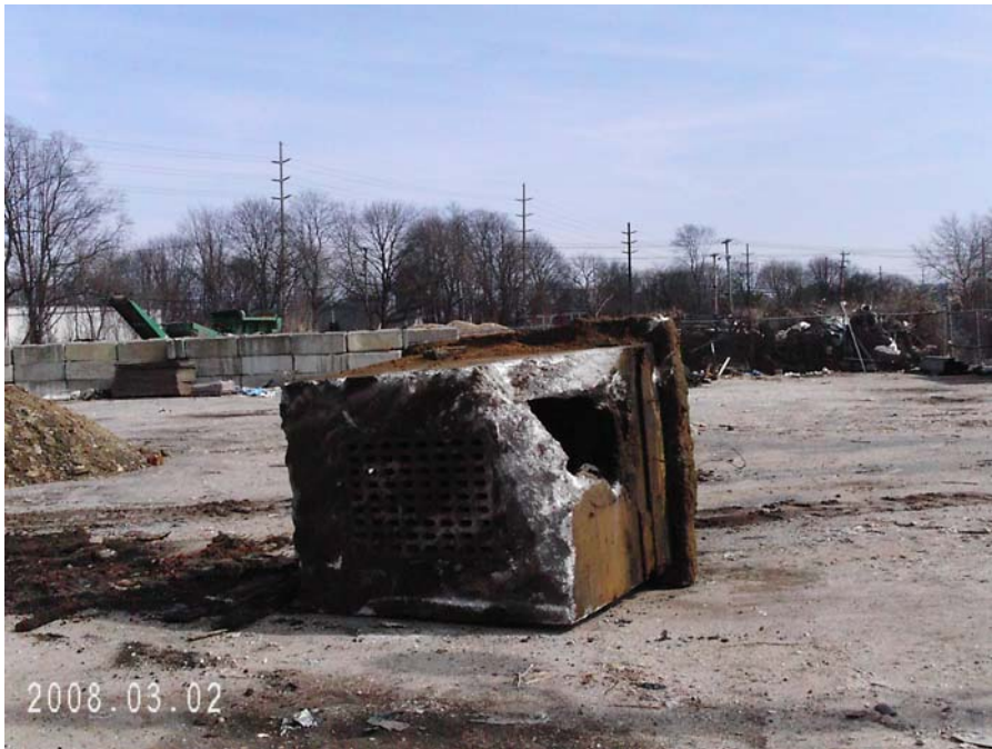
Photograph 80 – UK-45, interpreted as a stormwater catch basin, was located south of Building U in asphalt pavement. View is to northeast.
