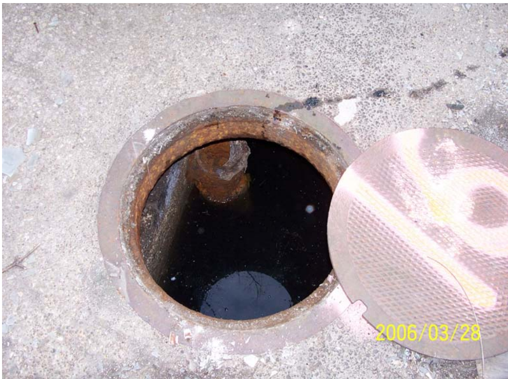
Photograph 19 - SF-16 and SF-17, interpreted as former storm or sanitary sewer access sumps, were 2-foot diameter steel manholes that led into a 15.5-foot long by 13.5-foot wide by 7.5-foot deep concrete vault. SF-16 manhole is shown above.
