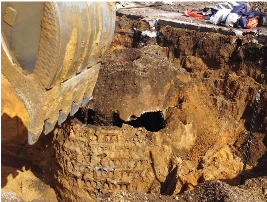
Photograph 87 – view of UK-56 (middle feature of the eastern Leaching Chamber Field) prior to removal of the feature.
