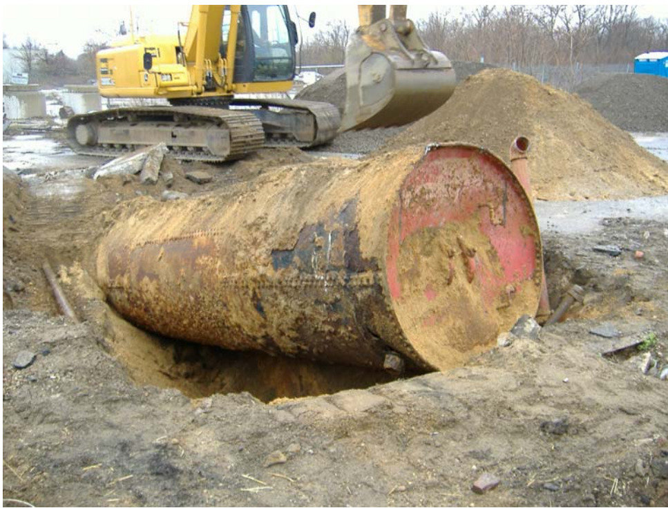
Photograph 35 – The SF-41 steel UST appeared to be used for containerizing water. Piping from SF-41 was traced to the water well located in the SF-39/SF-40 well vault.
