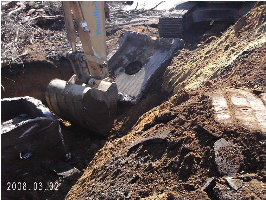
Photograph 91 – view of concrete lid being removed from UK-59. A portion of UK-59, interpreted as a stormwater drain cleanout box, can be seen on the left side of the photo.
