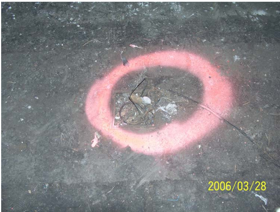
Photograph 23 – SF-19, interpreted as slab-mounted electrical junction boxes, consisted of 21 metal boxes. View above of metal-plate covered box is typical of the majority of boxes.
