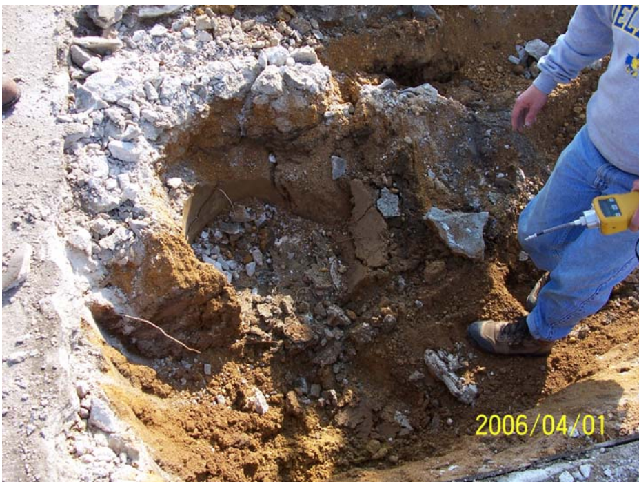
Photograph 40 – No stained soil was observed in the SF-43 excavation.
