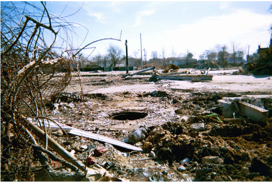
Photograph 78 - UK-44, interpreted as a stormwater catch basin, was located at the northeastern corner of Building U. Piping from UK-44 ran to SF-01, SF-08 and UK-45. View is to the south.
