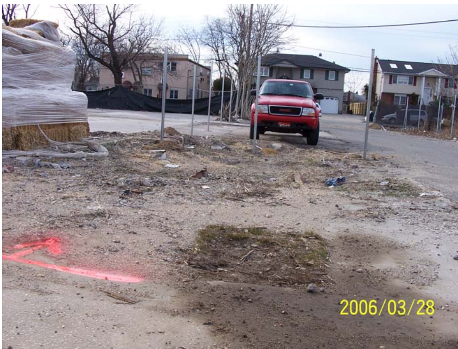
Photograph 34 – View of SF-41 prior to excavation (looking south).
