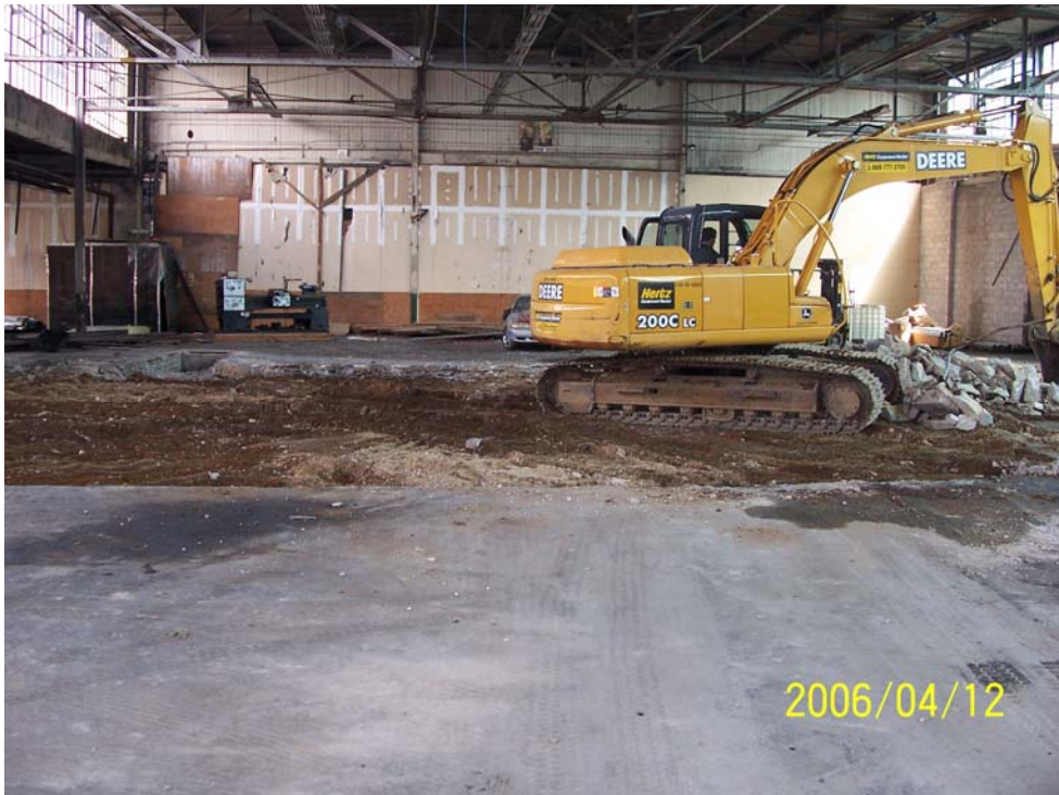
Photograph 24 – View of SF-19 excavation area for 21 electrical junction boxes.
