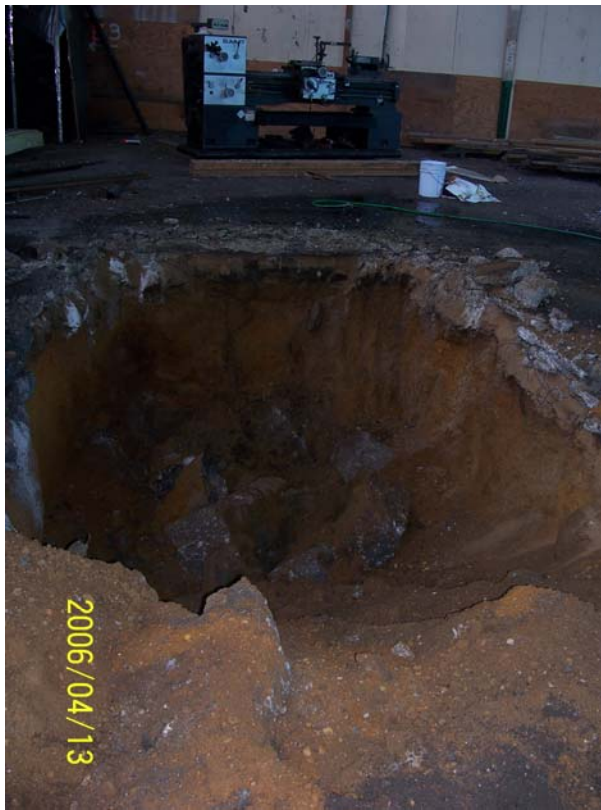
Photograph 55 – View of SF-49 excavation looking to the east.
