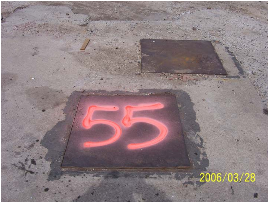
Photograph 57 – SF-55, interpreted as a former production water well vault and steel UST used for containing the well water. The vault was 10-feet by 10-feet by 8-feet deep with two 32-inch square steel manhole covers. View is to the north.
