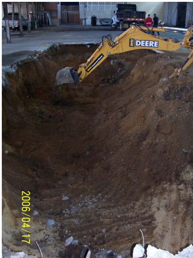
Photograph 27 – SF-20 excavation area looking east.
