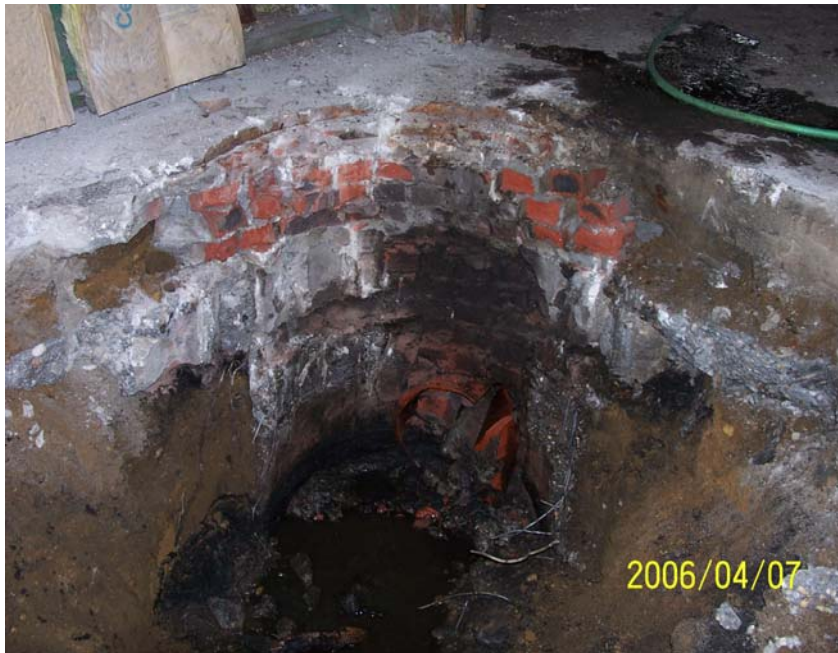
Photograph 12 – View of partially excavated brick and concrete-walled basin at SF-07.
