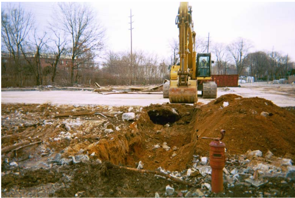
Photograph 82 – view of UK-46 (looking east), discovered while excavating test trenches across SF-48 excavation to verify that no UST was present at SF-48.
