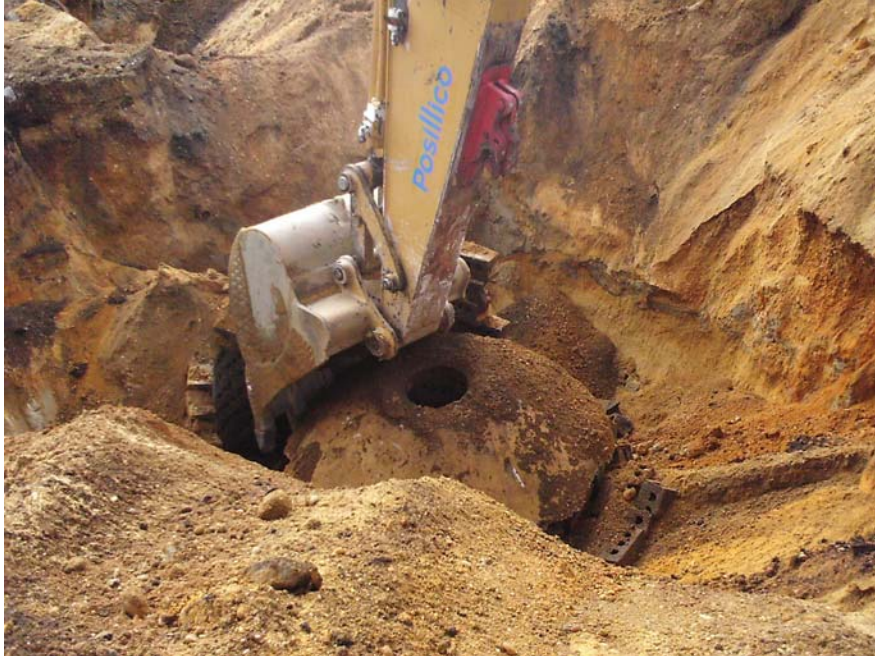
Photograph 84 – view of domed concrete lid of UK-54 being removed during excavation.
