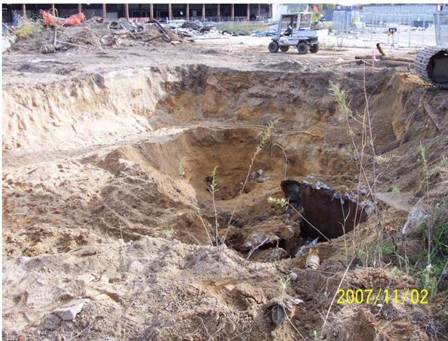
Photograph 75 – UK-37 excavation nearing completion (looking southeast).
