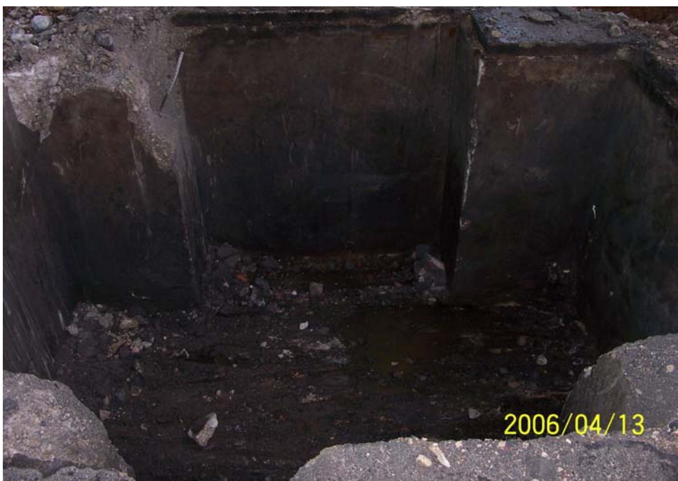
Photograph 26 – View of one of the three vaults excavated from SF-20 after removal of demolition debris.
