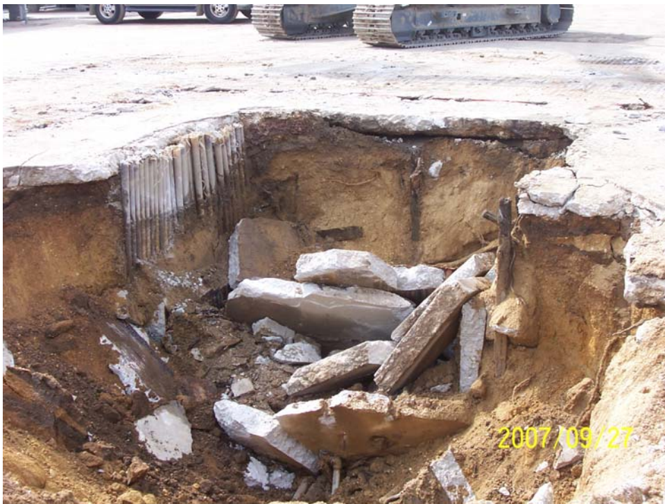
Photograph 71 – view of UK-33/UST-13A excavation.
