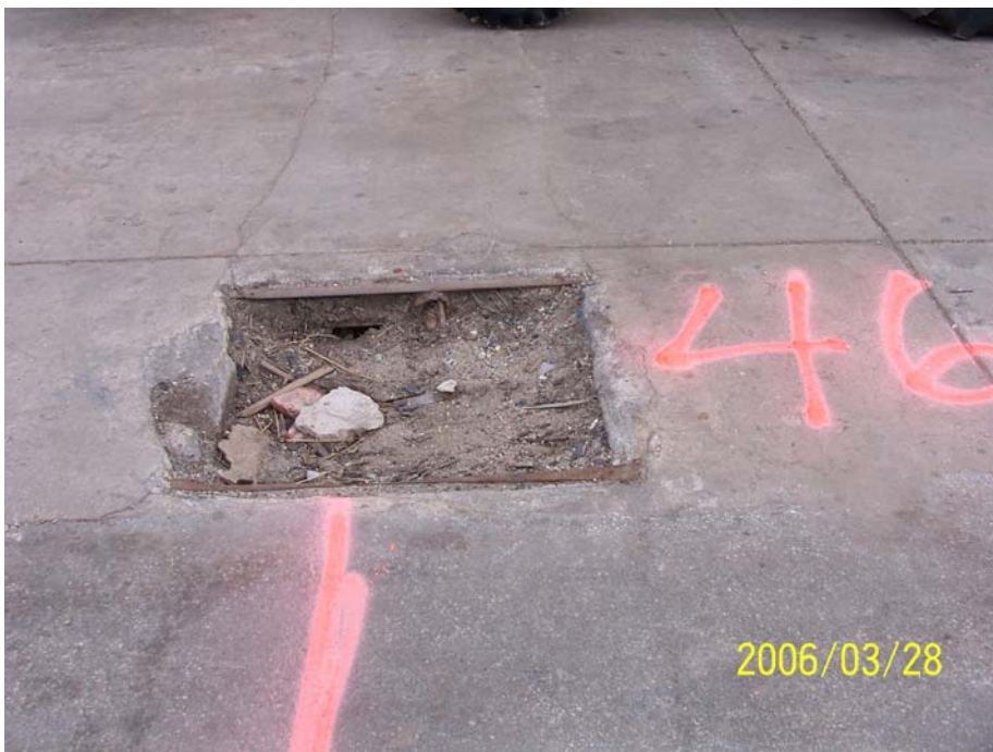
Photograph 45 – SF-46, interpreted as former lavatory floor drains and water supply piping, was comprised of two vaults located approximately 23 feet apart.
