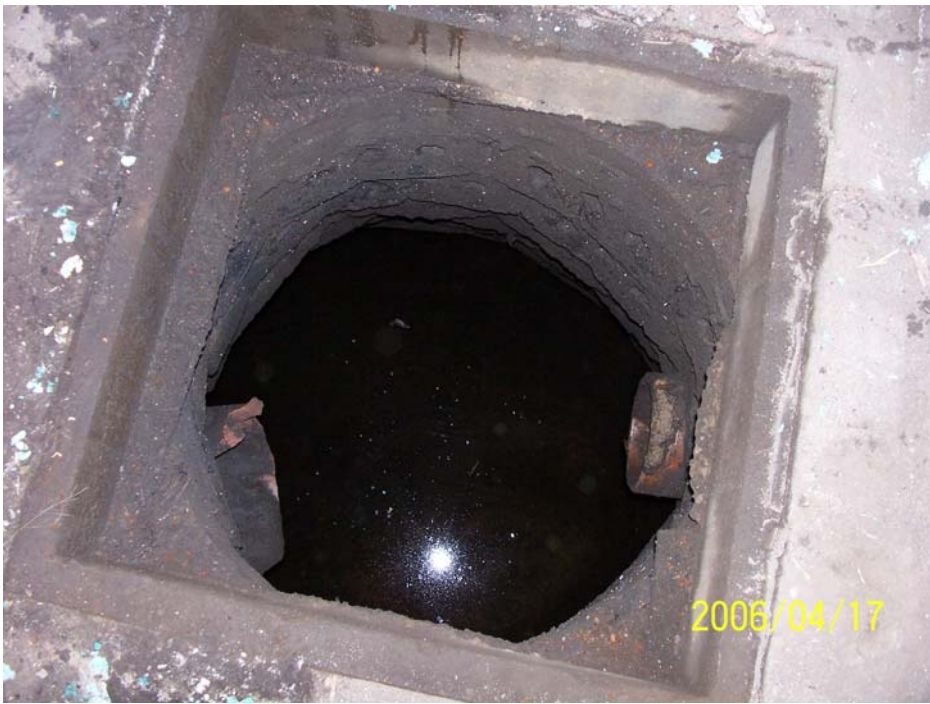
Photograph 5 - View of SF-03, interpreted as a storm water catch basin; SF-03 was a 32-inch diameter cinder block and brick-walled basin, ~10 feet deep with an open bottom and covered by a 34-inch square steel plate. The basin widened with depth and contained two terra cotta inlet/outlet pipes located approximately two feet bgs.
