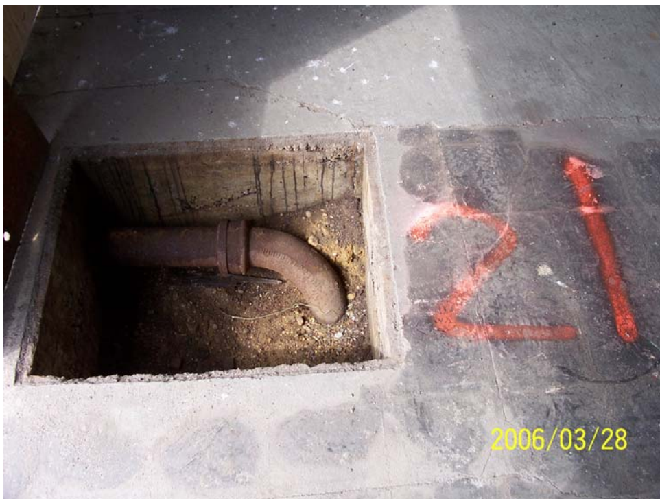
Photograph 29 – SF-21 contained horizontal east-west trending 4-inch diameter cast iron piping.
