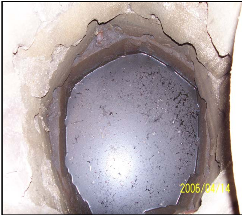
Photograph 9 – SF-05, interpreted as a storm water catch basin, was an ~24-inch diameter vertical brick basin with a solid concrete bottom that was covered by a 23-inch diameter steel manhole cover. SF-05 was connected to SF-06 by a terra cotta inlet/outlet pipe that entered the basin at a depth of 2 feet bgs.
