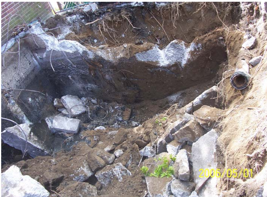
Photograph 19 - SF-16 and SF-17, interpreted as former storm or sanitary sewer access sumps, were 2-foot diameter steel manholes that led into a 15.5-foot long by 13.5-foot wide by 7.5-foot deep concrete vault. SF-16 manhole is shown above.
