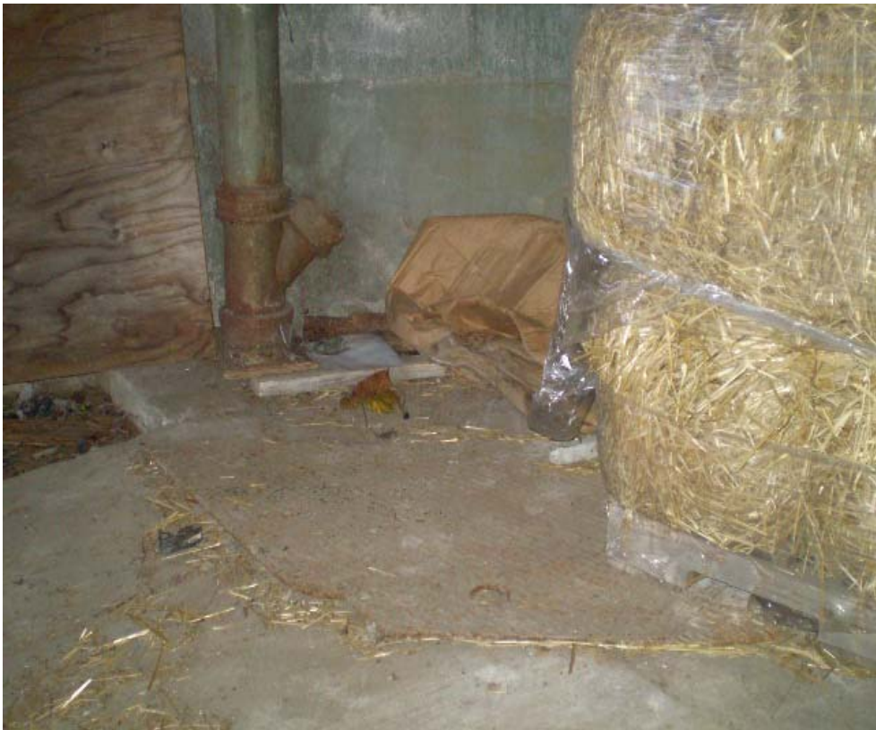
Photograph 13 – SF-08 was located near the northwestern corner of Building U. Pictured is the trapezoidal shaped steel cover. SF-08 was interpreted as a small brick and mortar catch basin, approximately 4-feet by 4-feet by 4-feet deep.. The roof drain pictured in the background discharged to SF-08. 6-inch diameter terra cotta piping entered SF-08 from the east and west.
