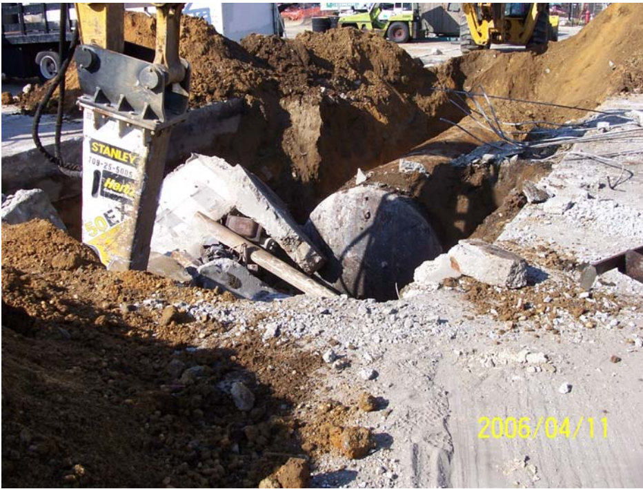
Photograph 59 – View during excavation of the vault and 6,200-gallon steel UST associated with SF-55.
