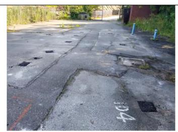
Photo 1: Soil boring surfaces restored in Area 1.
