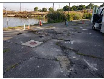
Photo 2: Soil boring surfaces restored in Area 2.
