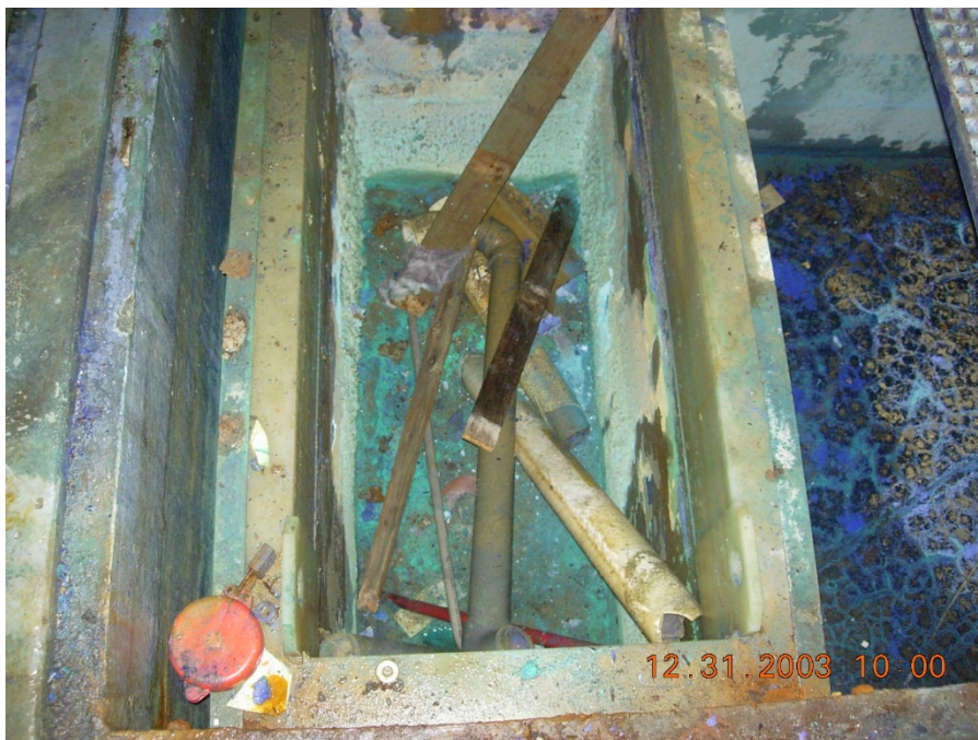
Sludge and debris in sump
