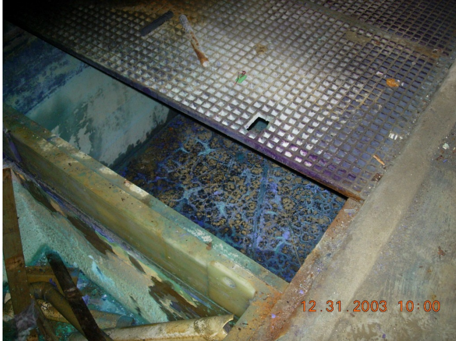
Sludge at bottom of sump
