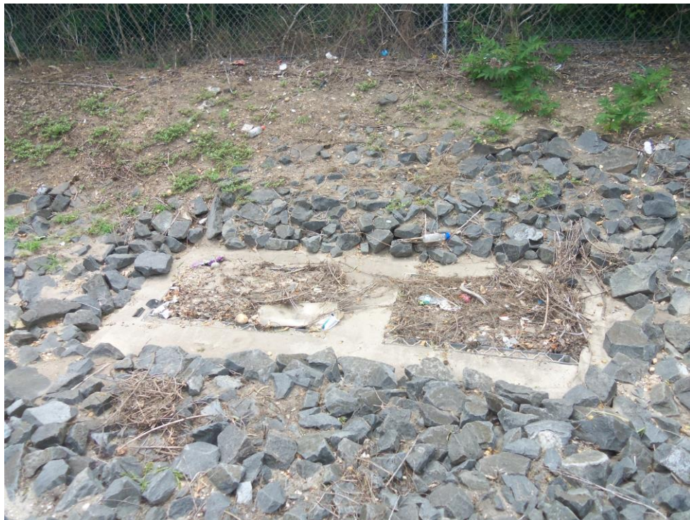
Siltation and Debris - CB#2
