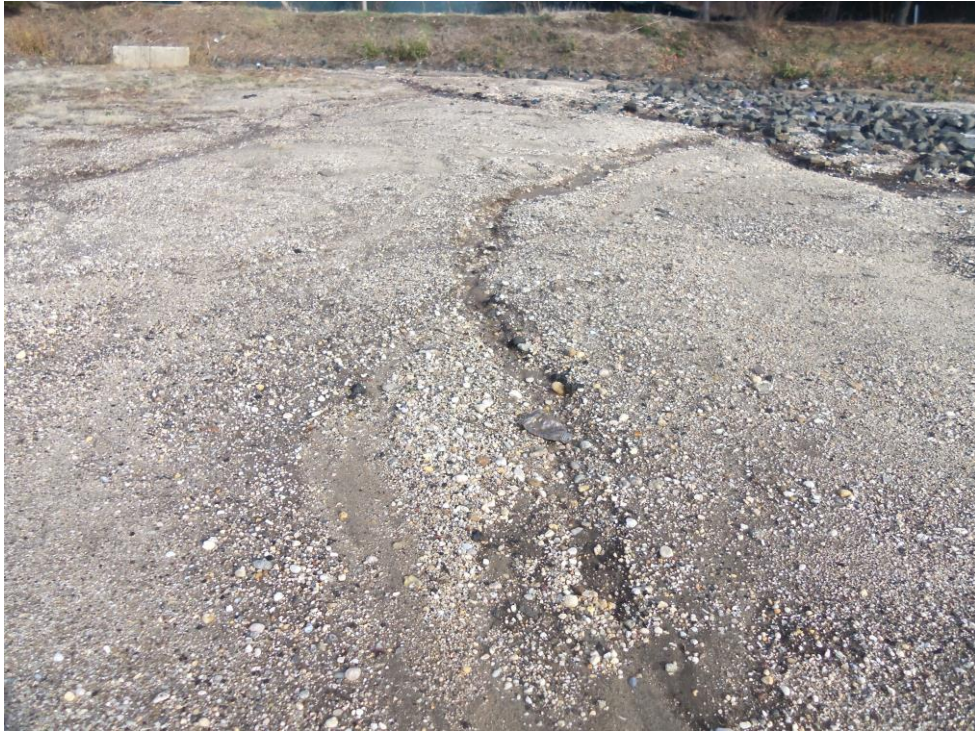
Surface Material Erosion in Area C
