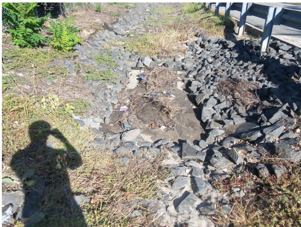
Catch basin #2 siltation and debris
