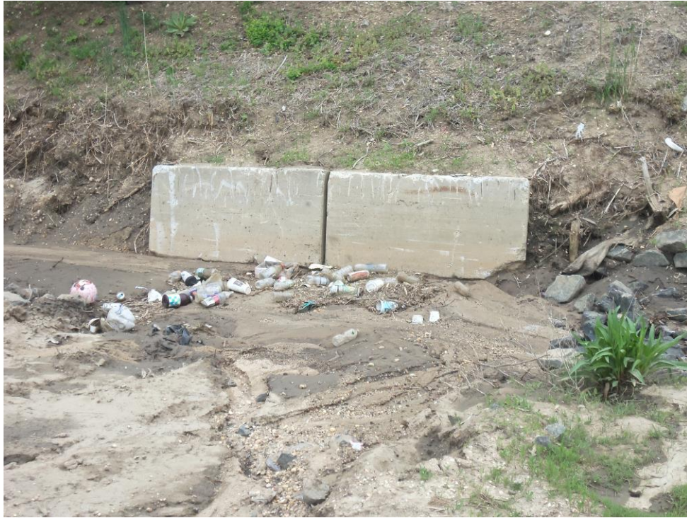
Siltation and Debris CB#5
