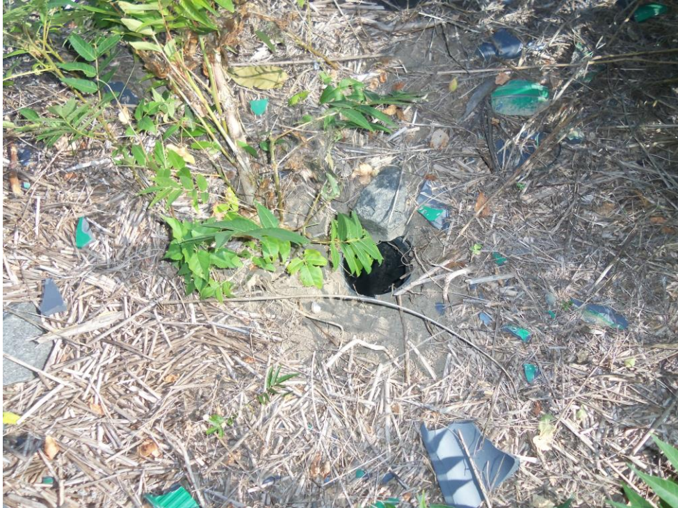
Well casing broken at grade – SW3
