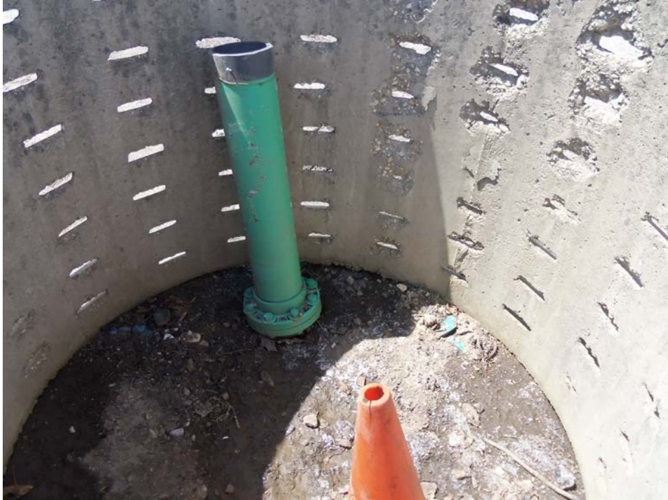
Well casing broken at/just below grade - R-8
