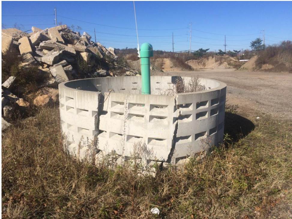
Protective Ring Damaged – R1
