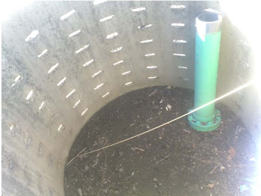
Well Casing Broken at/just below Grade- R8
