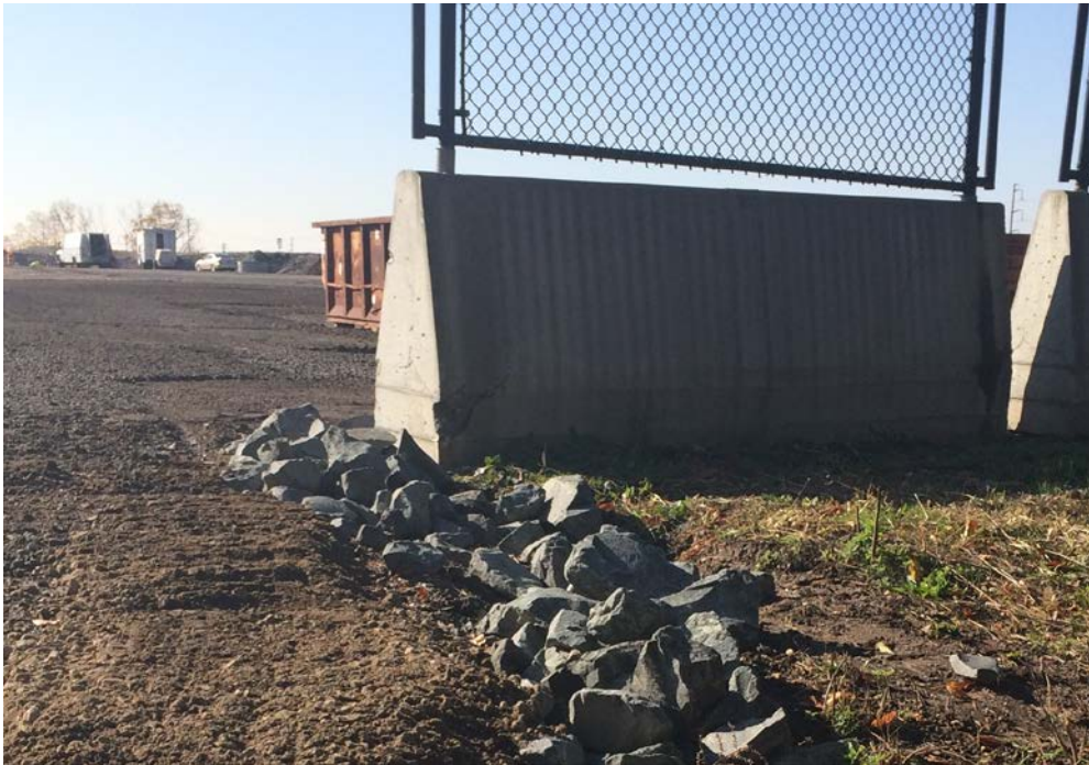
Area B Washout Repaired
