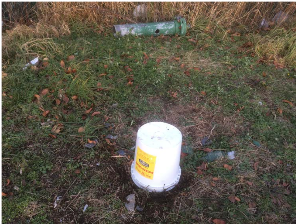
Well Casing Broken at Grade – NE16
