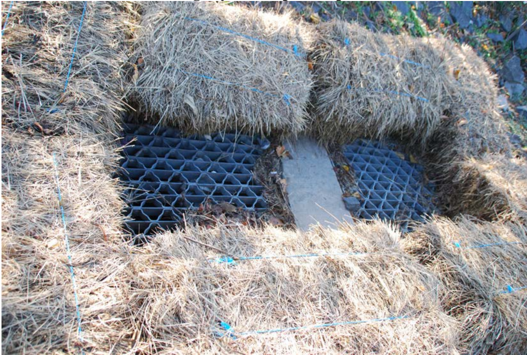
Catch Basin #2 Hay Bales Installed
