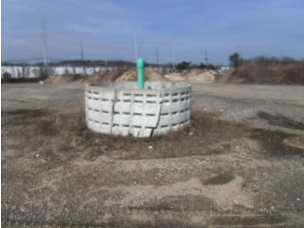
Protective Ring Damaged – R1
