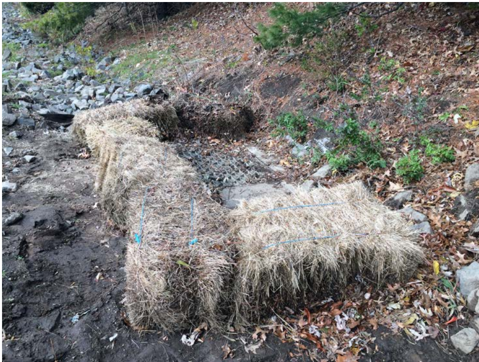
Catch Basin #5 Hay Bales Installed
