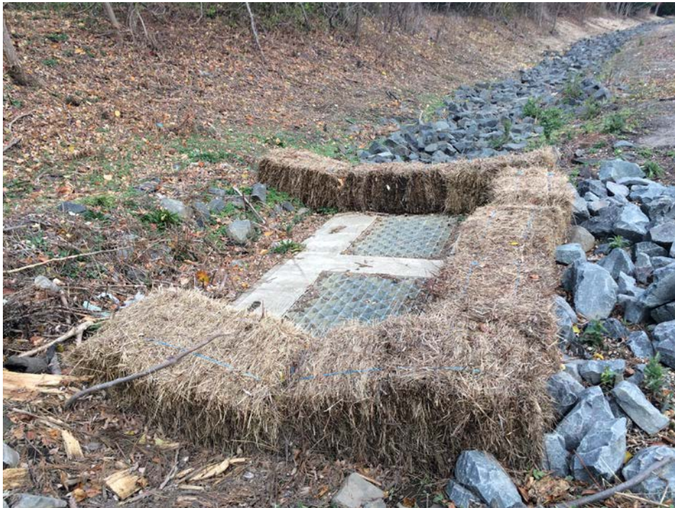
Catch Basin #3 Hay Bales Installed
