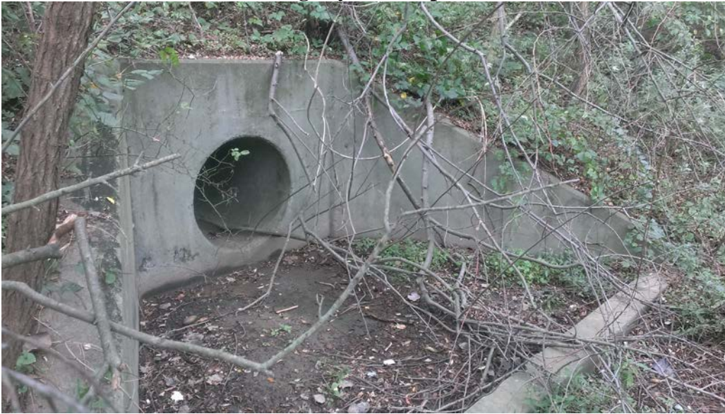
Minor Siltation/Vegetative growth – RB #358 (HW #4)
