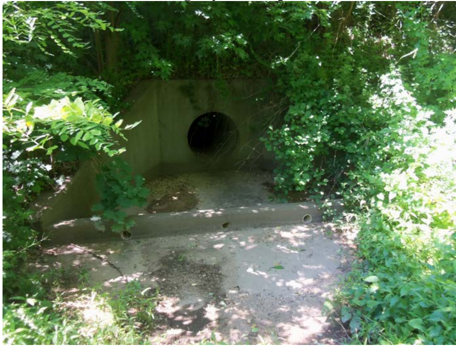
Minor Siltation/ Vegetative Growth –RB #284 (HW #2)
