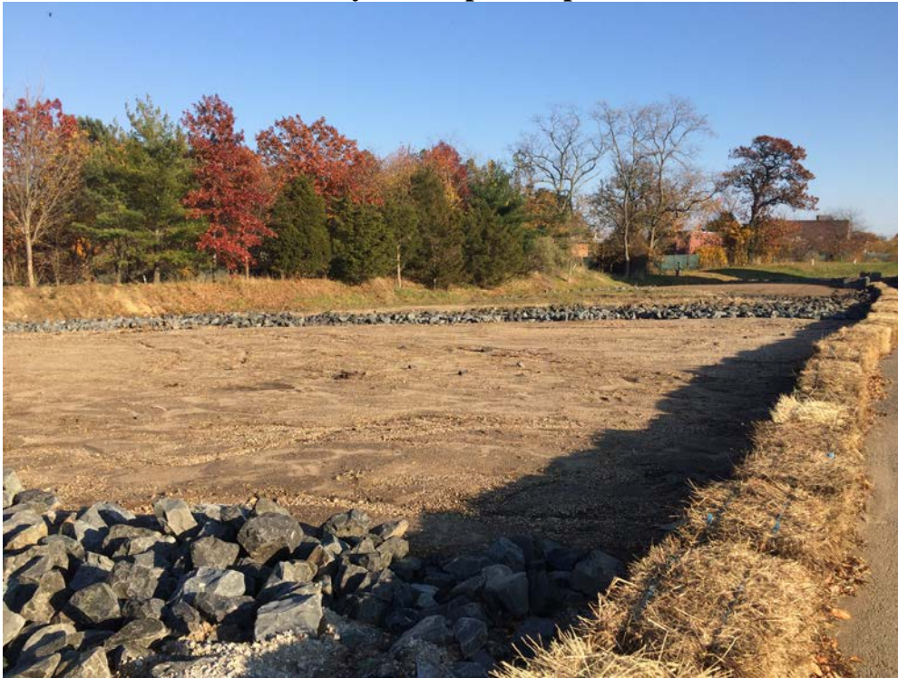
Area C Perimeter Regraded, Hay Bales and Rip Rap Installed
