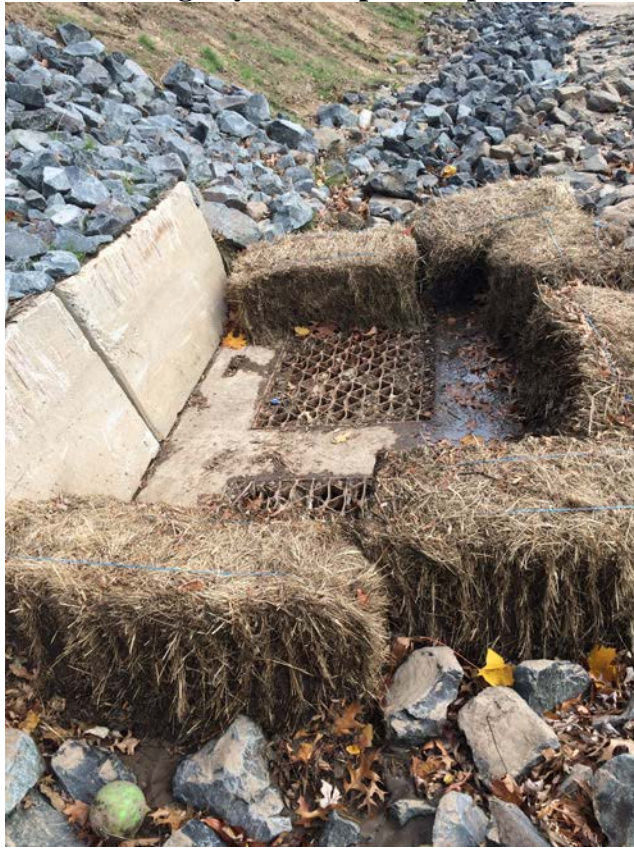
Catch Basin #4 Hay Bales Installed
