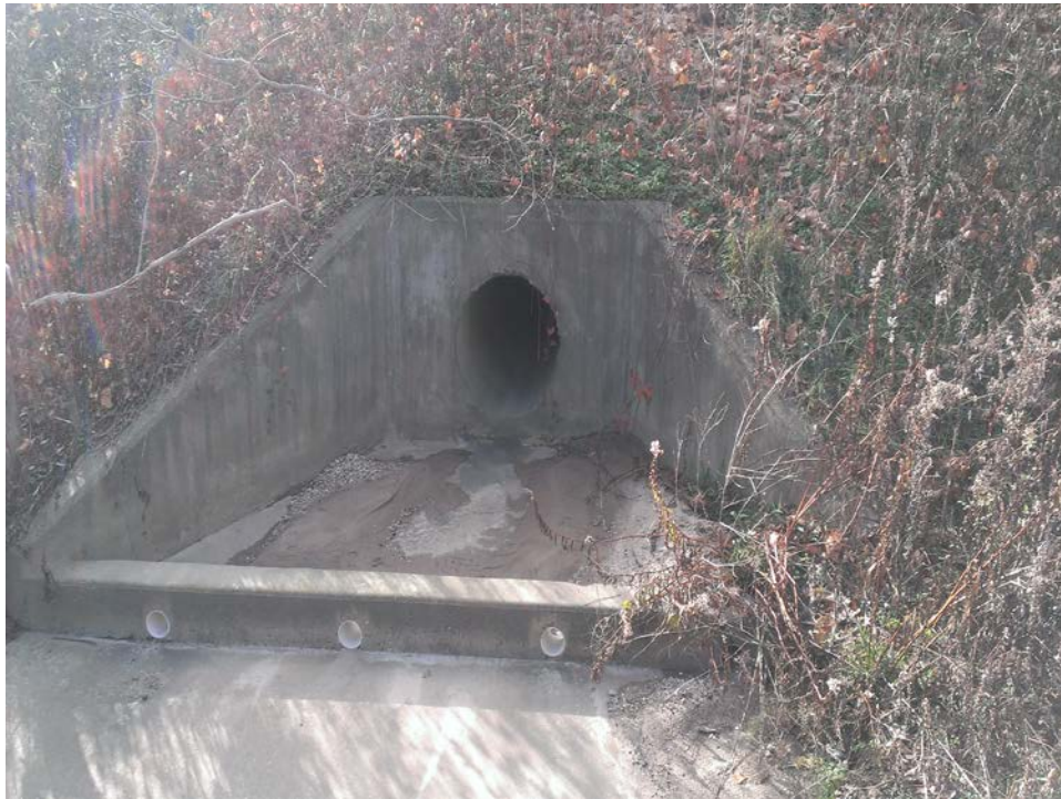
Minor Siltation/Vegetative growth – RB #284 (HW #3)
