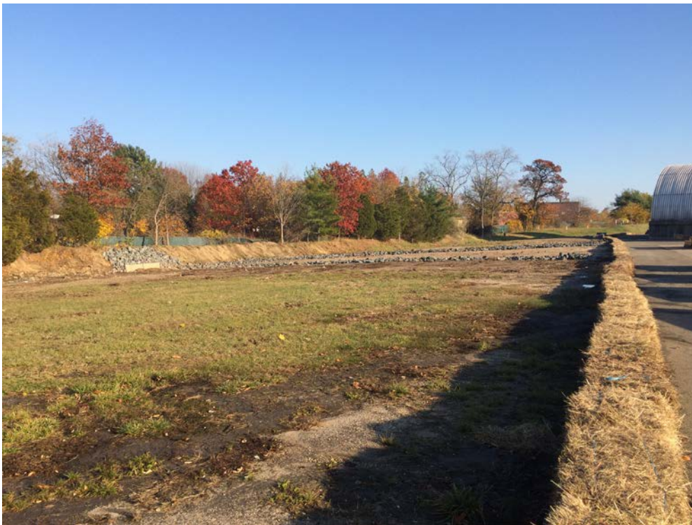
Area C Perimeter, Hay Bales and Rip Rap Installed
