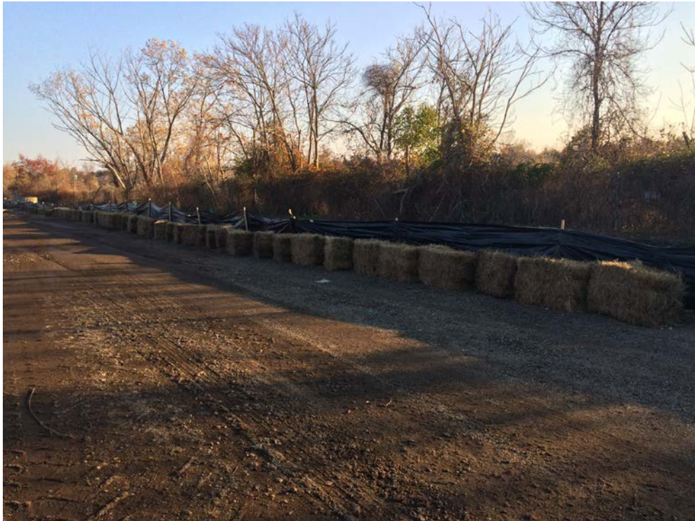
Hay Bales and Silt Fence along Ditch Section #6
