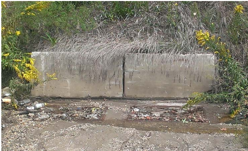
Siltation/Debris – Catch Basin #5
