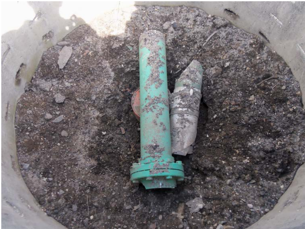
Well Casing Broken at Grade- R8
