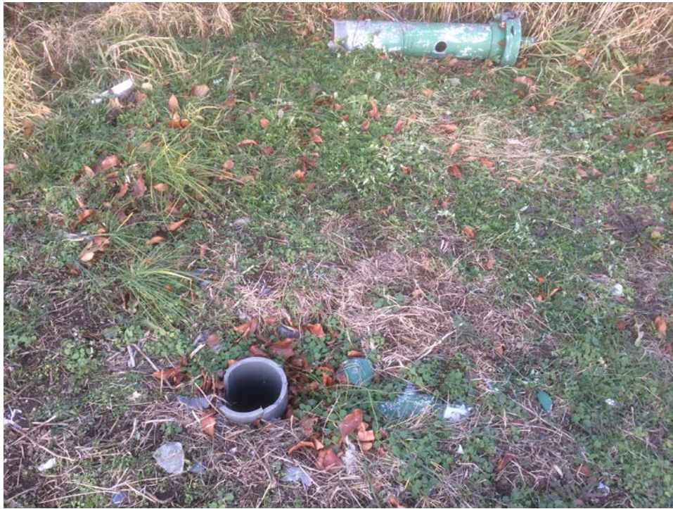
Well Casing Broken at Grade- NE16
