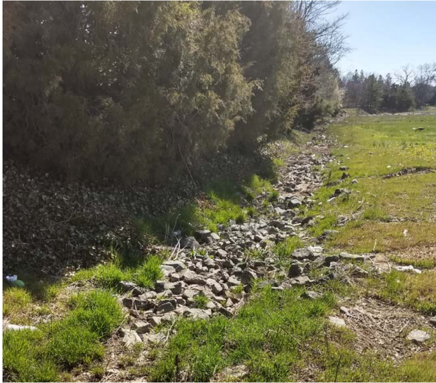
Some siltation, vegetation growth and debris – DS#3
