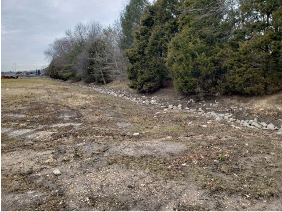
Lack of vegetation at perimeter in Area B
