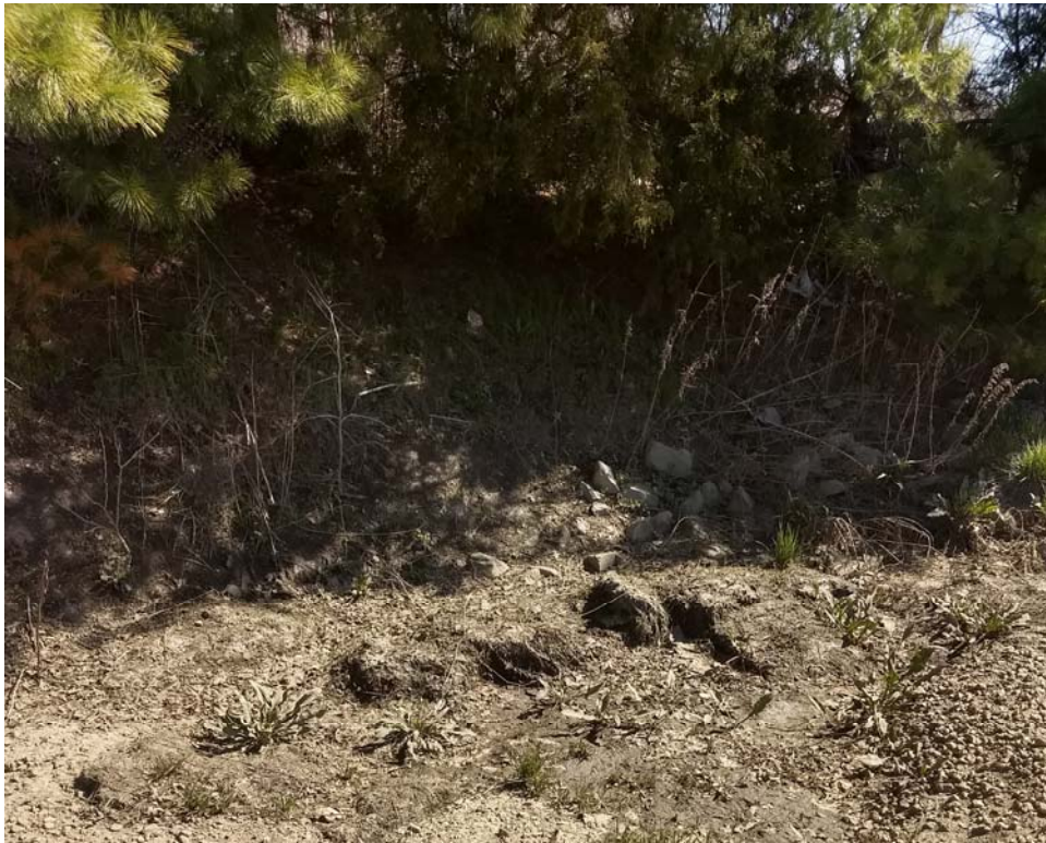
Surface erosion at perimeter in Area B
