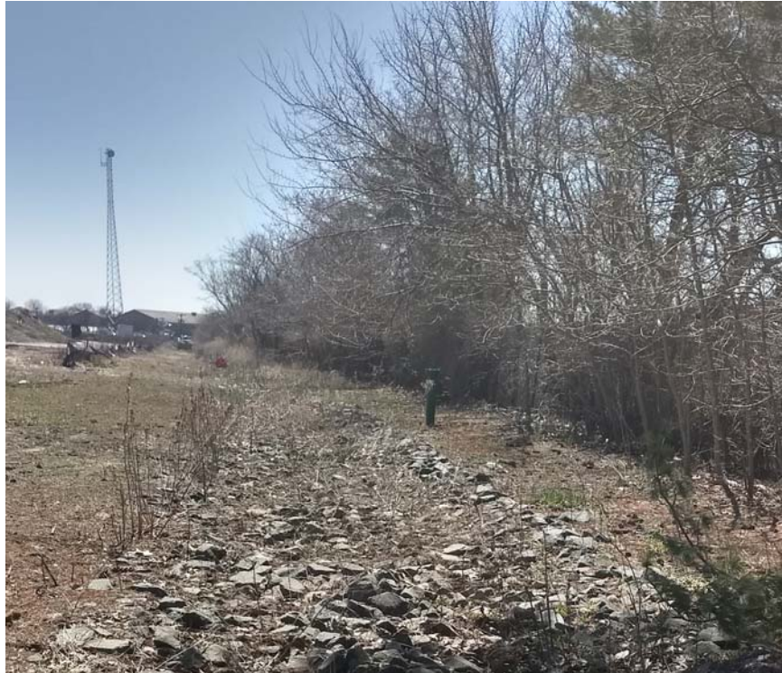
Siltation, vegetation growth and debris – DS#6
