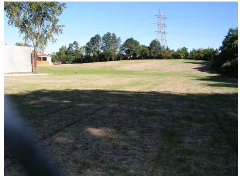
Site after debris removal 10/03/2003
