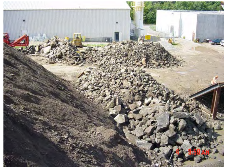
Concrete and processed fines stockpiles 8/4/2003
