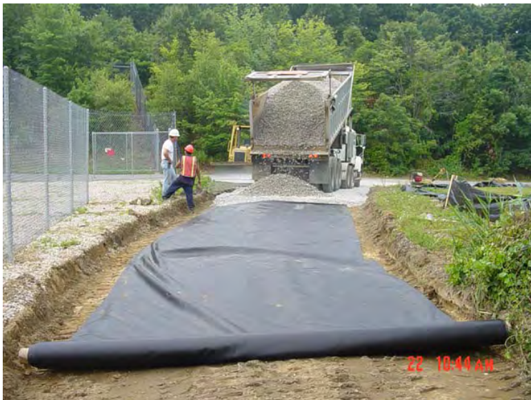
Access road construction 7/22/2003
