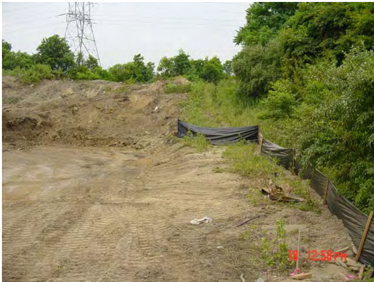
Silt fence erosion control 7/18/2003
