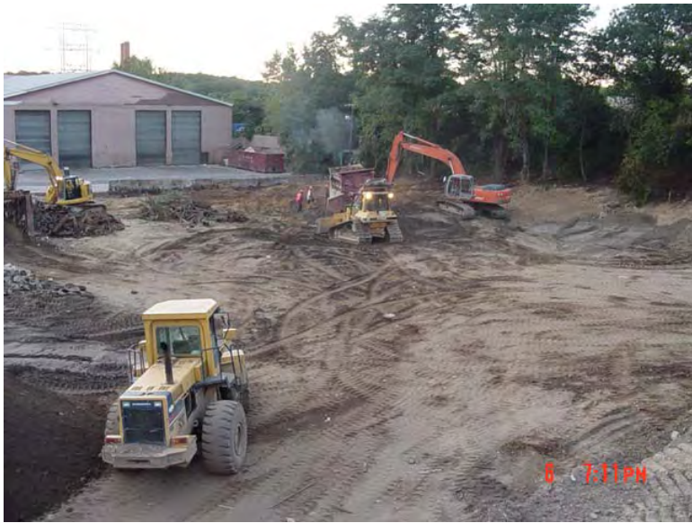
Last day of debris removal operations 9/6/2003
