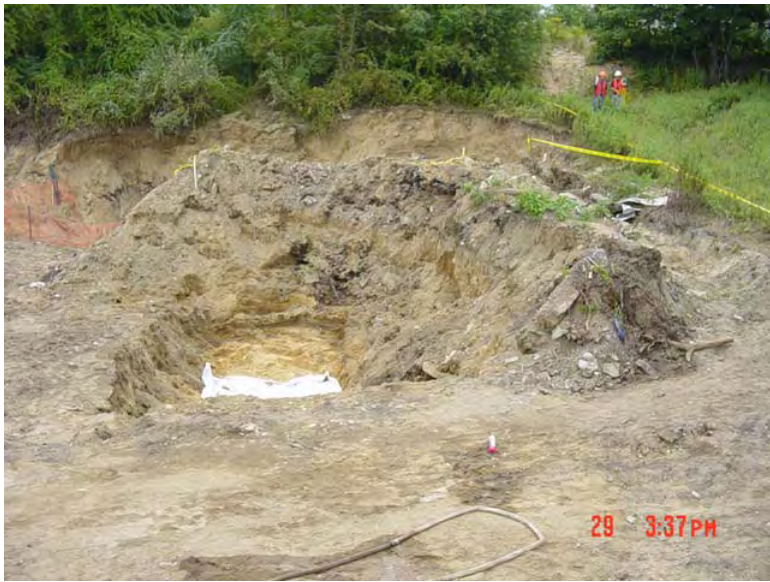
Completed Hazardous Area excavation 8/29/2003
