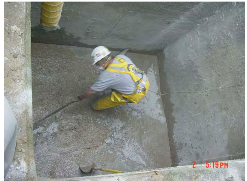
Sediment stabilization in storm water pits 9/02/2003
