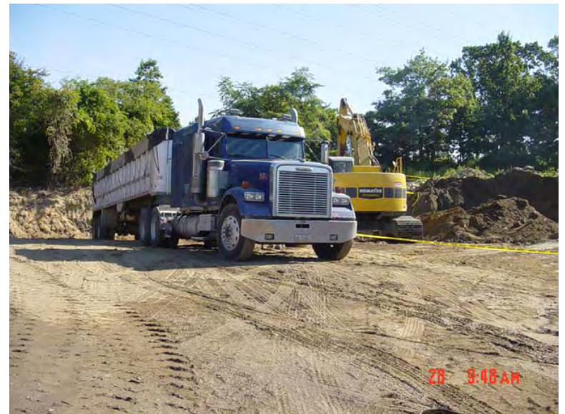
Loading hazardous materials for off-site disposal 8/28/2003
