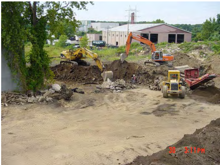
Debris removal operations 7/30/2003
