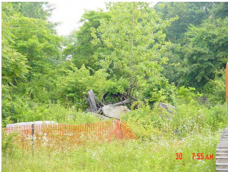
Debris area before clearing 6/30/2003
