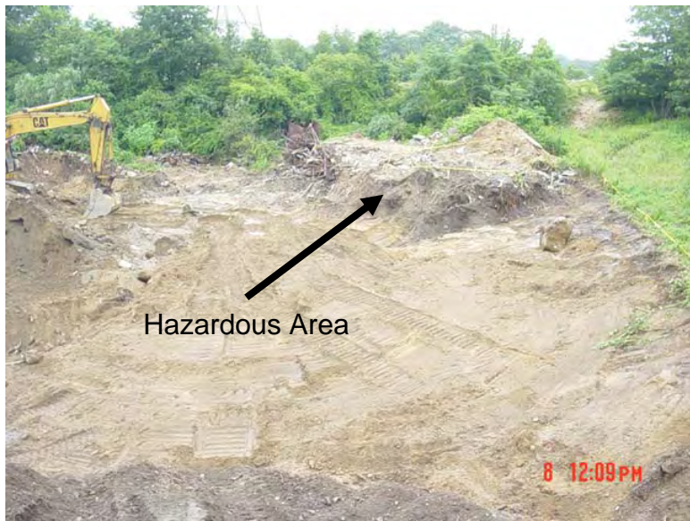
Hazardous Area before excavation 8/8/2003
