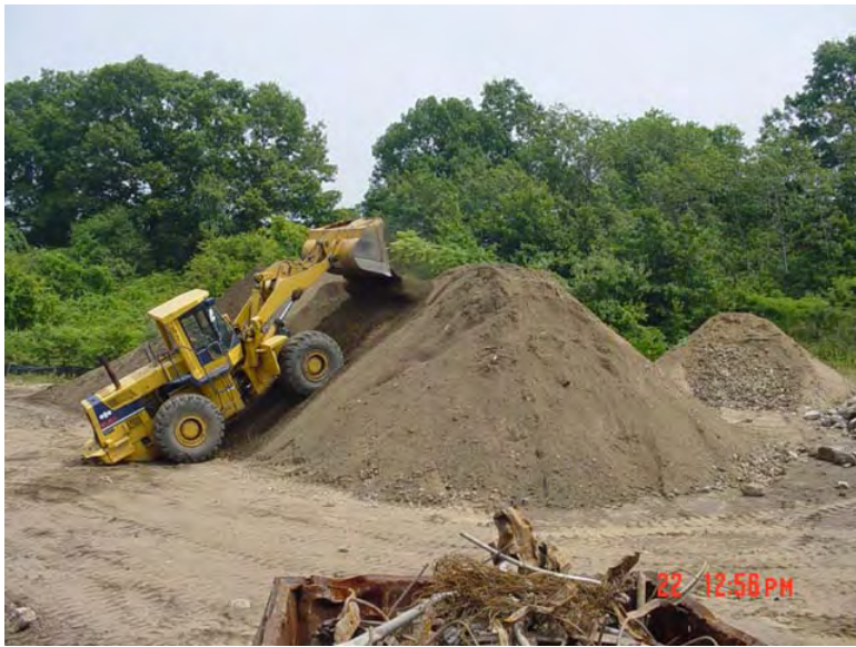
Stockpiling processed fines 7/22/2003
