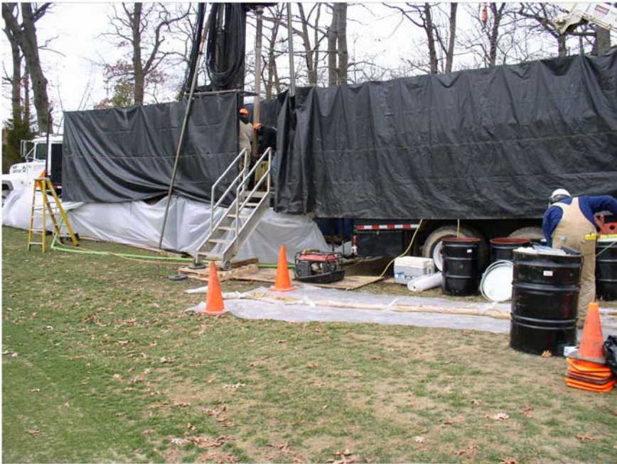
Drilling At EW-2D
