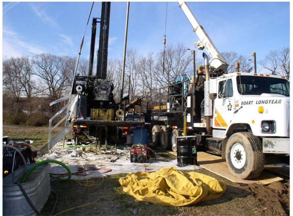
Setting up for groundwater sampling At EW-10C (side by side set-up)
