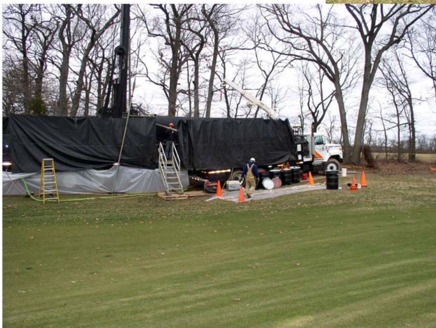
Drilling at EW-2D
