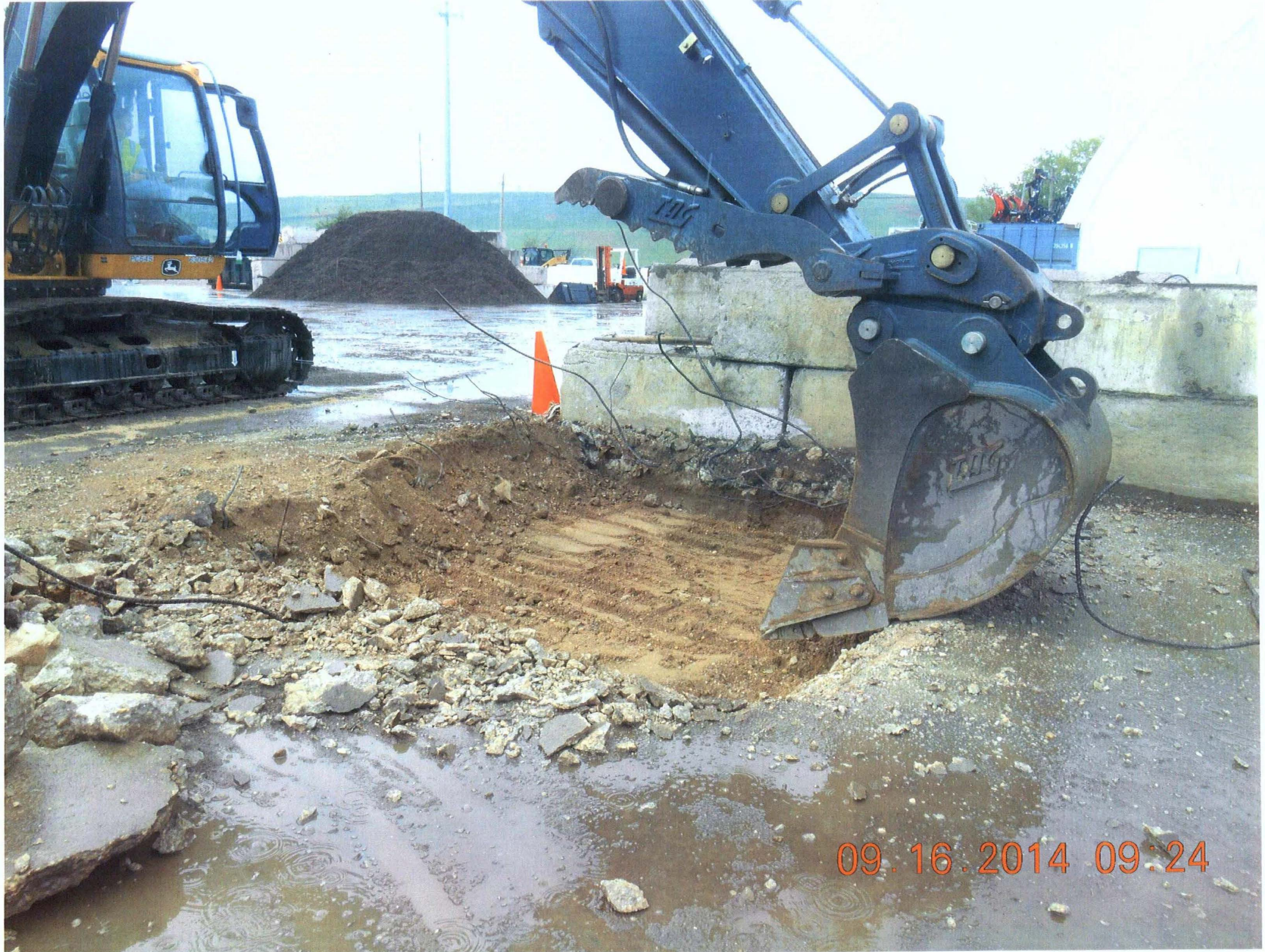
EXCAVATION AREA D
