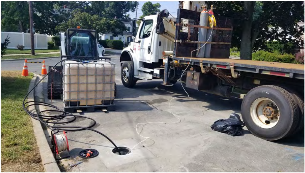
Well development of MW-CPC-37
