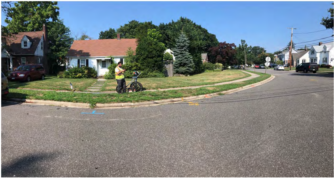
Subsurface utility mark out at MW-CPC-38
