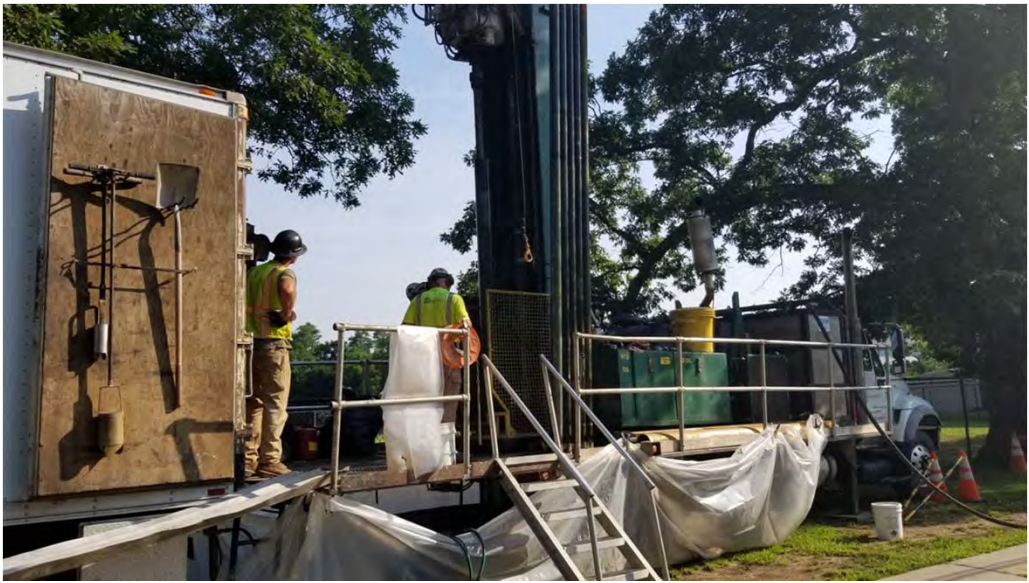
Drillers lowering sampling bailer down MW-CPC-36
