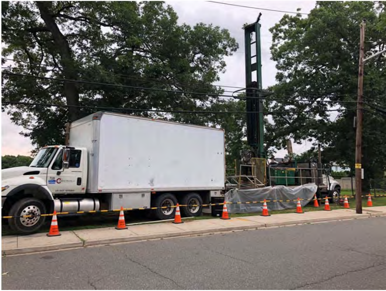
Drill rig and support truck setup on MW-CPC-36
