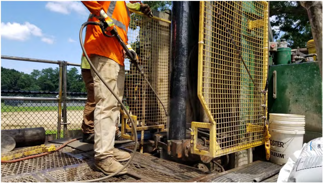
Cascade steam cleans well casing as it is removed from subsurface.
