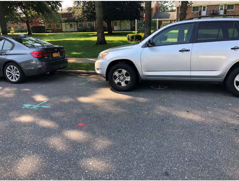
Subsurface utility mark out at MW-CPC-39
