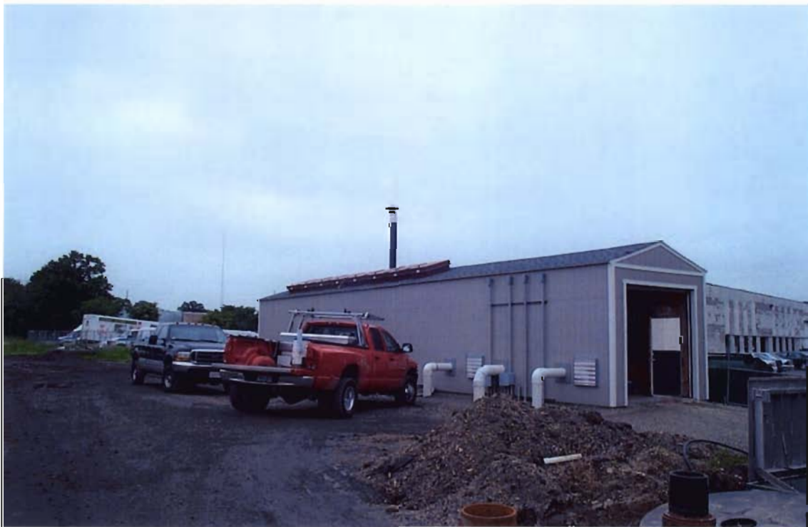
Photograph 9: Equipment building and exhaust stack.
