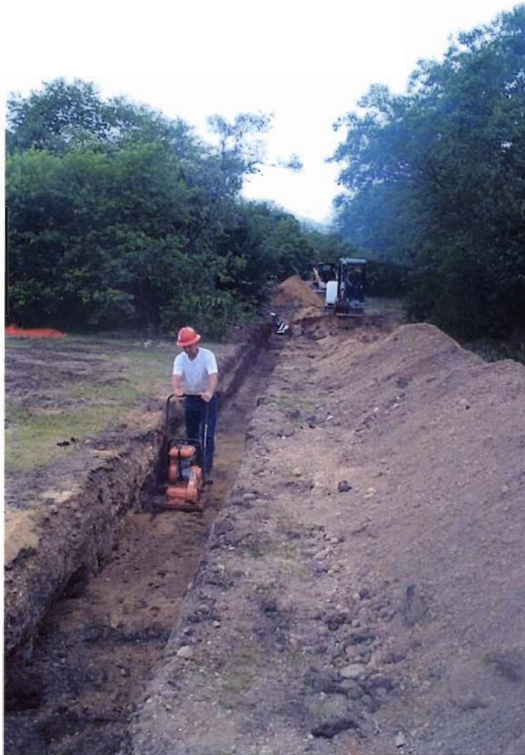
Photograph 5: Compacting backfill over piping.
