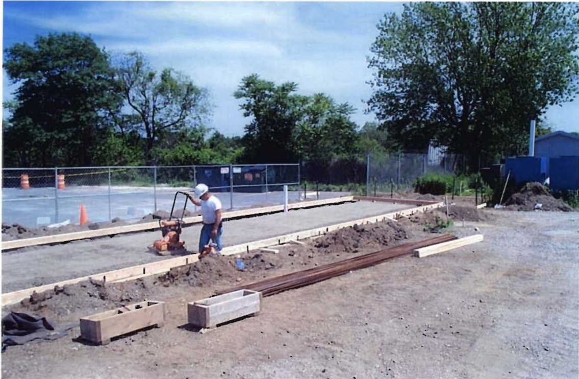
Photograph 1: Compacting subgrade for building foundation.
