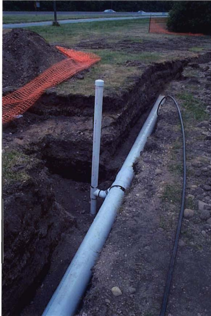
Photograph 4: Installation of condensate collection points.
