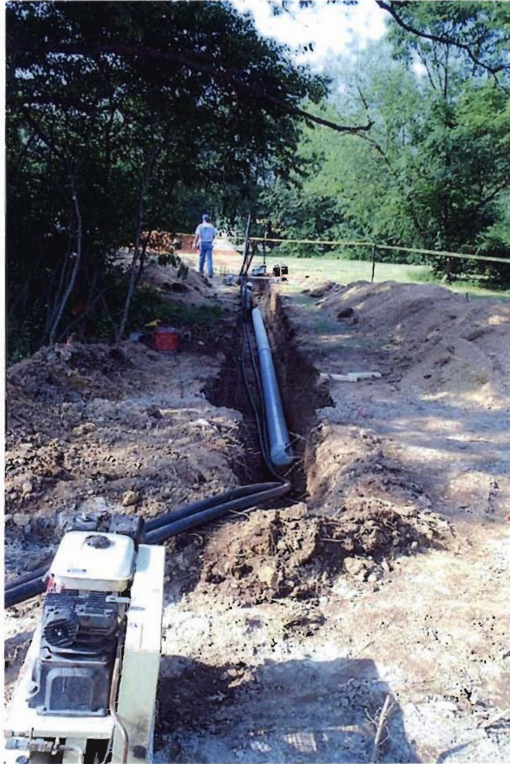
Photograph 3: Installing vapor transfer line and electrical conduits from well UVB-2.
