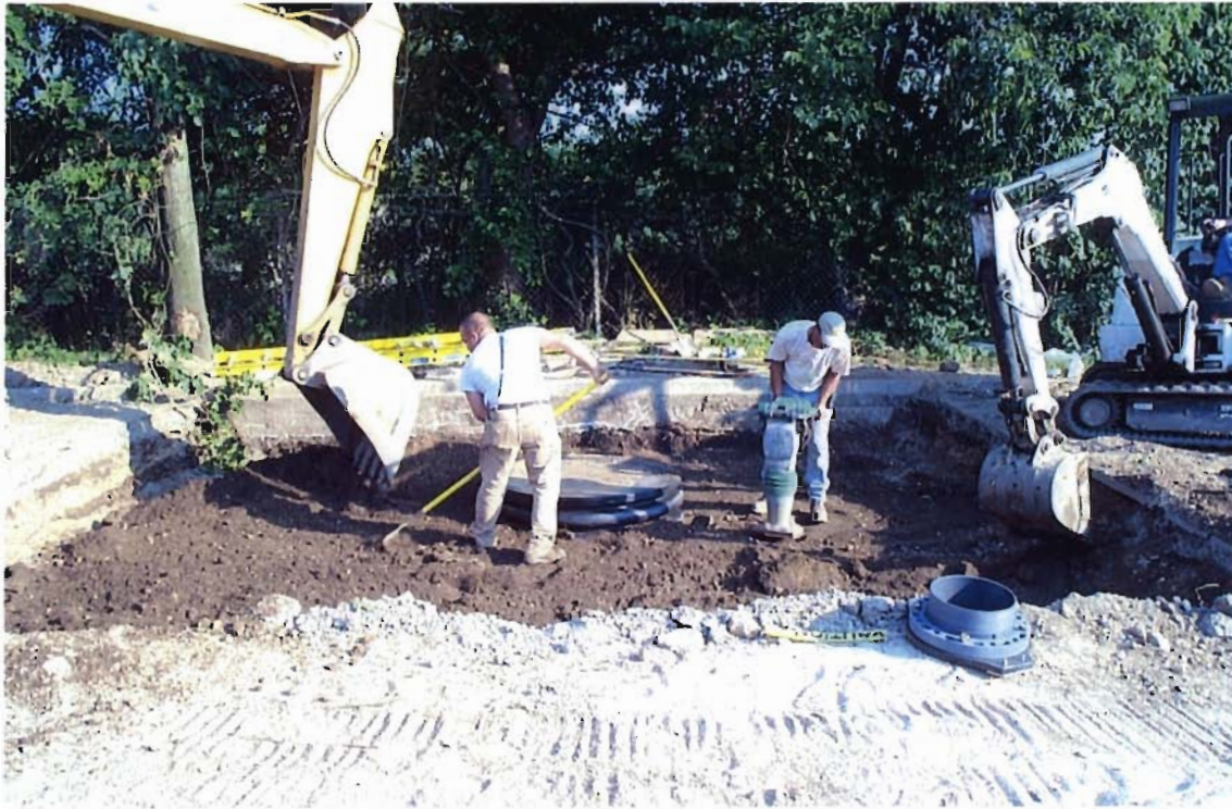
Photograph 6: Compacting fill around well UVB-3.
