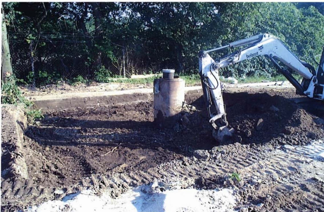
Photograph 2: Excavating around steel casing for well UVB-3
