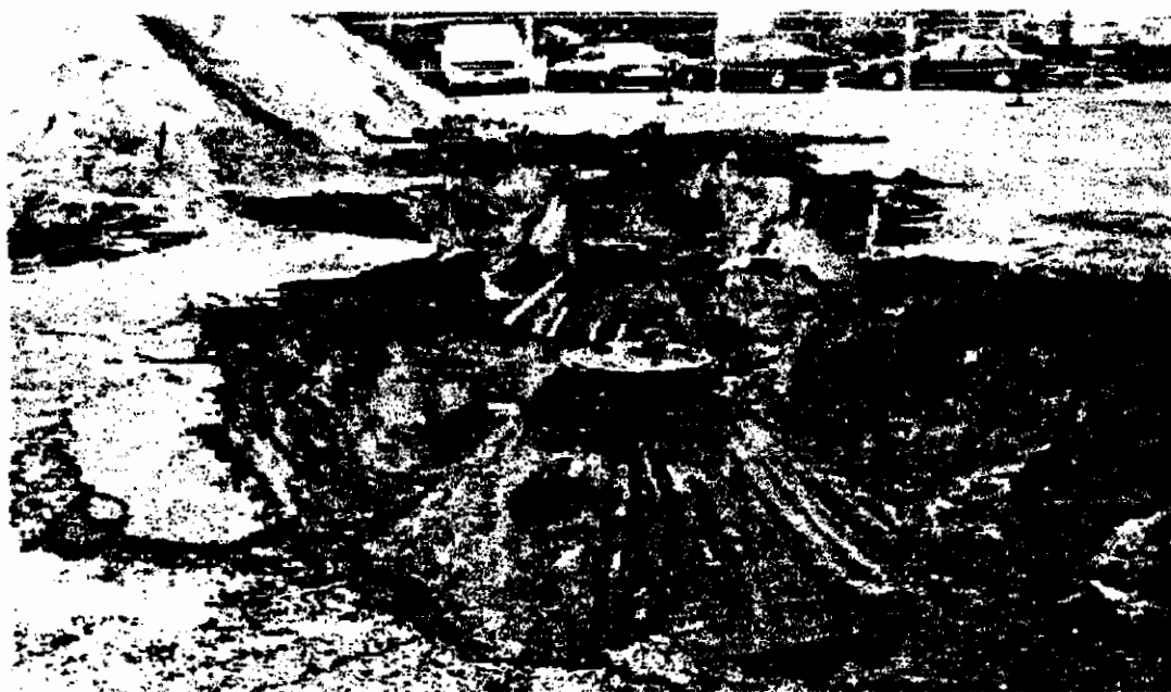
Figure 4: Exposed leaching pools during excavation
