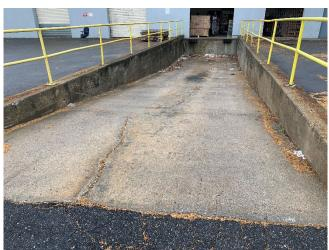
Minor cracking in asphalt cover system, facing southwest.
