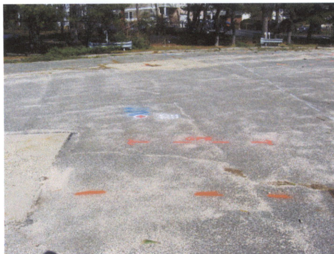
Photograph 11: View looking north toward R-SB-11.
