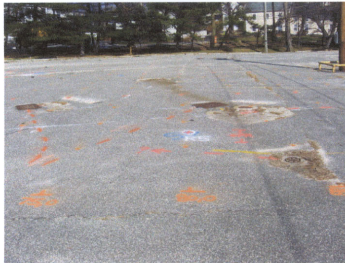
Photograph 4: View looking north toward PEBS R-SB-5. Electric lines are visible extending south from two electric vaults and a suspected utility is visible extending west immediately south of the PEBS.
