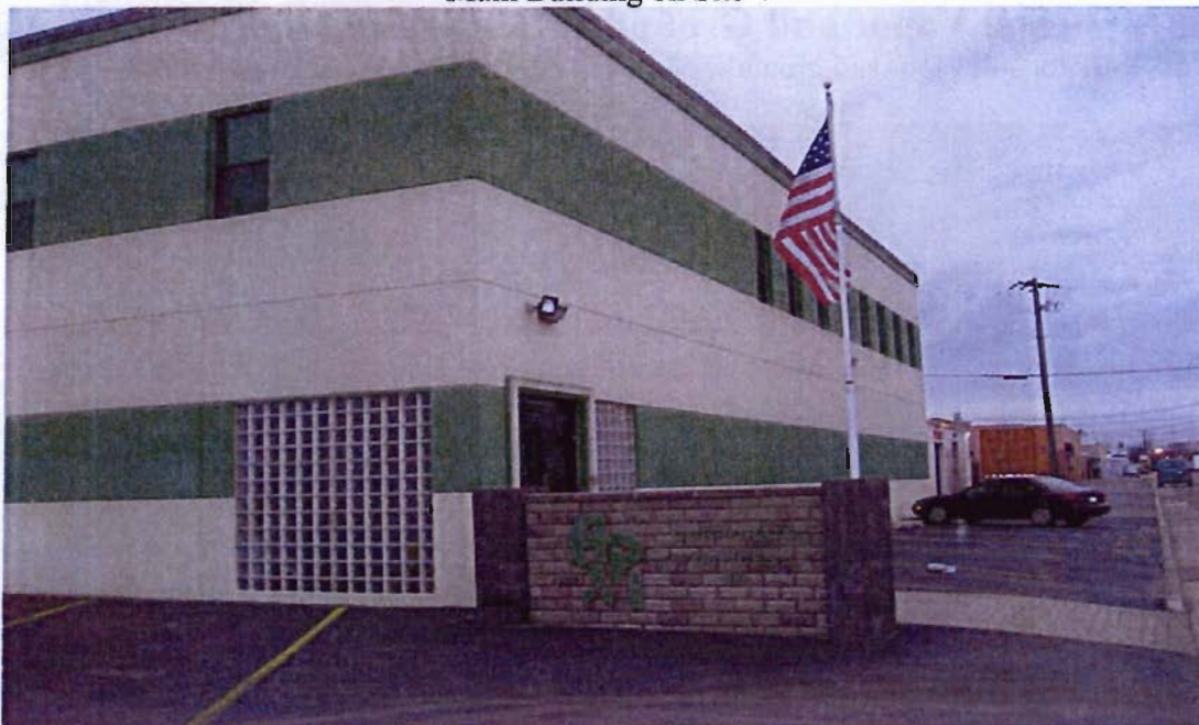
Main Building on Site V
