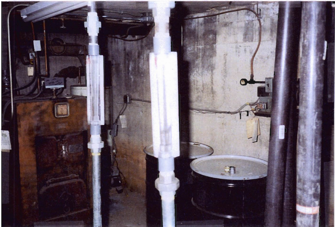
19. AS flow meters for high and low sparge points
