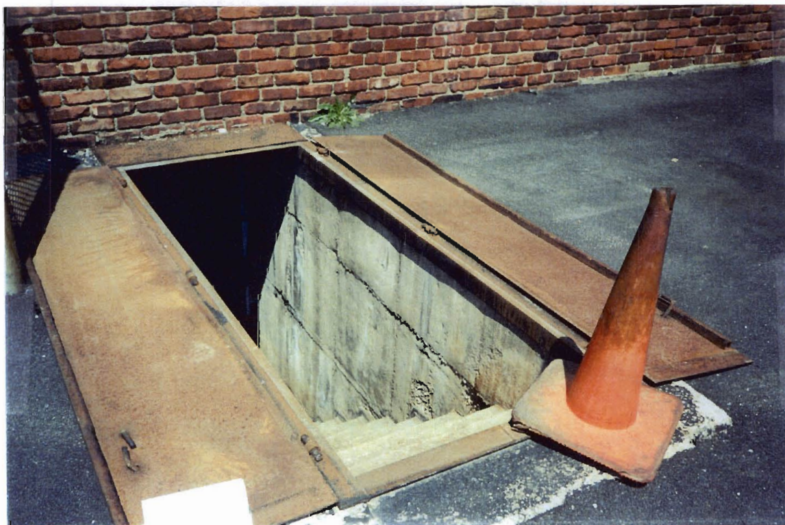
2. Metal doors providing access to Atlas Graphics basement
