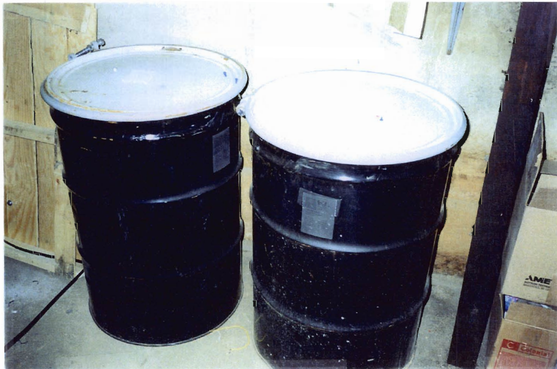
14. Storage drums in site basement for liquid collected from SVES moisture separator
