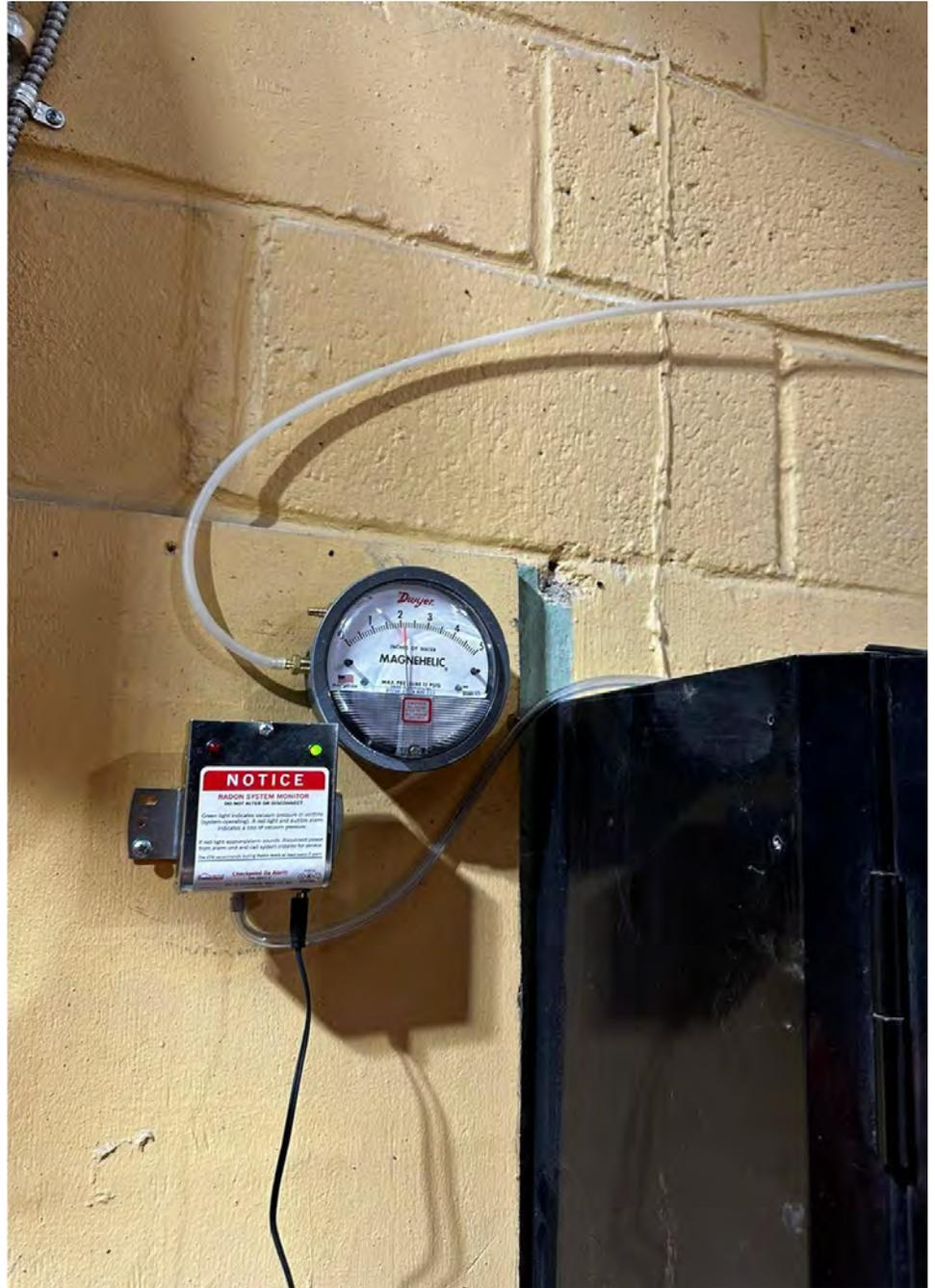
pressure alarm and sample tap were added after 3/22/23 inspection, The Magnehelic gauge was replaced out for a more appropriate range.
