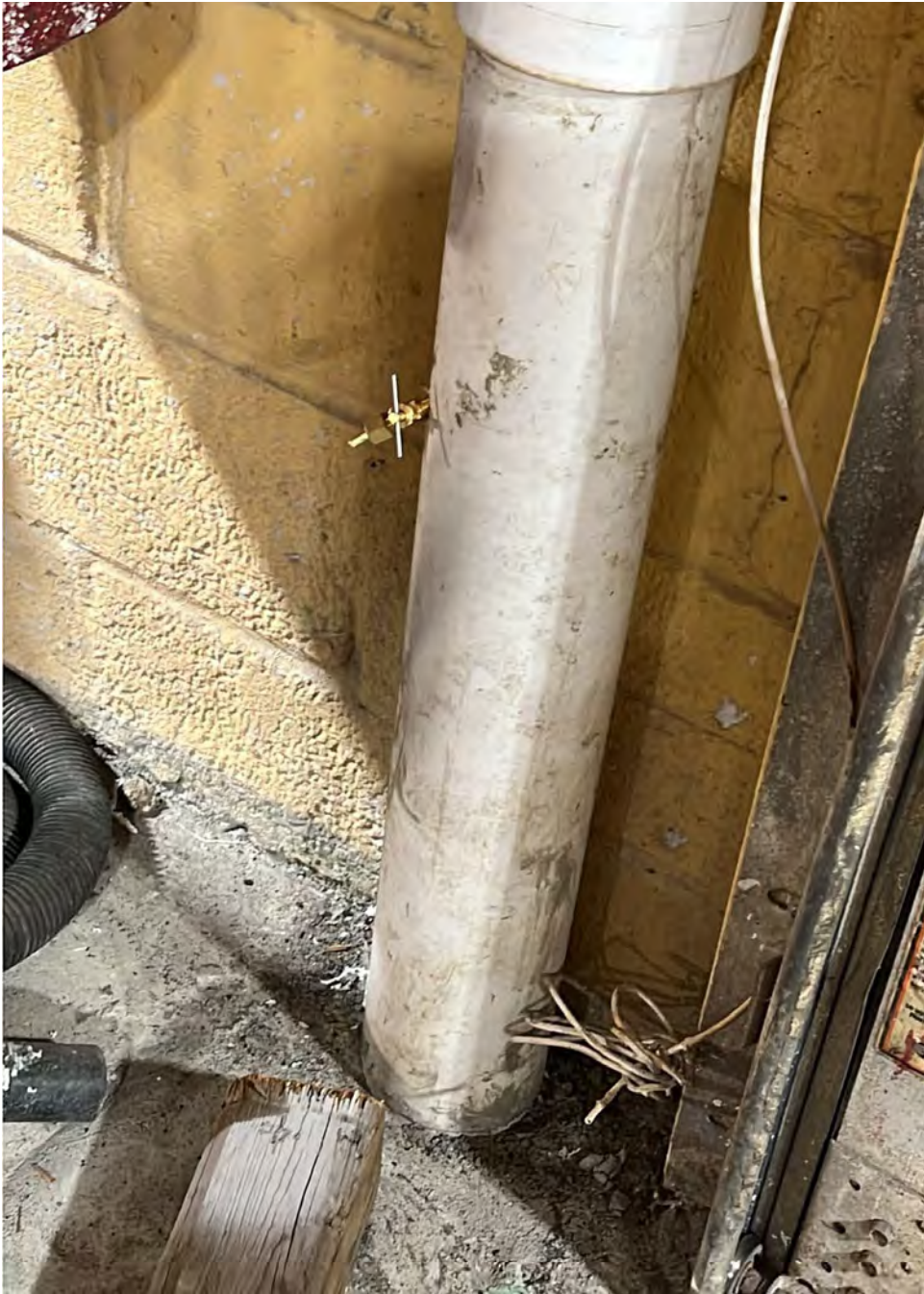
pressure alarm and sample tap were added after 3/22/23 inspection, The Magnahelic gauge was replaced out for a more appropriate range.
